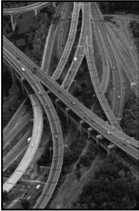
FIGURE 4.5 Roadway interchange in Waterbury, Connecticut.
