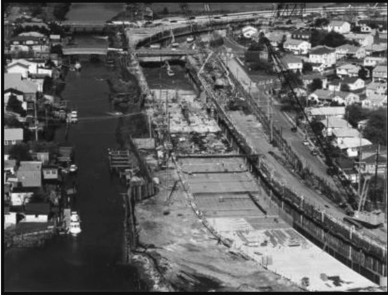
FIGURE 4.14 Construction of the Atlantic City/Brigantine Connector.
