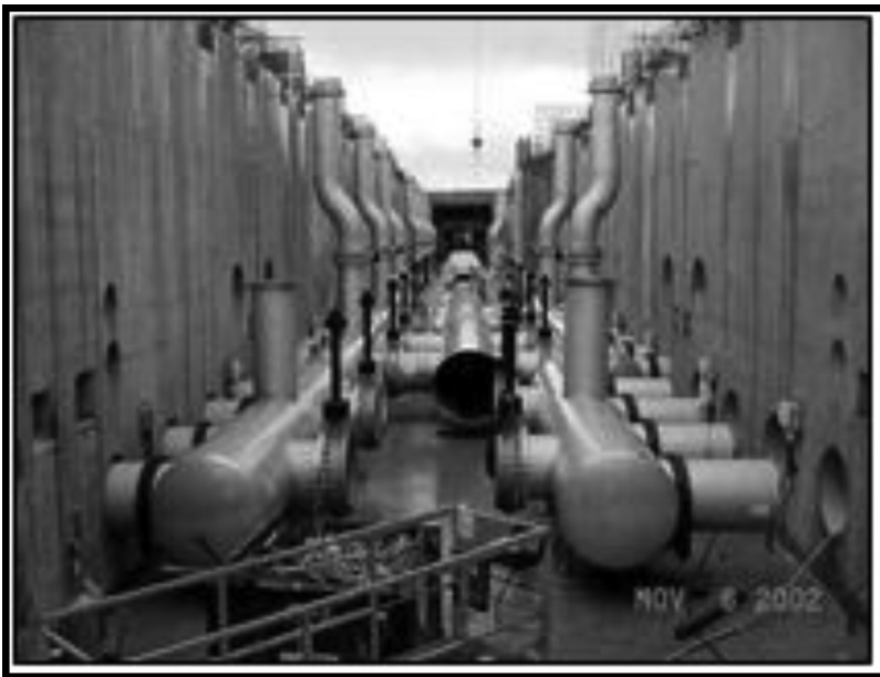
FIGURE 5.2 Construction of the BAF gallery.
