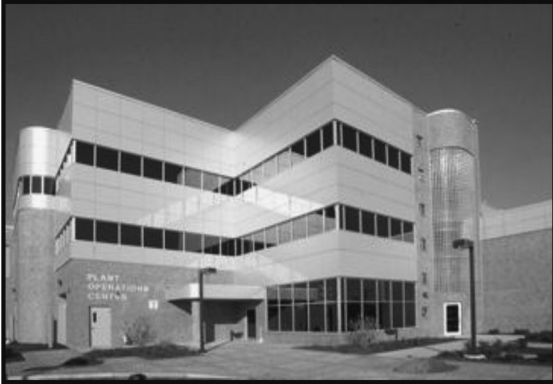
FIGURE 5.5 Plant operations center at Metro.
