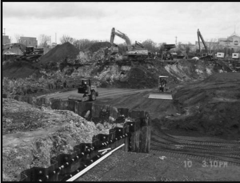
FIGURE 5.8 Excavation for Metro.
