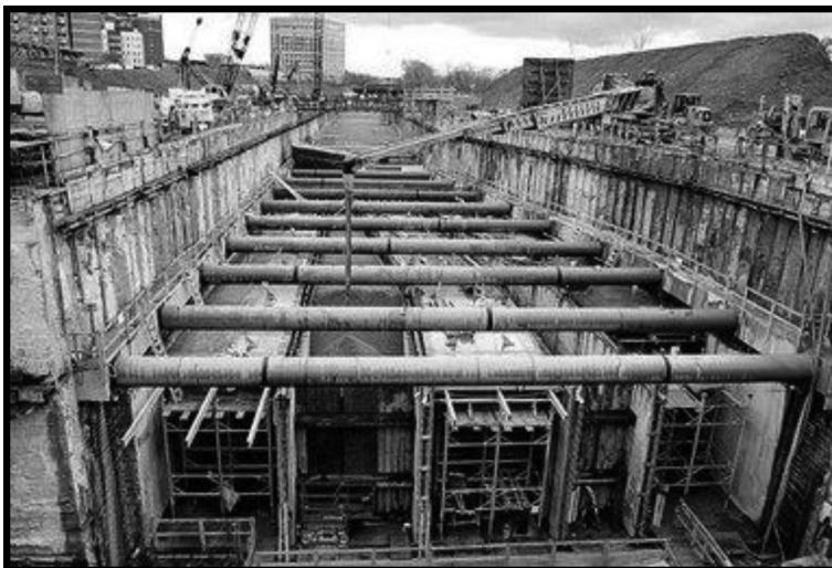
FIGURE 4.13 Cut and cover approach (Clinton Storage Facility).
