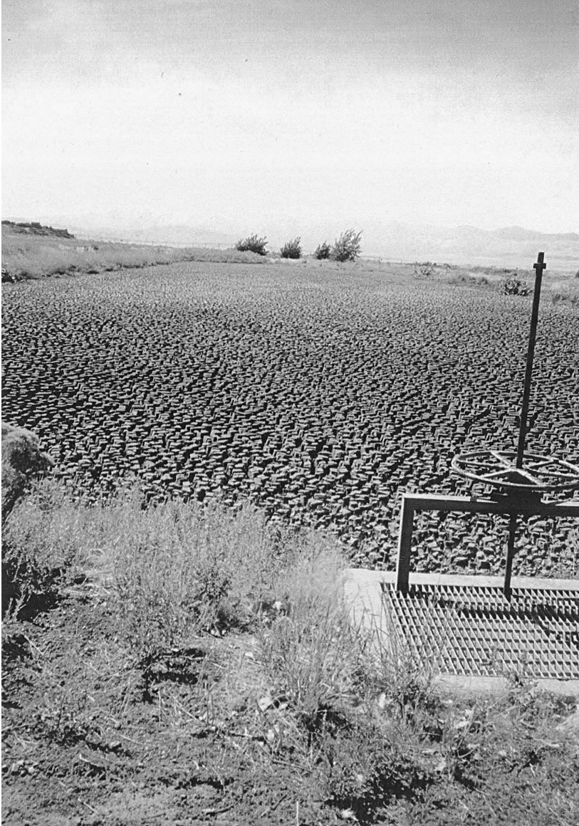
Figure 5.5.38b View of Sludge Dewatering Lagoon with Dried Sludge
