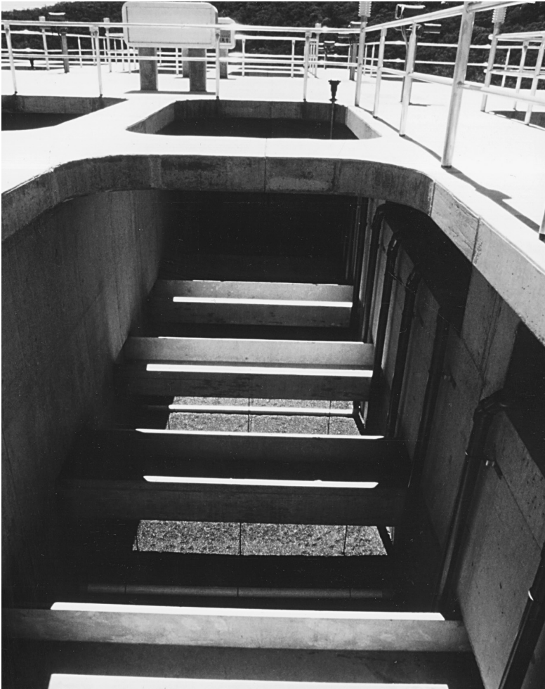
Figure 5.5.26a Filter Cell, Granular Media Gravity Filter
