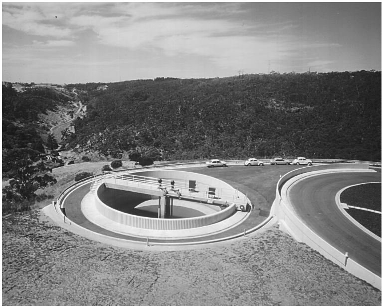
Figure 5.5.33a Filter Waste Wash Water Storage Tank
