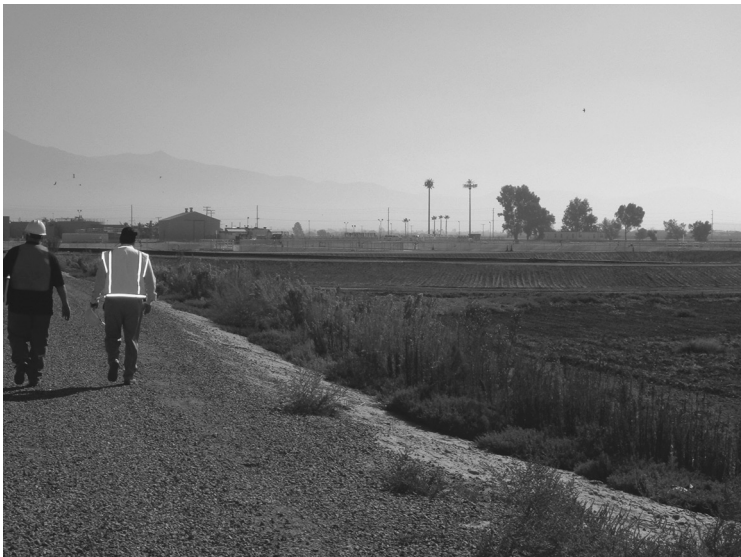
Figure 5.5.38a View of Sludge Dewatering Lagoons
