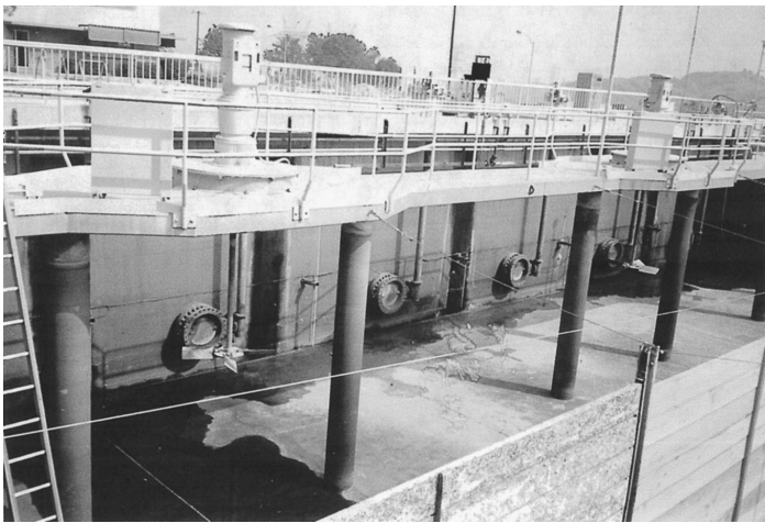
Figure 5.5.21a Vertical Shaft Flocculator with Mixing Blades
