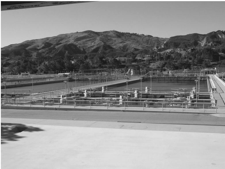
Figure 5.5.17a Flocculation and Rectangular Clarifier Basins
