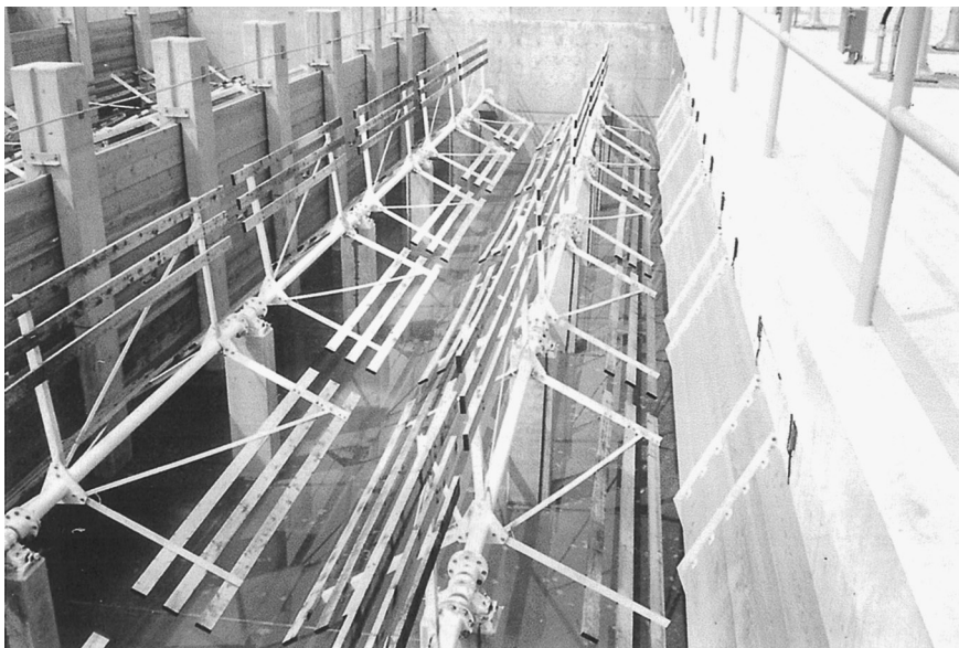
Figure 5.5.21b Horizontal Shaft Flocculator with Paddle-Type Blades
