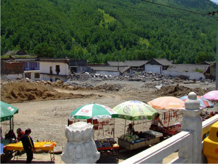
Fig. 6.2 Dozens of local homes were demolished in Taihuai, Mount Wutai, after the area became a national park and a world heritage site in 2010
