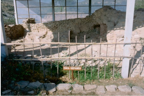
Fig. 3.2 Photograph of House 11–12 (or ‘potter’s house’) at the tell of Sesklo, as preserved today, showing the internal organisation during the final phase of the house, when the internal partition wall was introduced, the entrance to room 11 on the left was blocked and the porch or sheltered yard behind it was abandoned. Buttress, recesses and walls of room 12 on the right coated with multiple layers of red plaster; lower part of the wall also lined with upright stone slabs. Large retaining wall of the tell visible in the background. (Photograph by the author)
