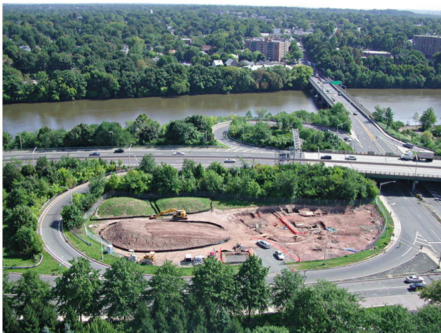
Fig. 9.1 Overhead view of route 18/27 interchange site, New Brunswick, New Jersey
