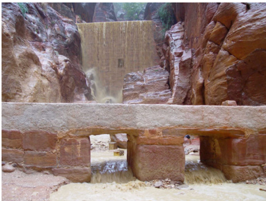
Fig. 2.42 Overflow in Qantara Dam, 2004 (Courtesy S. Farajat)
