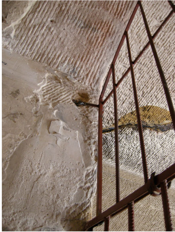
Fig. 2.33 Damage to stonework due to fixing of grille to wall in Biclinium 849, 2010 (Courtesy PNT and Courtauld)
