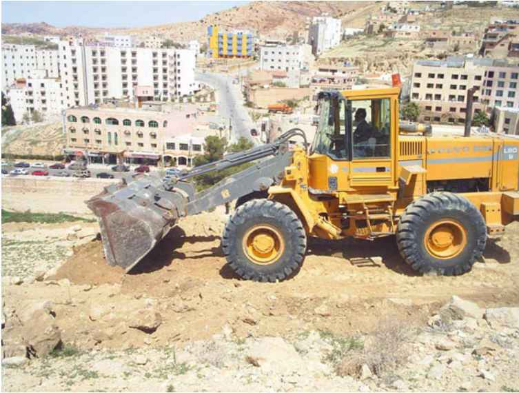
Fig. 2.14 Bulldozer levelling area for terracing, 2007 (Courtesy PNT)
