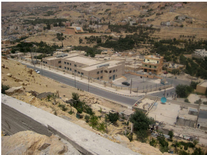
Fig. 2.13 Traditional architecture in Khirbet Bani Atta after demolition, 2011 (Courtesy PNT)
