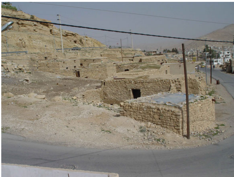
Fig. 2.12 Traditional architecture in Khirbet Bani Atta before demolition, 2004 (Courtesy S. Farajat)
