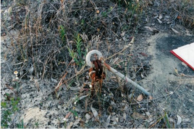
**Fig. 8.14** Cyclone chain anchor set into concrete block
