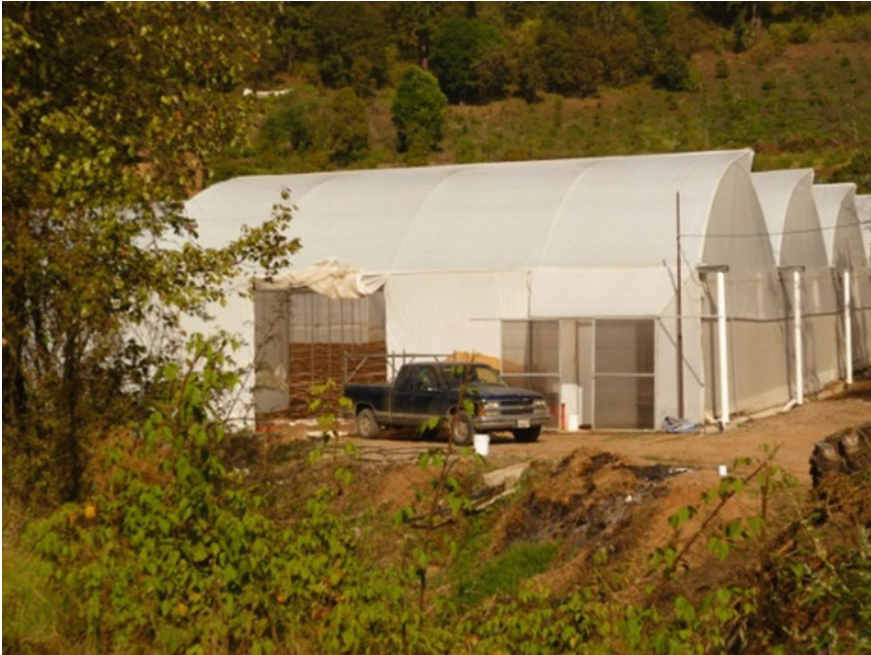
Fig. 4.2 Installation process of a greenhouse for tomatoes in Las Vueltas, Coatepec Harinas, State of Mexico. Source Photograph taken by the author during the research carried out in the community
