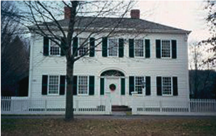
Fig. 3.7 Home of Ebenezer Hinsdale and Anna Williams and later tenants. Photograph by Broughton Anderson. Used by permission
