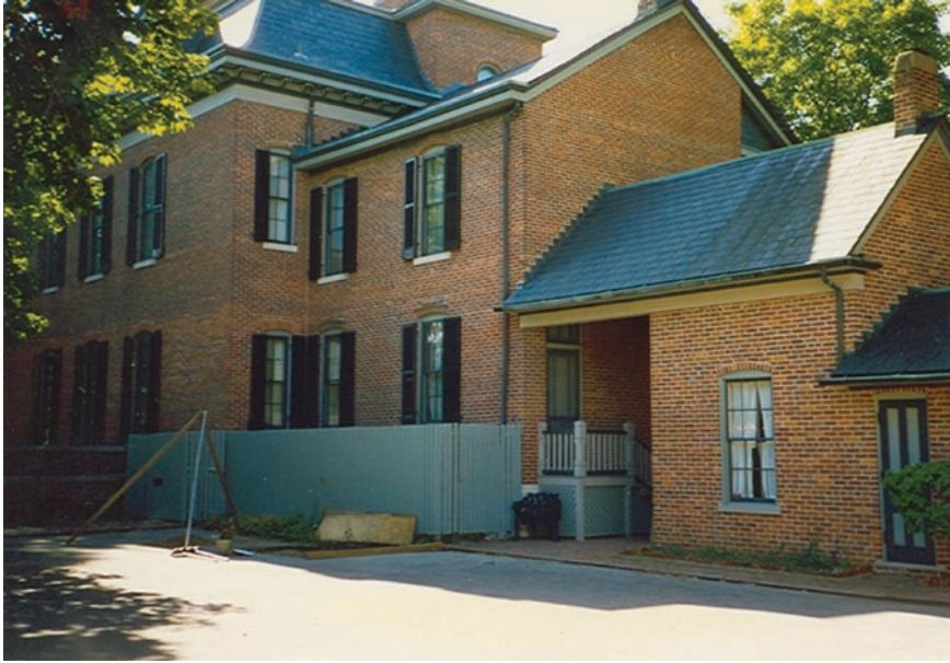
Fig. 4.3 The rear section of the Morris-House showing (from left to right) the main house, the kitchen ell, the roofed passageway, the summer kitchen, and attached privy. Facing southeast. Photograph by the author
