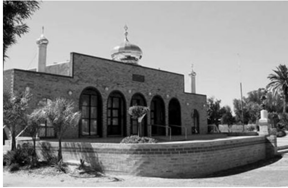
Fig. 11.1 Katanning Mosque, Andrews Road Katanning, November 2005 (Kirrily Jordan)
