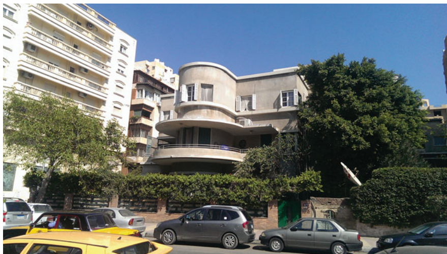
Fig. 11.4 Villa listed on the local level ( source : Authors)
