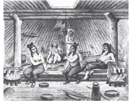
FIGURE 82 “Interior of the igloo of Noulloumallok.” Stylized view of one sleeping area within the house, indicating leaned timbers for the back wall. Heavy Y-shaped posts uphold part of the frame (inaccurately drawn) supporting the central roof (with skylight). Note the slightly raised sleeping platform, soapstone lamps (also misdrawn) on lateral wooden stands (with drying racks—evidently floating—above them) that sit on the central floor, and a general clutter of utensils, vessels, and weapons about the house. From Petitot 1887; 1981:40.
