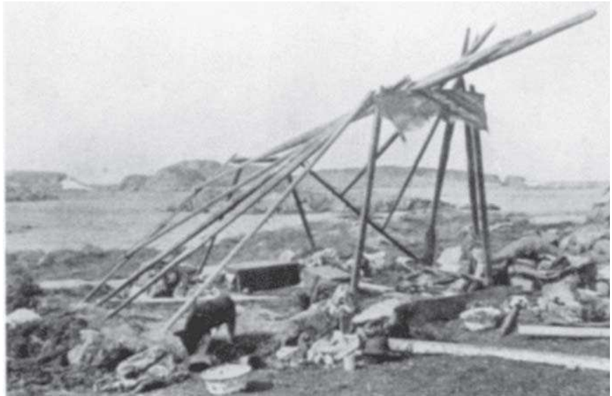
FIGURE 28 Framework for erqulik [double-arch] tent. The lower rear arch (left) has two central uprights as well as two forward-leaning lat- erals, which spread the back considerably and provide support for the side-wall poles. From Birket-Smith 1924:fig. 119.
