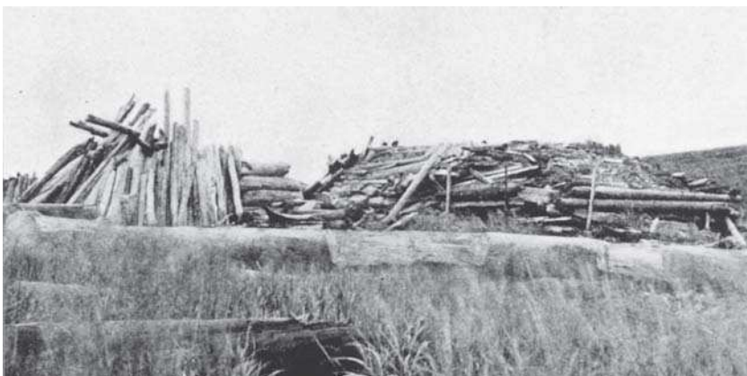
FIGURE 83 “Mackenzie River house in summer. The doorway to the forty-foot alleyway is at the left of the picture.” Note the rude stacking of timbers, some vertical, others horizontal. From Stefánsson 1913:60 ff.
