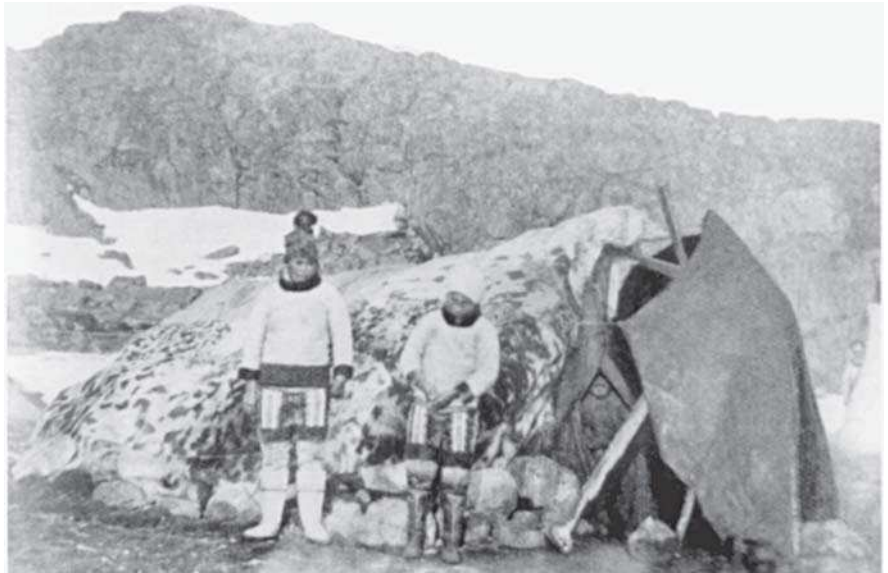
FIGURE 27 “Sealskin tent of erqulik [double-arch] type. Notice windbreak in front.” From Birket-Smith 1924:fig. 117.
