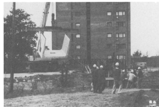
Figure 7.64 Stages of construction
