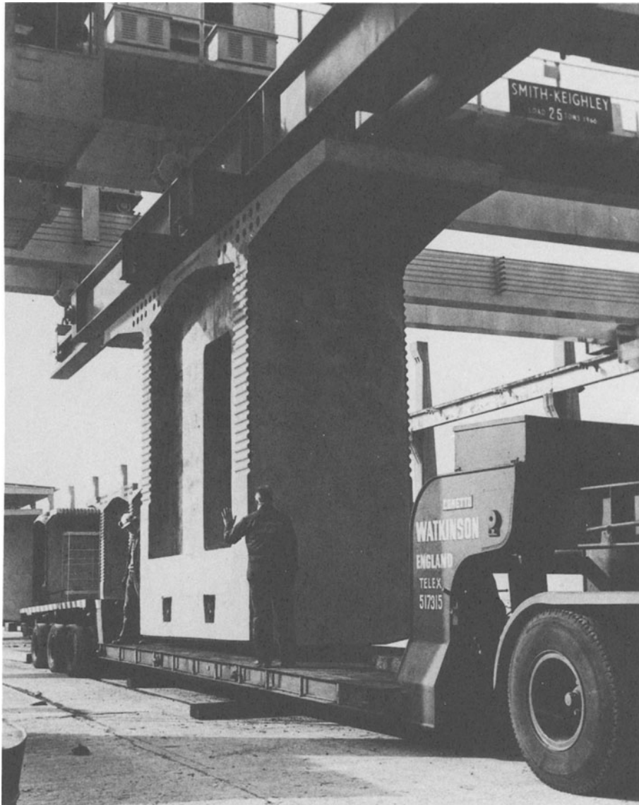
Figure 7.1 Bridge segment: reinforced concrete bridge unit being loaded for transport (courtesy of Dow-Mac Concrete Ltd)
