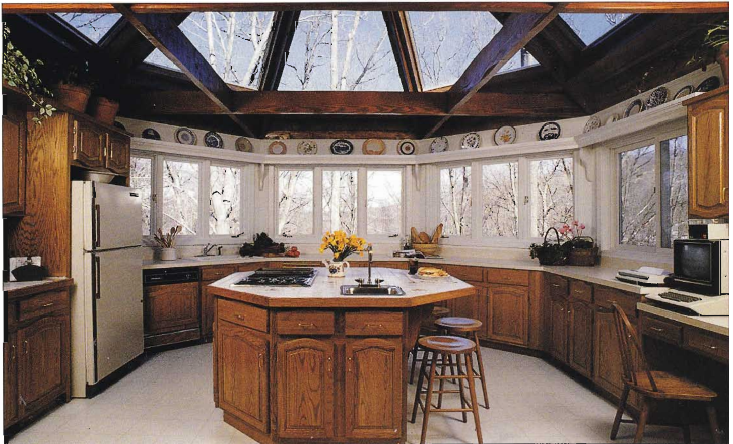
Skylights placed between the rafters of this vaulted ceiling allow for stargazing during midnight snacks. Raising the ceiling increases the perceived square footage of any room.
