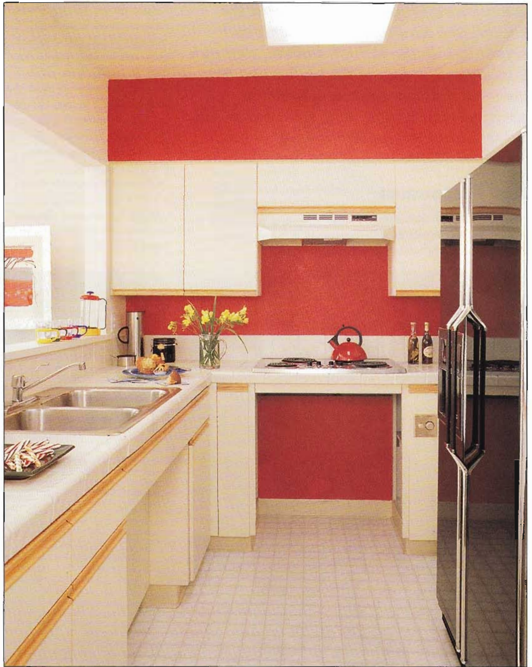
A wheelchair user remodeled this galley-shaped condominium kitchen to serve his special needs. The open space under the cooktop allows him to pull in close while cooking; shelves in the opening hold pots and pans; burner controls are placed within reach on the right side of the cooktop. Eliminating the under-sink cabinet and lowering the counter provide sink access.
