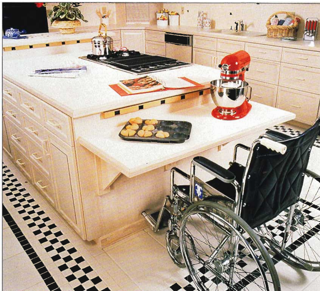
Remember electrical needs on kitchen islands. A strip of receptacles provides juice for a multitude of modern appliances on this cantilevered work surface.
