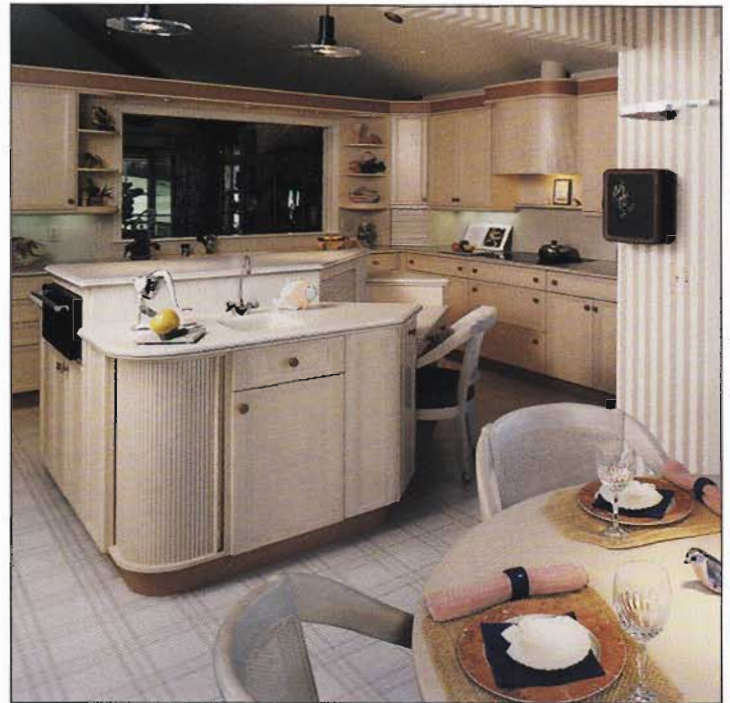
Because tambour doors, seen here on the island, behind the desk, and covering the corner appliance garage, provide interior access without having to allow for door swing, they are a good choice for tight spaces.
