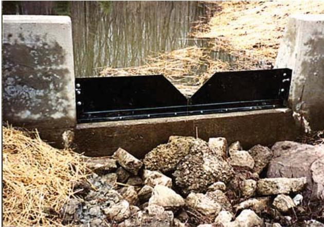
Figure 12.10 V-notch weir. Photograph courtesy of US Geological Survey.
