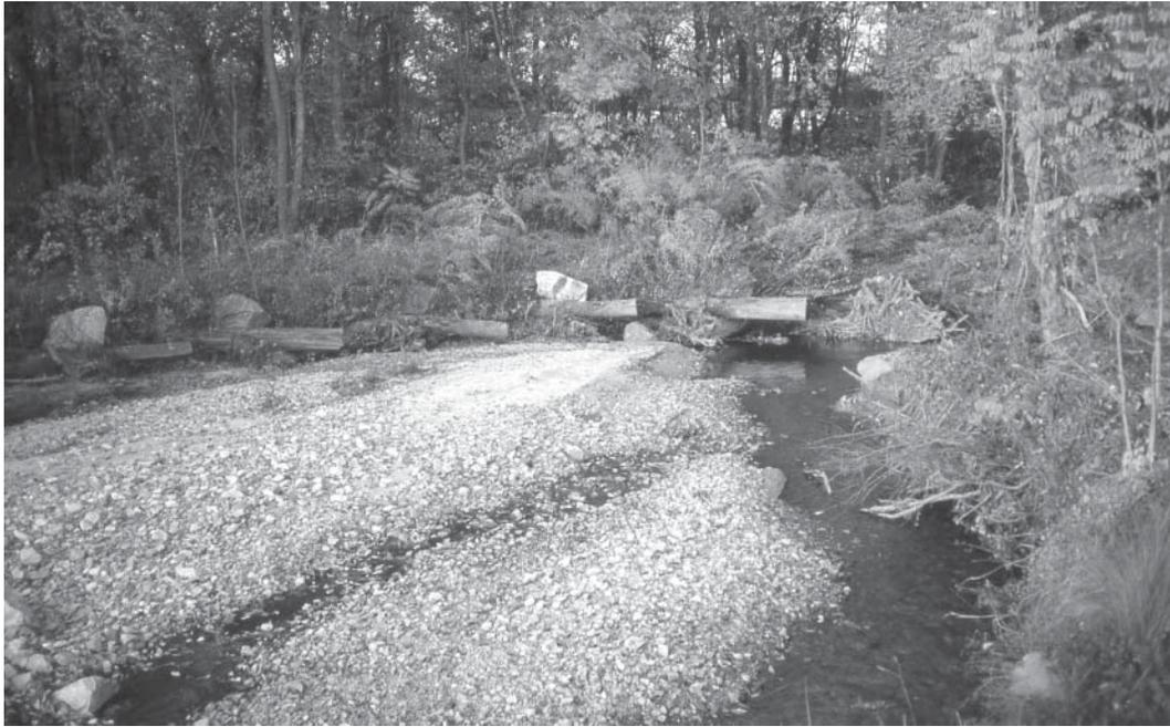
**Figure 7.16** View downstream on Deep Run in 1999, after project construction, showing root-wad and boulder structures in left bank still intact, but abandoned, as the stream eroded a new channel to the right of the idealized meander bend constructed here. Source: Kondolf, 1999.
