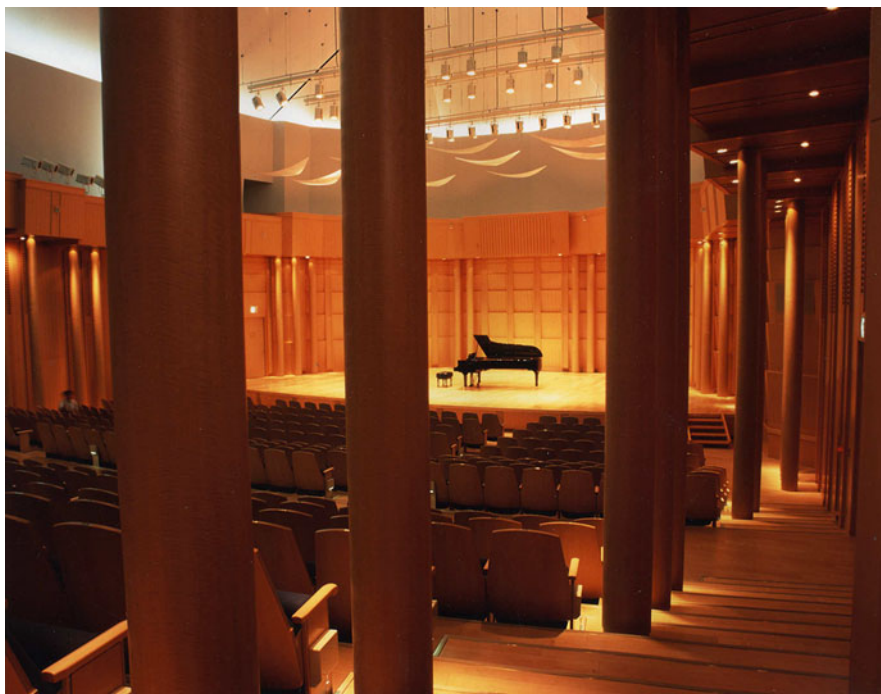
Photo 13.3 Tsuyoma Music Cultural Hall (Belle Foret Tsuyama) with 52 columns (each of the columns was 30 cm in diameter) located in front of the walls
