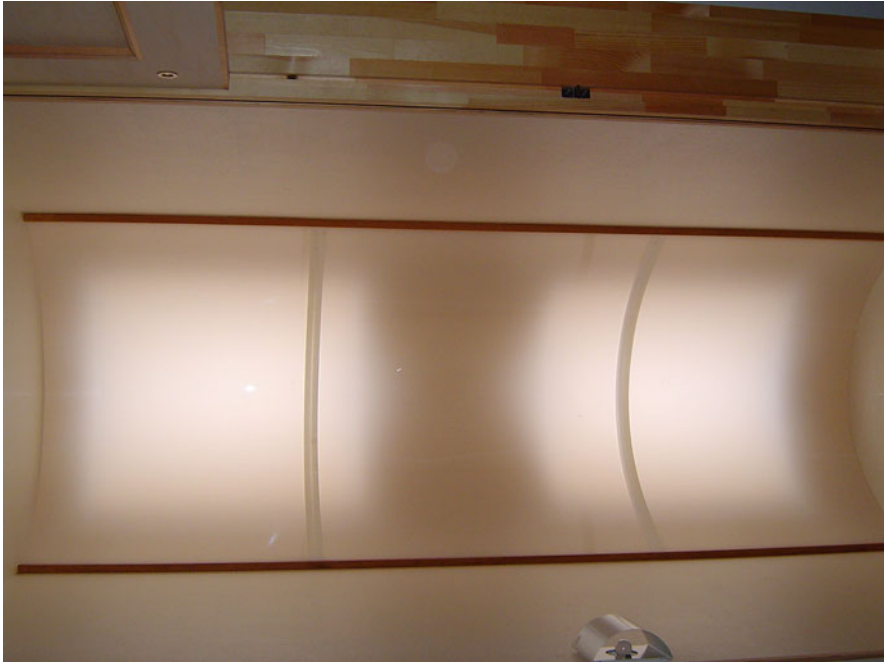
Photo 11.8 Aisle with scattered skylights
