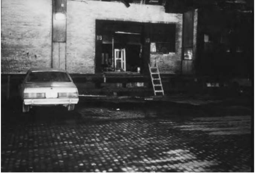
Figure 11.2 The existing loading dock area before the project began.
