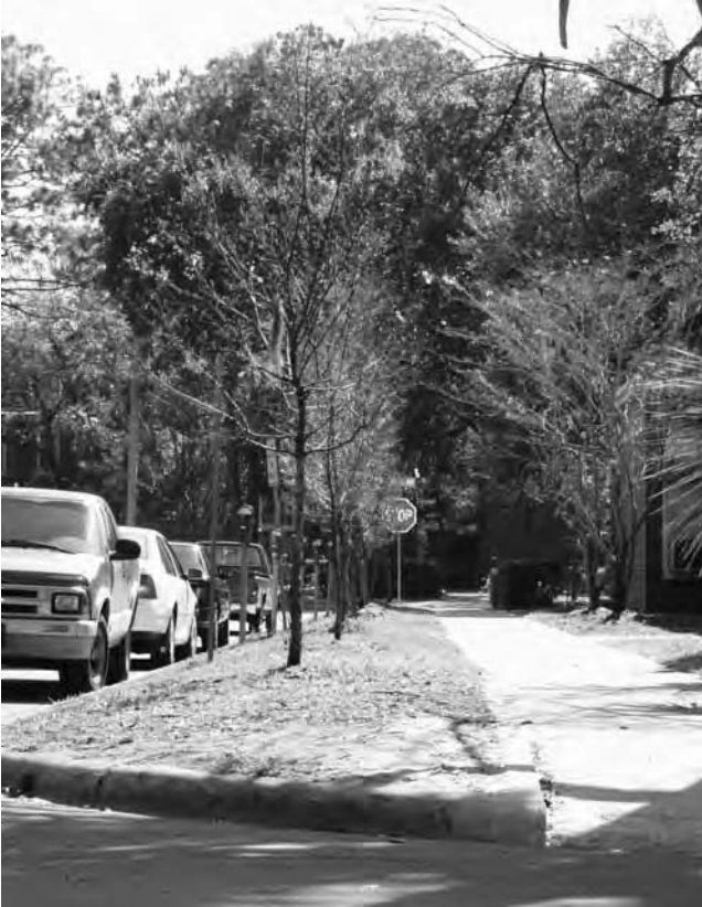
Figure 13.16 A vegetation strip needs to be large enough for a root plate (6 feet) and provide a viable soil material for plant growth. The soil needs to be either protected throughout construction, which is difficult, or replaced with a specified soil material. If the soil is replaced over a compacted subgrade, or if natural drainage is limited, then designed drainage is necessary to prevent periodic flooding. (Photo credit: J. Grabosky.)
