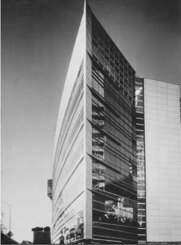
Figure 9.2 New York Psychiatric Institute — corner of building. (Photography by Dan Cornish.)
