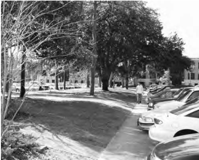
Figure 13.13 Berm planting on the University of Florida Campus parking lot. Note the width and sloped sides to the pedestrian walkway. (Photo credit: J. Grabosky.)
