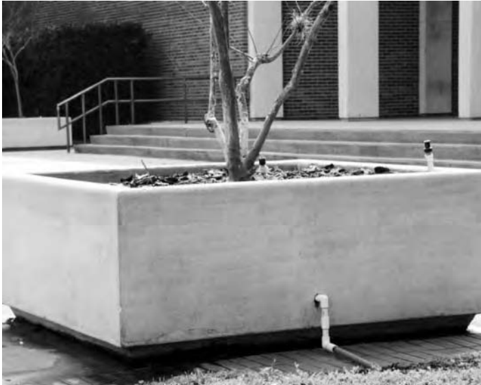
Figure 13.24 Stationary container with 2 irrigation risers. Drainage is gravitational out to the pavement surface treatment. Note the discoloration near the container. (Photo credit: J. Grabosky.)
