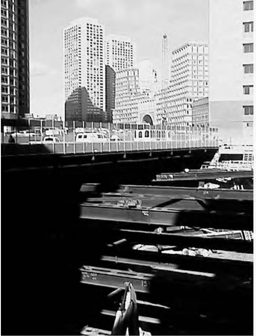
Figure 3.11 A deep internally braced excavation in Boston, MA.
