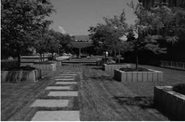
Figure 13.10 Roof-top landscapes re-create a landscape in a thin veneer of soil. Containment and control of irrigation and drainage must be considered to protect the building. (Photo credit: E. Gilman.)
