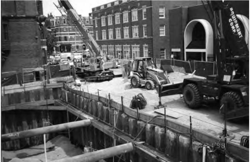
Figure 3.10 Overview of braced excavation, Boston, Massachusetts.
