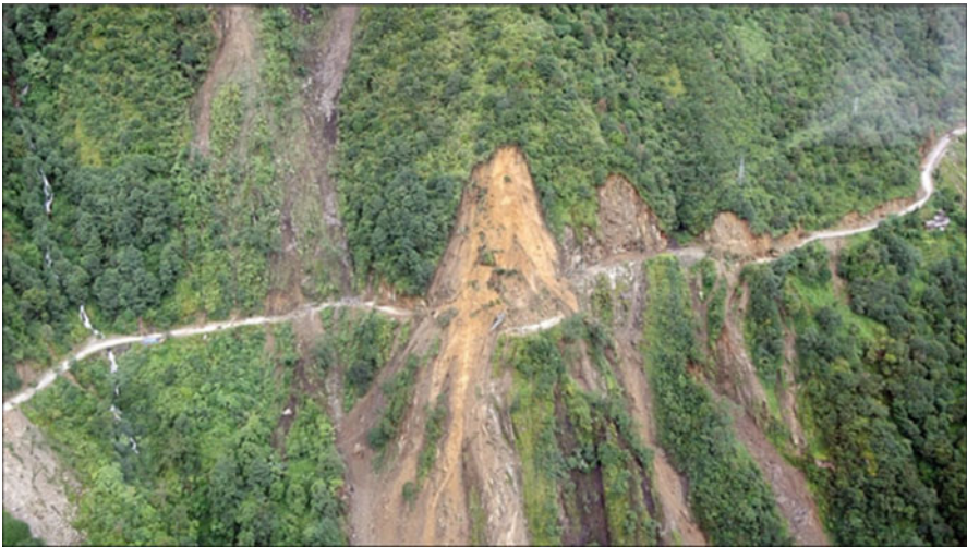
Fig. 6.2 Landslide-affected roadway in Darjeeling District ( Source: Save the Hills)
