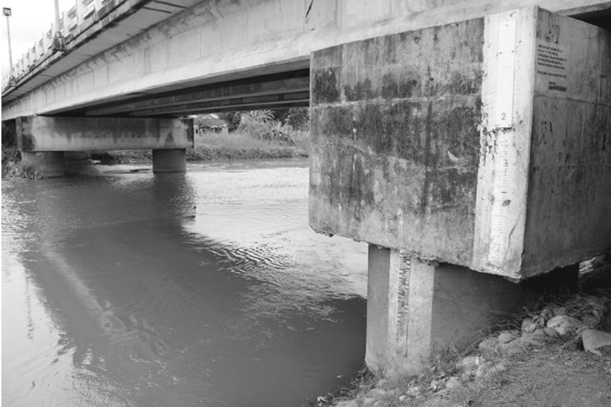
Fig. 8.8 Flood maker under the bridge (Photo by F. Molina 2014)
