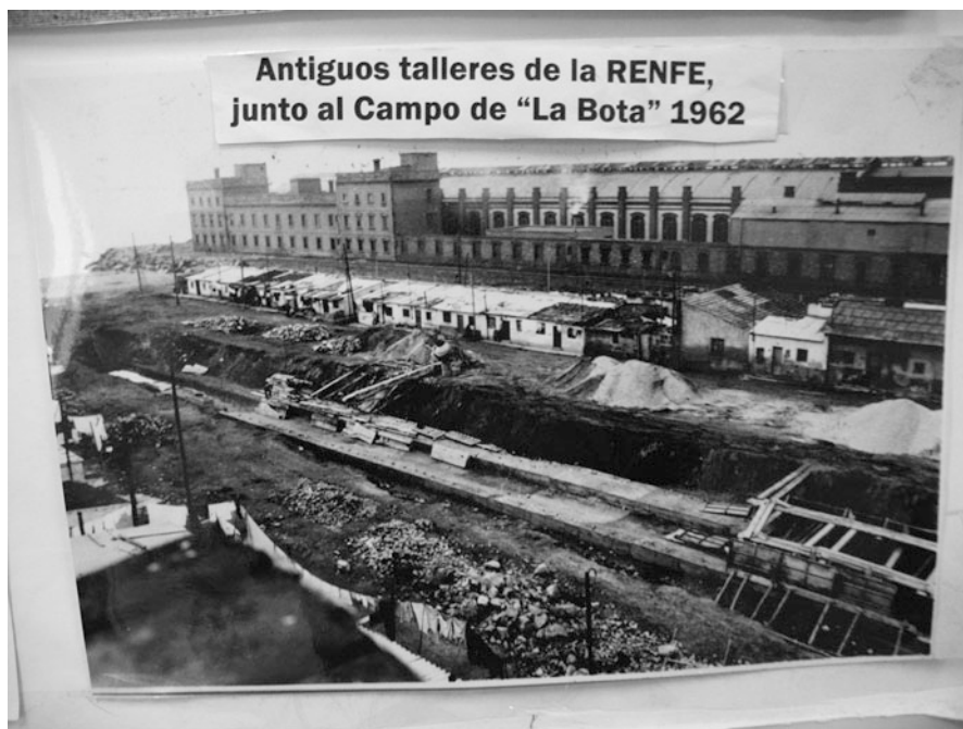
Fig. 1 Old stores of the Spanish railway company in the Forum's space in 1962 (Photo: archive of the neighborhood association)
