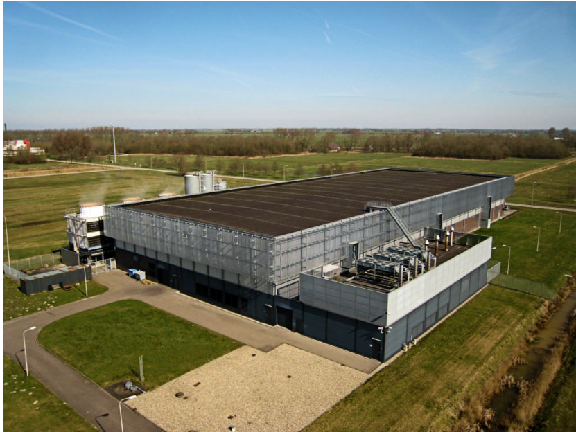
Figure 1: Sig Telehousing datacentre, Groningen Kite Aerial Photograph © 2009 Eric Kieboom, All Rights Reserved
