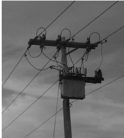
FIGURE 11.10 Three-phase recloser that provides fault sensing and switching.
