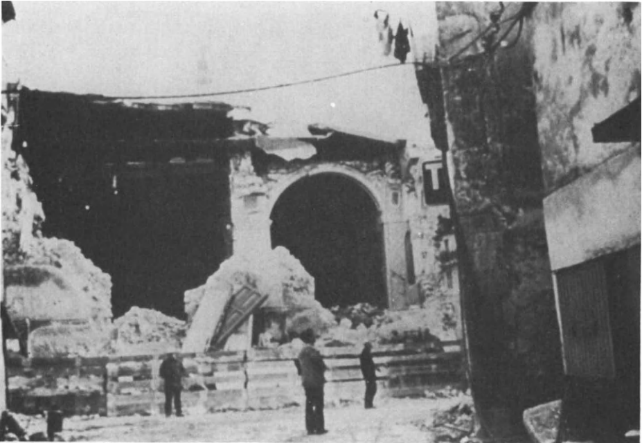
Figure 1.8. Valvano, Italy: Collapse of Church Caused by Earthquake of November 23, 1980. National Academy Press.
