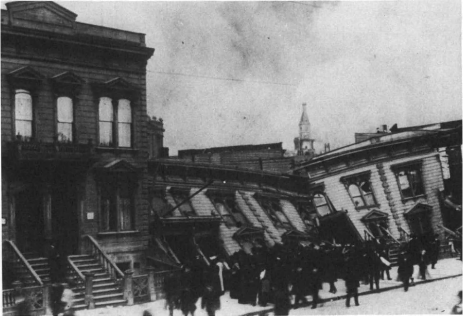
Figure 1.14. San Francisco, California: Buildings Affected by Ground Subsidence in Earthquake of April 18, 1906. NOAA/EDIS.
