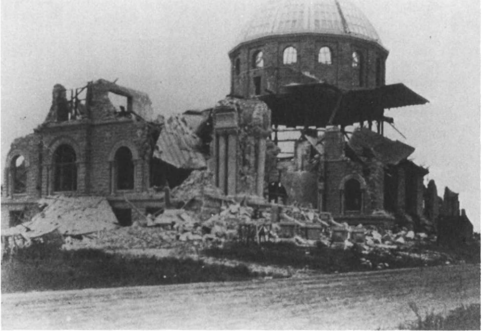
Figure 3.3. Palo Alto, California: Stanford University Library, Shepley, Rutan and Coolidge, Archs., 1887-1891, Damage from Earthquake of April 18, 1906. USGS.
