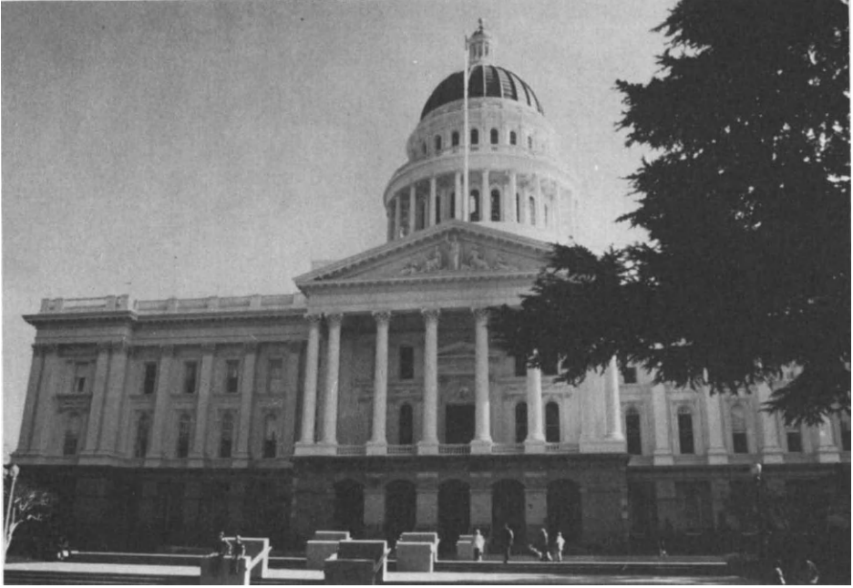
Figure 3.36. Sacramento, California: California State Capitol, Miner Frederick Butler, Arch., 1864-1974, Rebuilt, Restored and Seismically Strengthened, 1980.
