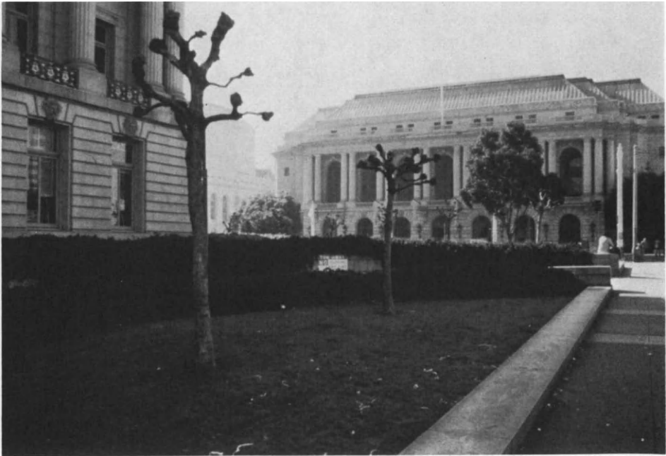
Figure 3.29. San Francisco, California: San Francisco Museum of Modern Art, Brown and Landsburgh, Archs., 1932, Steel Frame and Concrete Construction.
