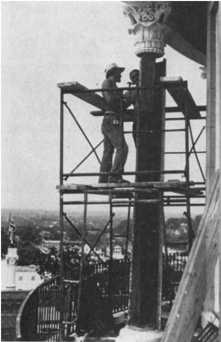
Figure 5.39. Montgomery, Alabama: Alabama State Capitol, 1850, Sectional Steel Columns Threaded Through Base and Capital Being Wrapped by Wood Shafts.
