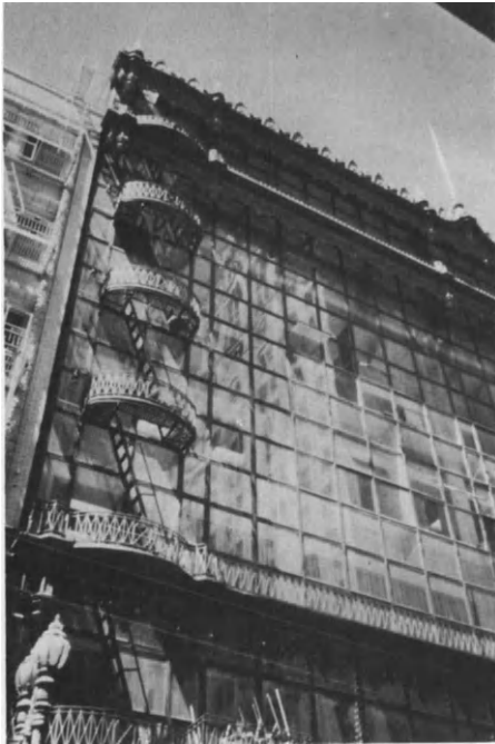
Figure 3.38. San Francisco, California: Palace of Fine Arts, Bernard Maybeck, Arch., 1915, Pan Pacific Exposition Theme Building, Originally Lath and Plaster, Rebuilt with Reinforced Concrete, 1960's.
