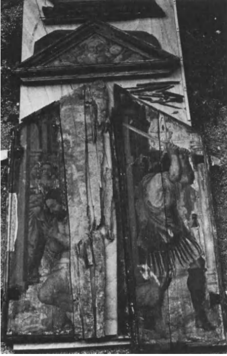
Figure 5.52. Maiano, Italy: Chiesa di San Giovanni Battista, Tabernacle, 17th Century, Broken Pieces after Earthquake of May 6, 1976.
