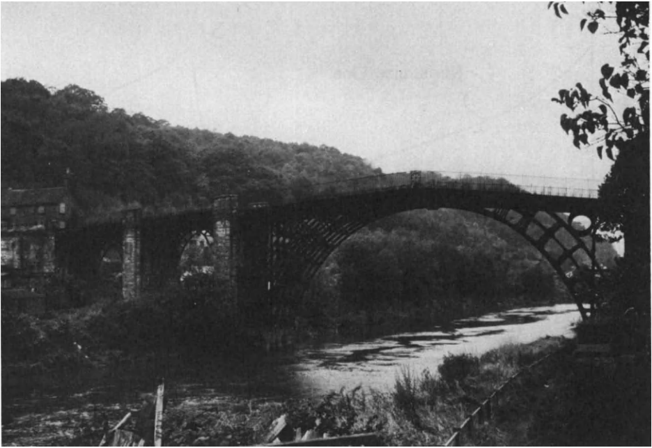
Figure 3.25. Coalbrookdale, England: Iron Bridge Across the Severn River Built in 1779. This First Important Structural Use of Cast Iron was Saved from Effects of Gradual Ground Movement by Inserting a Massive Concrete Bed Underground Between the Stone Piers.
