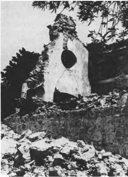
Figure 6.8. Montenegro, Yugoslavia: Church, Showing Destruction Caused by Earthquake of April 15, 1979.
