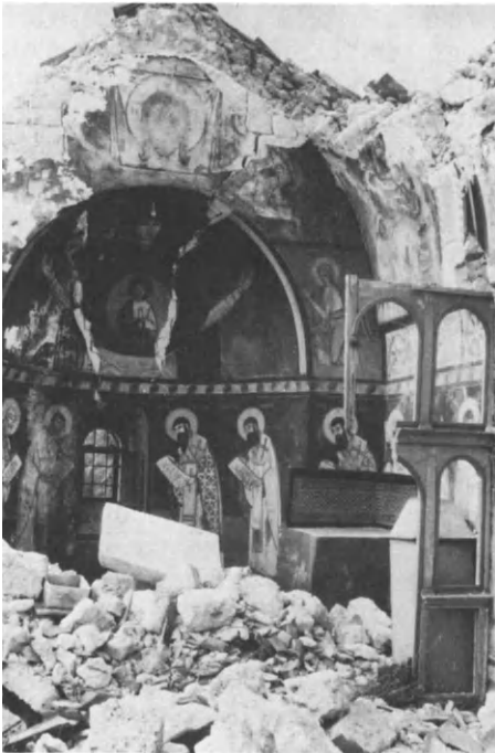
Figure 1.10. Montenegro, Yugoslavia: Frescoed Church After Earthquake of April 15, 1979.
