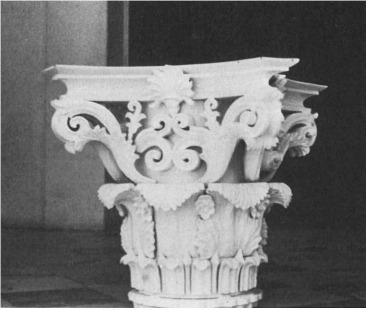
Figure 5.38. Montgomery, Alabama: Alabama State Capitol, 1850, Cast Aluminum Replacement Capitals Made in 1977.
