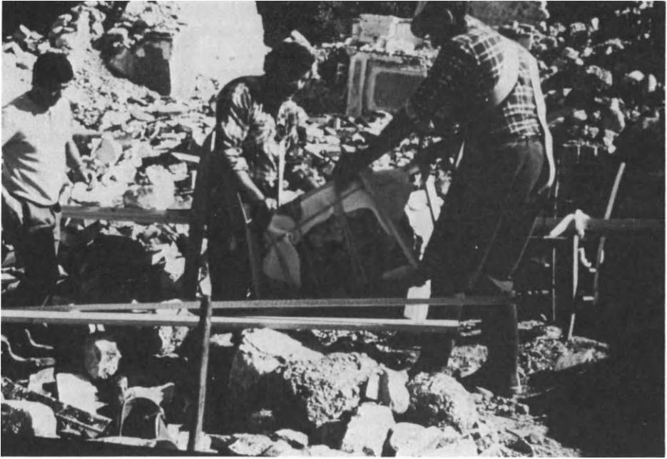
Figure 1.21. Villuzza of Ragogna, Italy: Eleventh Century Fresco Fragments Being Removed with their Supporting Masonry, "Stacco a Massello," Church of San Lorenzo. These Frescoes Came to Light as a Result of Earthquake of May 6, 1976.
