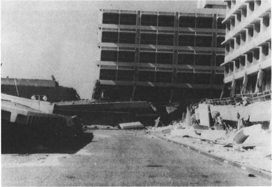
Figure 3.20. Sylmar, California: Olive View Hospital after Earthquake of February 9, 1971.
