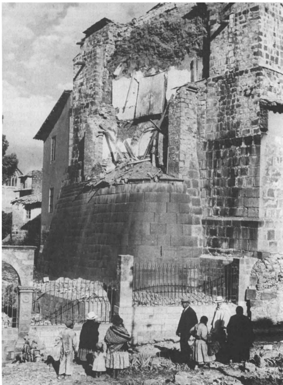
Figure 6.1. Cuzco, Peru: Church after Earthquake of May 21, 1950.
