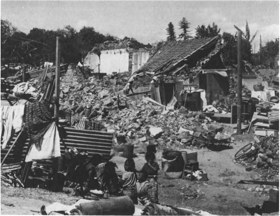
Figure 6.4. Chimaltenango, Guatemala: Destruction of Vernacular Buildings in Earthquake of February 4, 1976.
