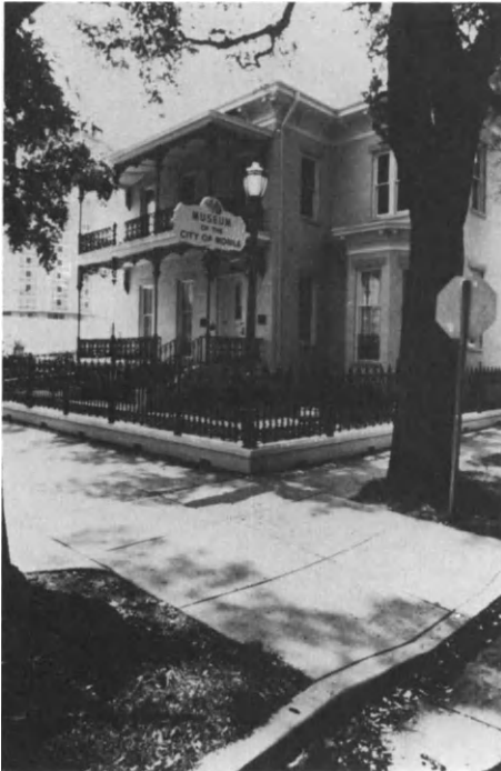
Figure 5.27. Mobile, Alabama: Bernstein House, 1872, Without Window Shutters Before Hurricane Frederick, September 12, 1979.
