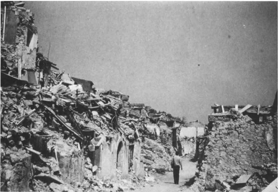
Figure 1.17. Campania-Basilicata, Italy: Village Street after Earthquake of November 23, 1980.
