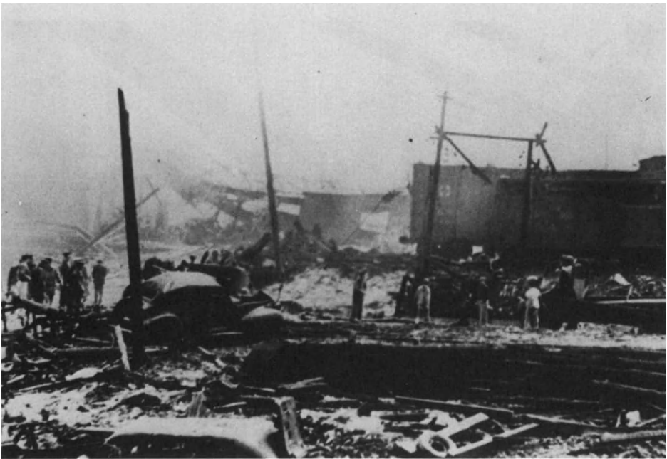
Figure 3.19. Texas City, Texas: Rail Yard Explosion.
