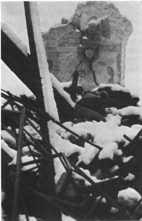
Figure 1.31. Venzone, Italy: Cathedral, the Gonfalone Chapel after its Collapse and the Complete Destruction of the Vault Paintings in the Earthquake of September 15, 1976.
