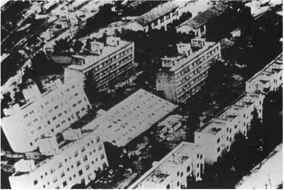
Figure 3.9. Niigata, Japan: Apartment Houses Tilted by Failure of Soil from Liquefaction in Earthquake of June 16, 1964. NOAA/EDIS.
