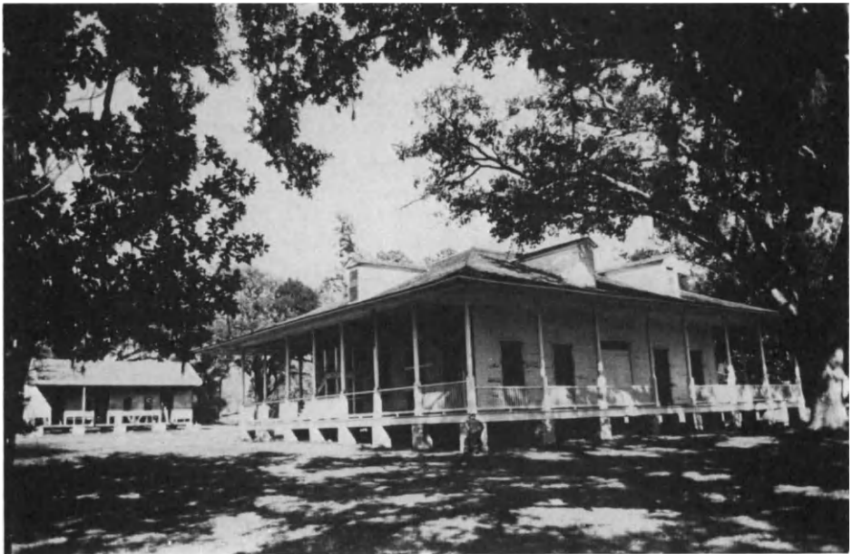
Figure 5.33. Biloxi, Mississippi: Gillis House, 1839, Eaves Lost in Hurricane Camille, August 18, 1969, Restored and Strengthened Which Survived Hurricane Frederick, September 12, 1979.
