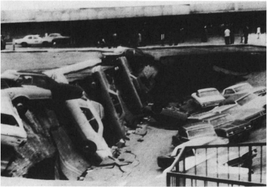
Figure 3.18. Ground Surface Failure from Collapse of Subterranean Chamber.
