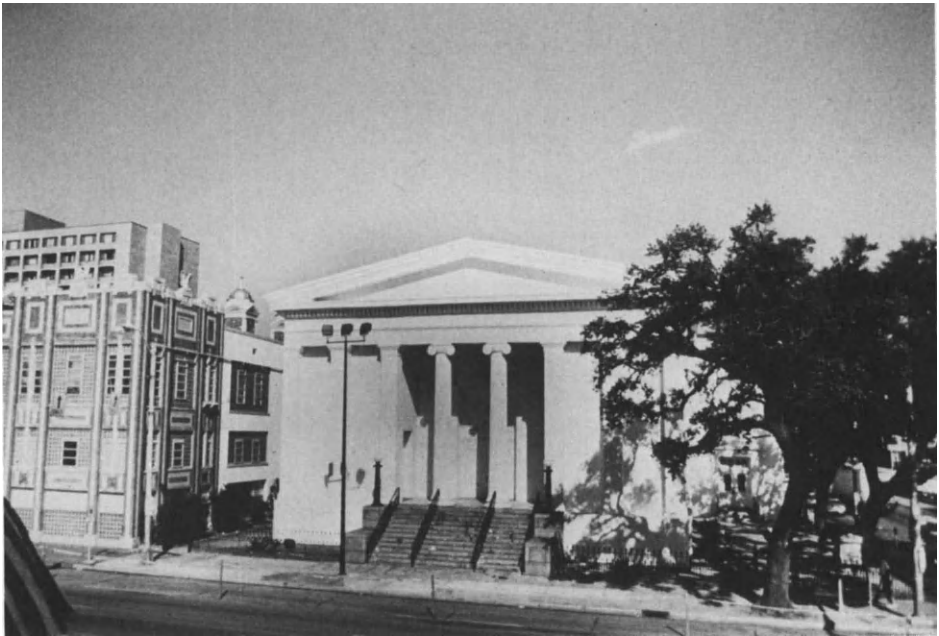
Figure 5.43. Mobile, Alabama: Government Street Presbyterian Church, James Gallier, Sr. and Charles B. Dakin, Archts., 1835, Which Survived Hurricane Frederick, September 12, 1979.
