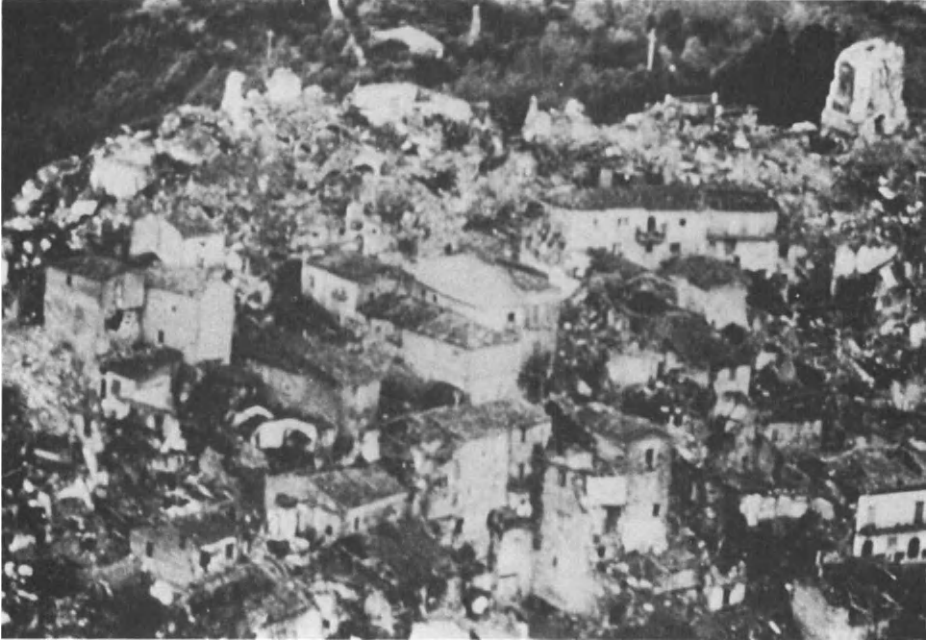
Figure 1.7. Campania, Italy: Destruction of Hill Town by Earthquake of November 23, 1980. National Academy Press.
