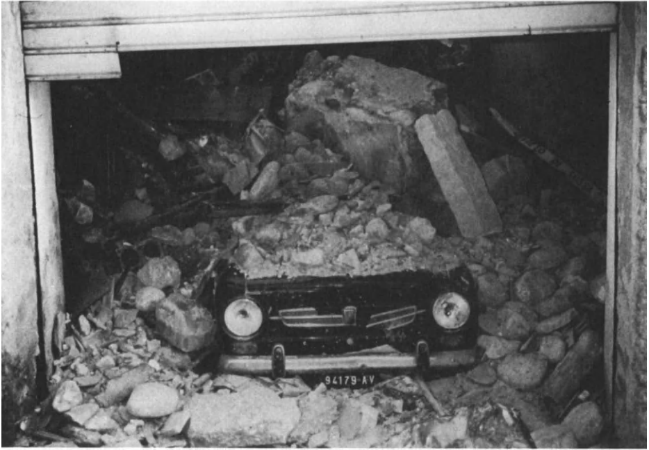
Figure 1.16. Campania-Basilicata, Italy: Collapsed Modern Building after Earthquake of November 23, 1980.
