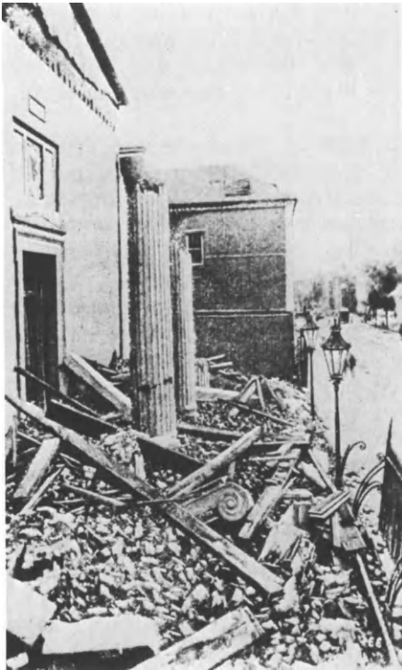
Figure 3.2. Charleston, South Carolina: Damage to Hibernian Hall, 1840, 105 Meeting Street, from Earthquake of August 31, 1886. USGS.
