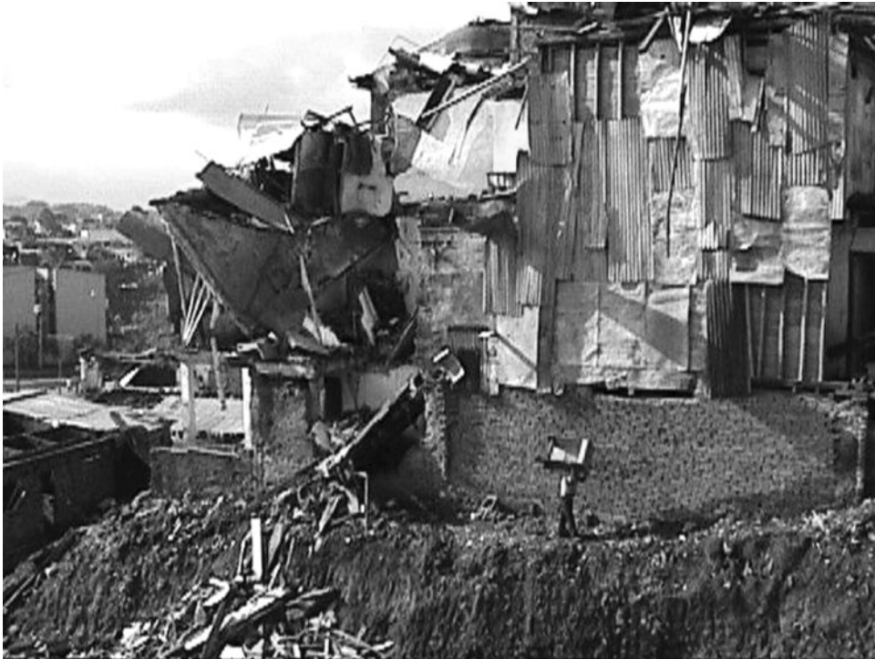
Earthquake damage in Armenia, Colombia, 1999 (World Vision International).
