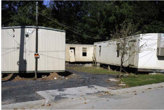
FIGURE 7-3 Austell, Georgia, October 19, 2009. This Cobb County elementary school's 18 temporary classrooms were immersed in 12 feet of water from Sweetwater Creek and are extensively damaged. FEMA Public Assistance funds may pay up to 75 percent of the costs to repair or replace them if an application is made and eligibility is determined.
