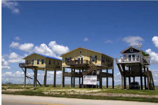
FIGURE 1-1 Gilchrist, Texas, August 16, 2009. These stilt homes were the only structures still standing in the town of Gilchrist after Hurricane Ike destroyed it. FEMA is still working with local, state, and federal agencies to rebuild the town.
