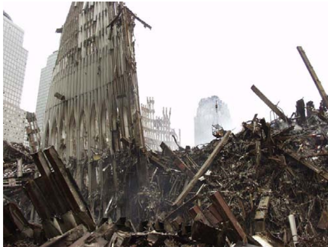
FIGURE 9-2 New York City, New York, September 25, 2001. Fragments of the World Trade Center facade are all that remain of the 110-story structures that once dominated the skyline of lower Manhattan. Photo by Mike Rieger/ FEMA News Photo.
