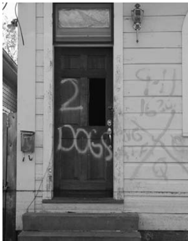
FIGURE 1-3 New Orleans, Louisiana, on September 18, 2005. This shows the damages to homes and property in the lower ninth ward due to Hurricane Katrina. The markings on these houses were made by the search and rescue teams who looked for survivors after the storm. Searchers wrote the date the house was searched, the time, which search party was involved, any survivors found, and any animals that were still in the house. From Andrea Booher/FEMA.
