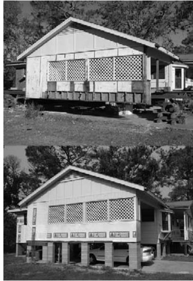
FIGURE 3-1 Pascagoula, Mississippi, November 29, 2005, and August 8, 2006. Before (top) and after (bottom) photos of the elevation of a house flooded by the storm surge of Hurricane Katrina. Elevating a house is an excellent way to protect it against flooding. Mark Wolfe/FEMA.
