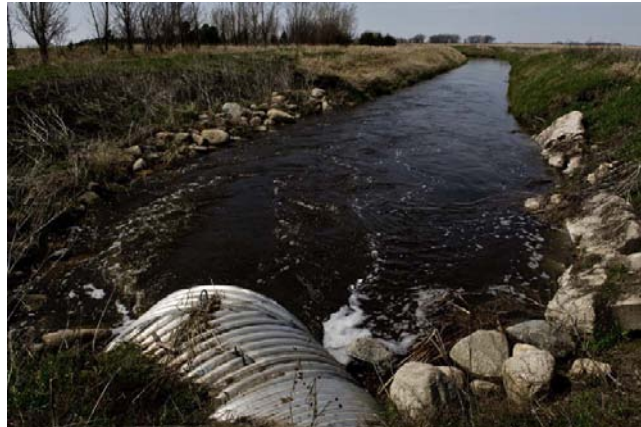
FIGURE 3-5 Sargent County, North Dakota, May 4, 2009. Rocks and an angled culvert help prevent bank erosion on drain 11 in Sargent County. Many areas of North Dakota were covered with floodwater weeks after the storms and floods occurred in March. Eliud Echevarria/FEMA.
