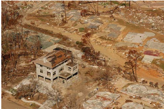
FIGURE 3-2 Pass Christian, Mississippi, October 4, 2005. Aerial photo of the only surviving home in the area that was completely destroyed by Hurricane Katrina. Foundations are all that remain of most of the neighboring homes. The surviving home was built using many FEMA standards. John Fleck/FEMA.
