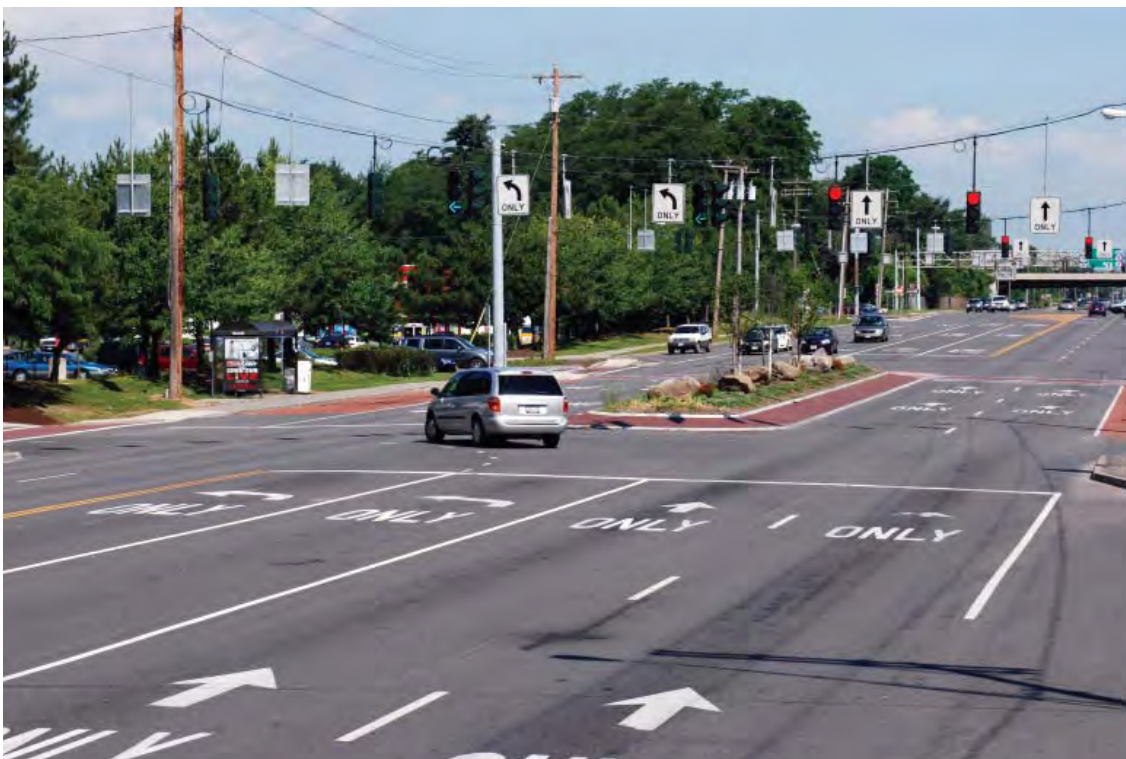
Figure 7-10. Urban Arterial with Dual Left-Turn Lanes
