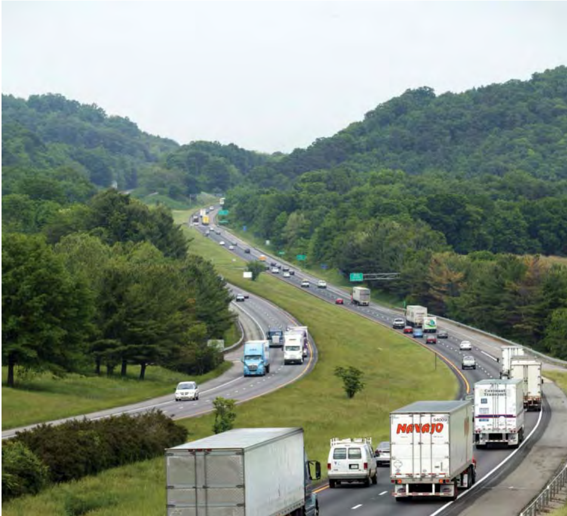
Figure 8-1. Typical Ground-Level Rural Freeway
