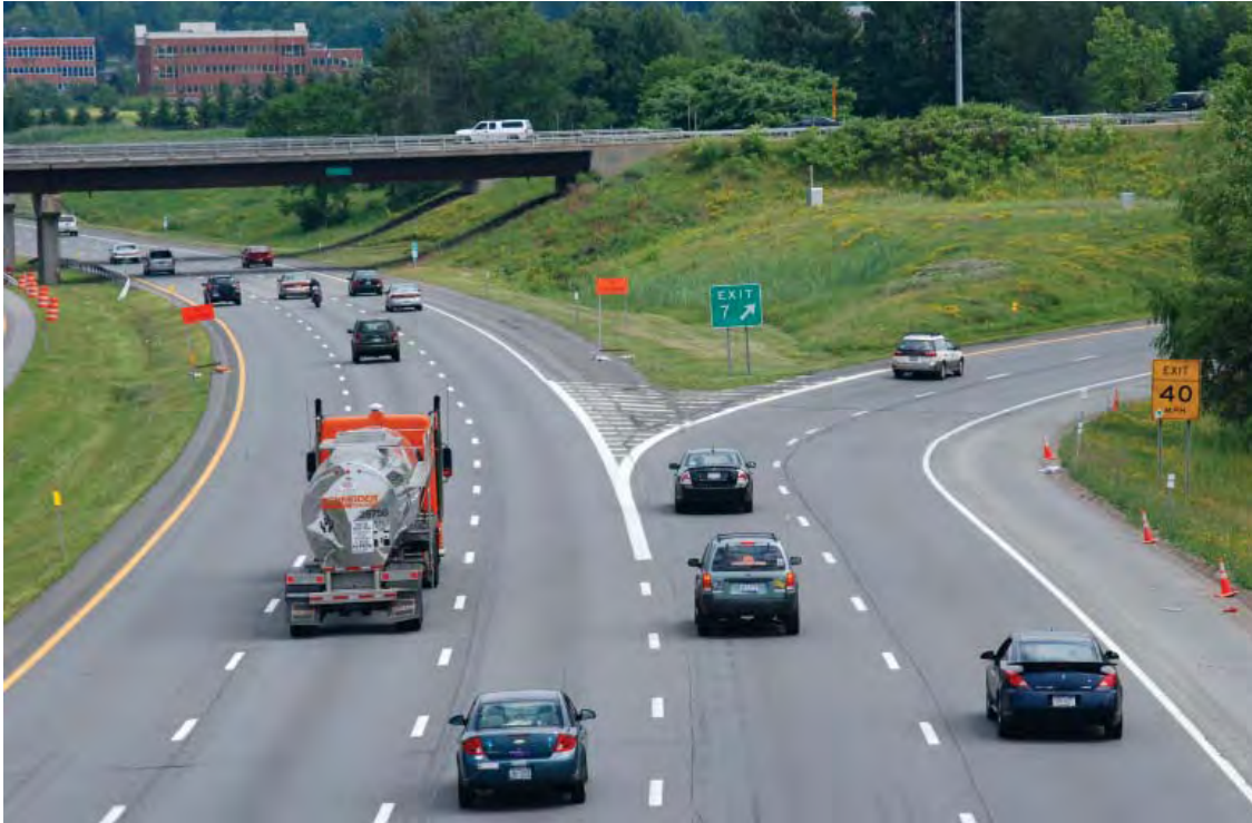
Figure 10-66. Gore Area, Two-Lane Exit
