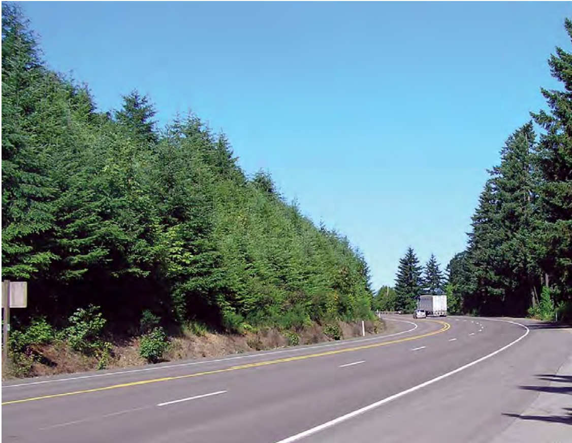
Figure 7-1. Climbing Lane on Two-Lane Rural Arterial
