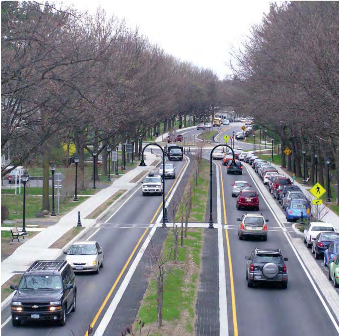
Figure 7-9. Divided Arterial Street with Parking Lane
