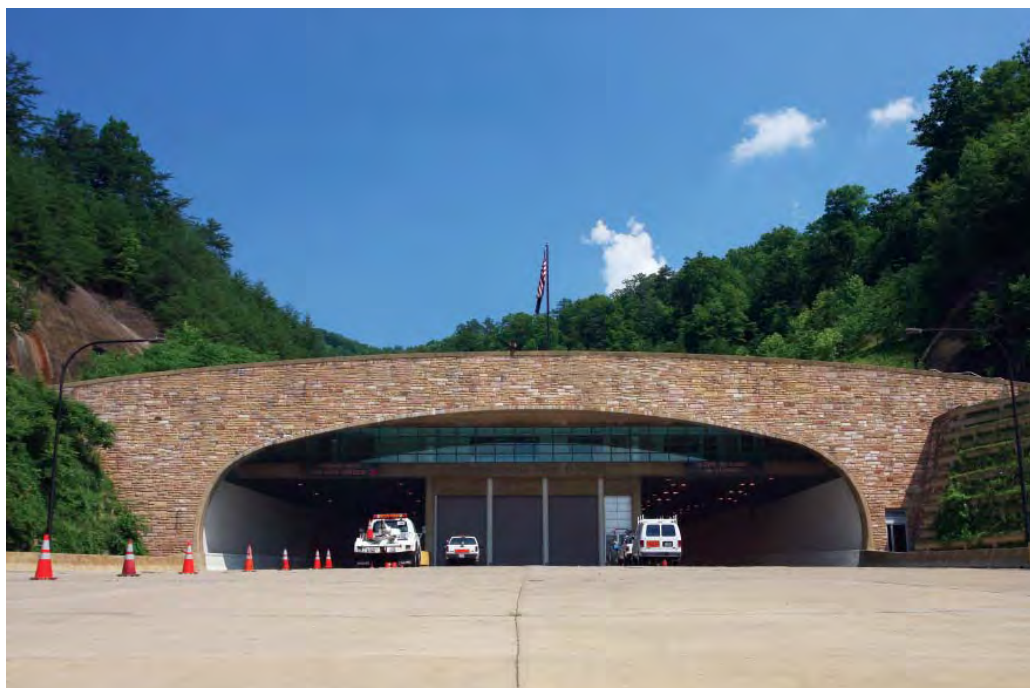
Figure 4-16. Entrance to a Freeway Tunnel
