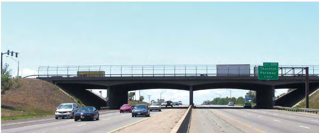
Figure 10-4. Typical Grade Separation Structure with Open-End Span
