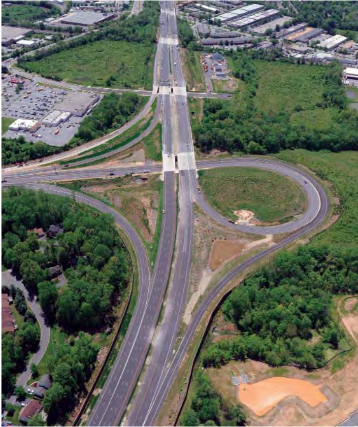
Figure 10-14. Trumpet Freeway-to-Freeway Interchange
