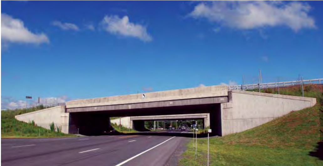
Figure 10-3b. Typical Grade Separation Structures with Closed Abutments
