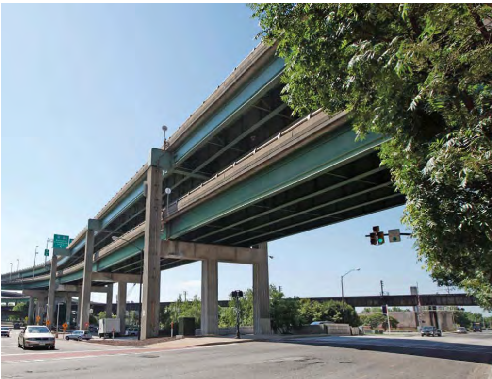
Figure 8-11. Two-Level Viaduct Freeway
