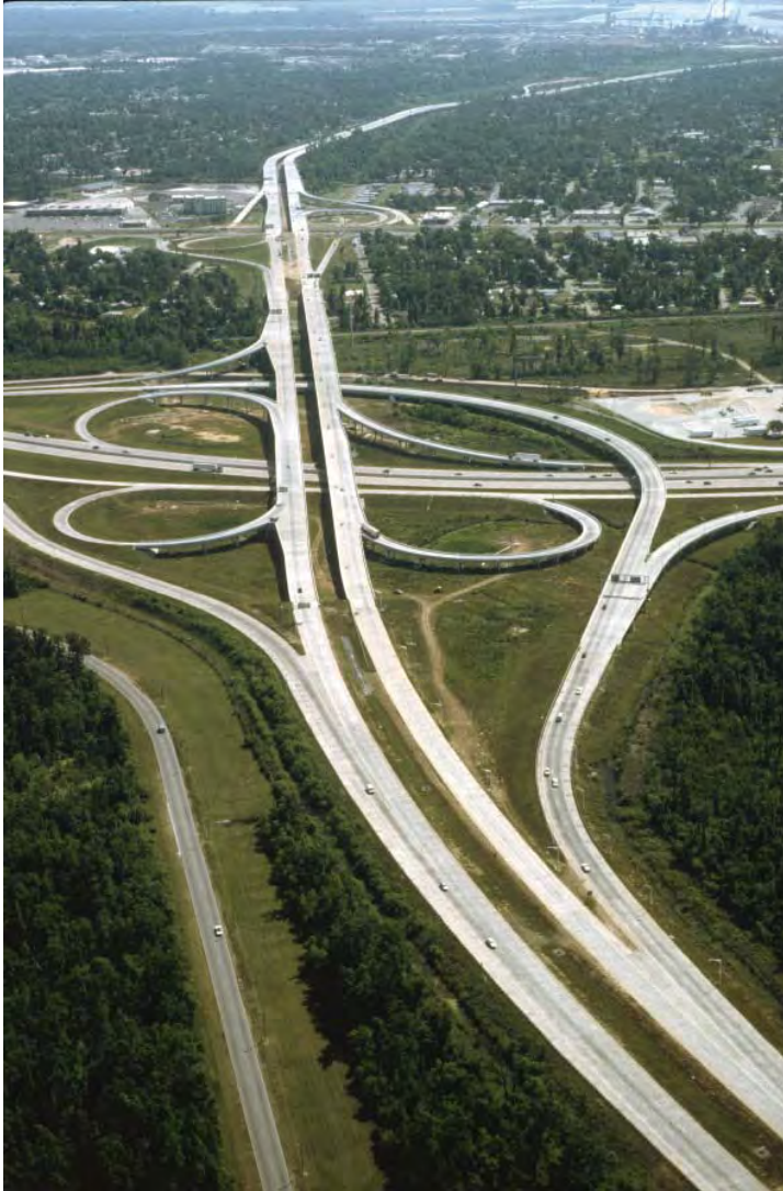
Figure 10-42. Cloverleaf Interchange with Semidirect Connection
