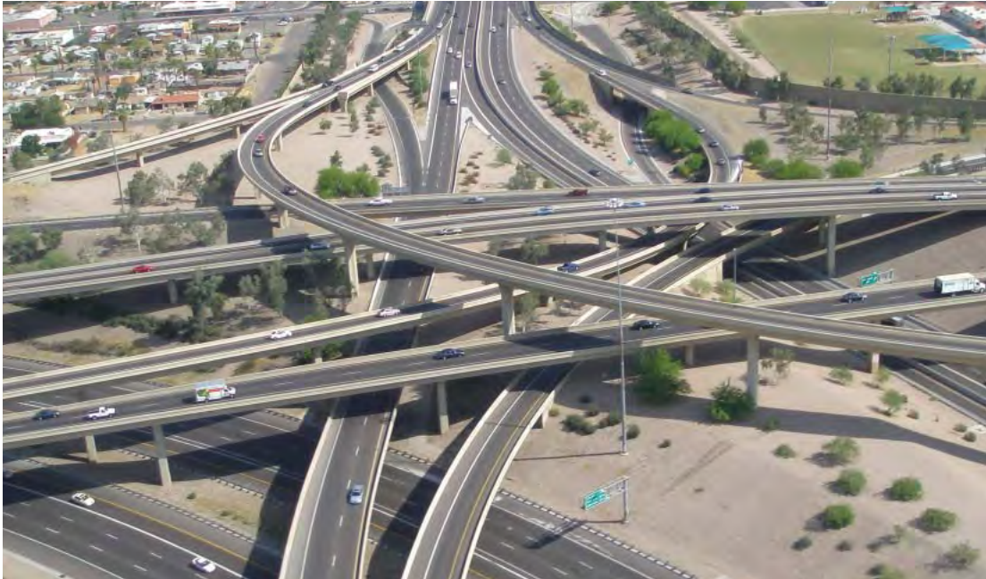
Figure 10-37. Four-Level Directional Interchange
