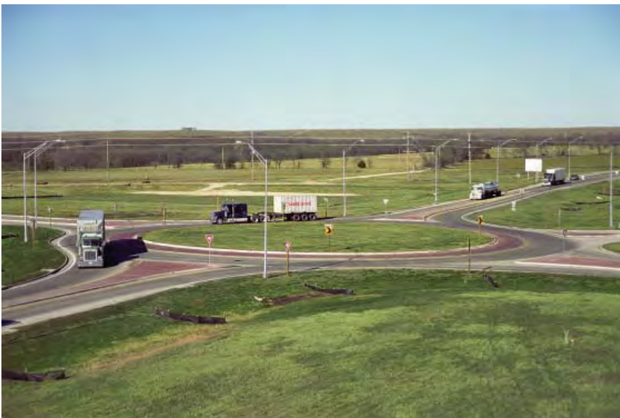
Figure 9-69. Typical Roundabout in a Rural Setting
