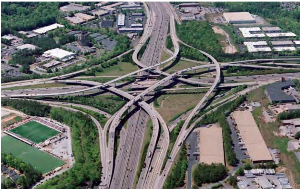
Figure 10-36. Four-Level Directional Interchange
