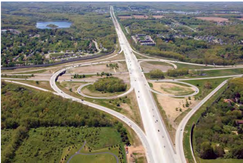
Figure 10-41. Four-Leg Interchange, Cloverleaf with a Semidirect Connection
