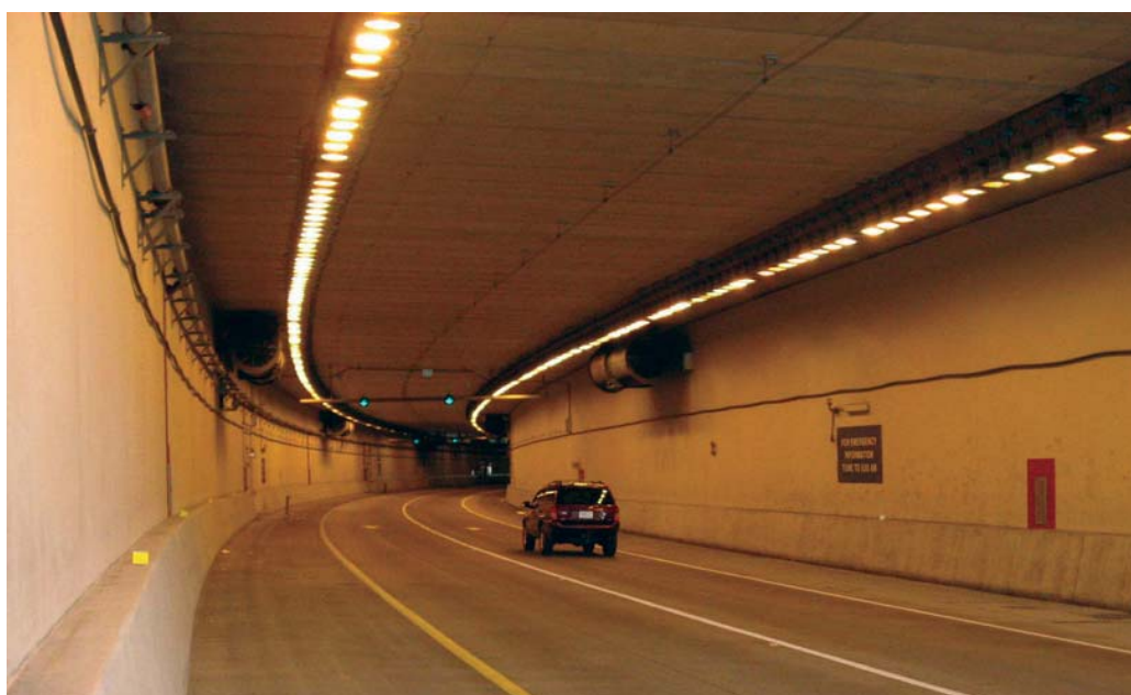
Figure 4-17. Interior of a Two-Lane Directional Tunnel
