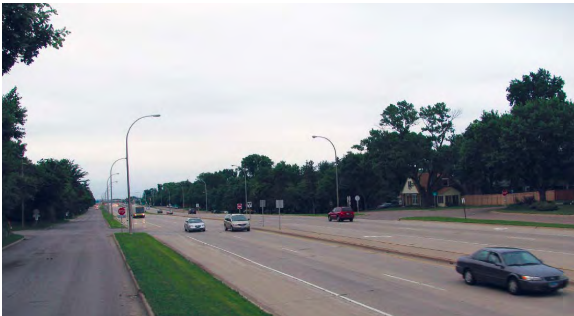
Figure 7-11. Divided Arterial Street with Two-Way Frontage Road
