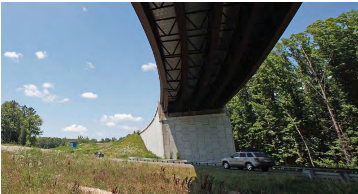
Figure 10-3a. Typical Grade Separation Structures with Closed Abutments
