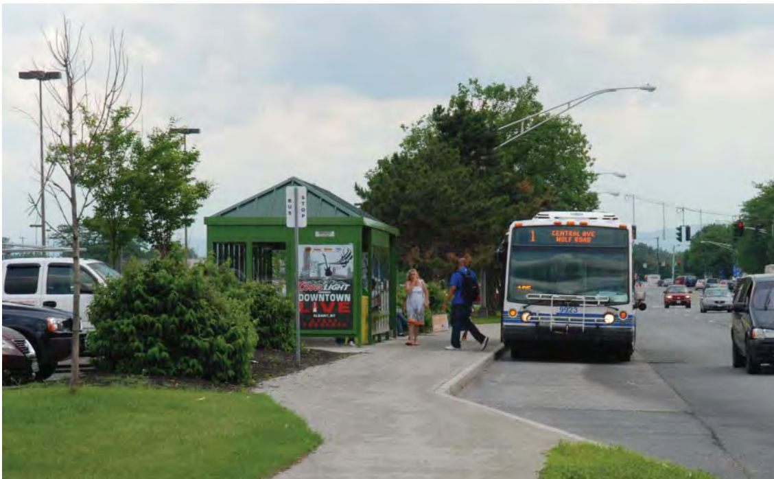
Figure 4-23. Midblock Bus Turnout
