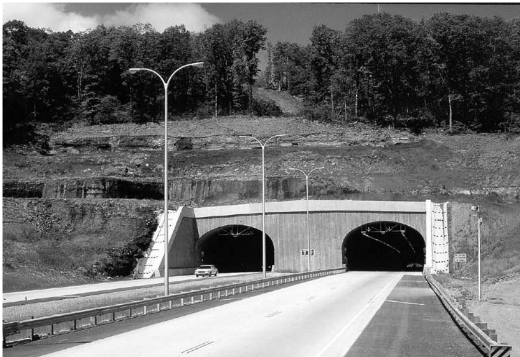
Exhibit 4-19. Entrance to a Freeway Tunnel
