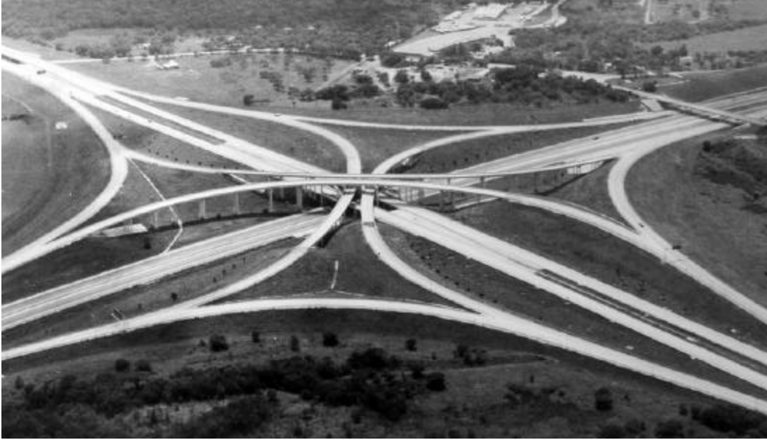
Exhibit 10-36. Four-Level Directional Interchange
