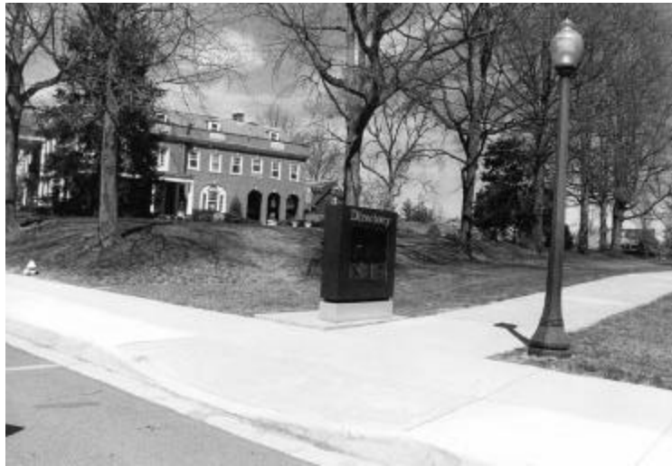
Exhibit 4-25. Sidewalk Curb Ramp at Midblock
