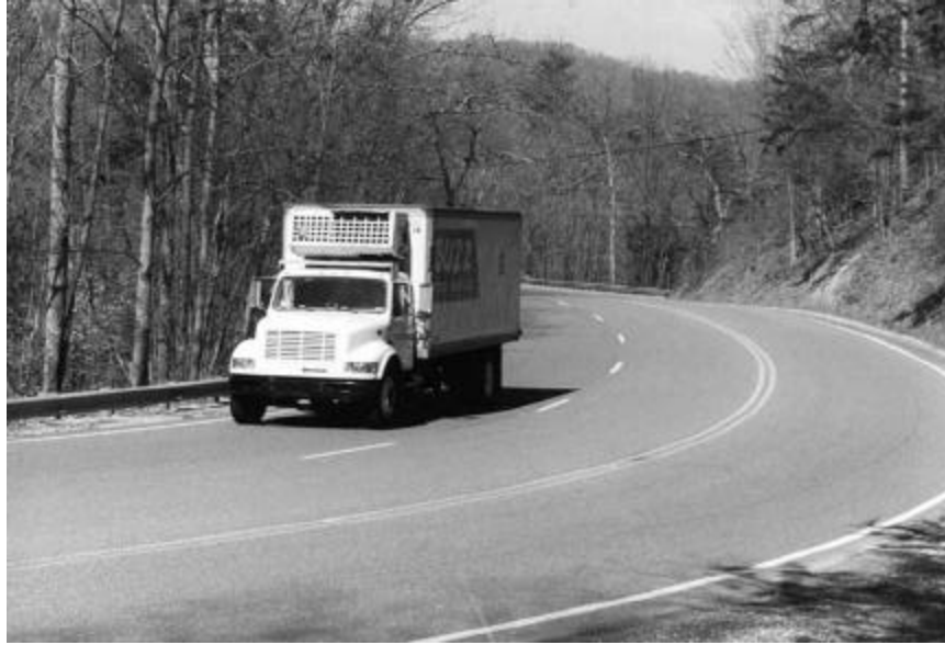
Exhibit 7-4. Climbing Lane on Two-Lane Rural Arterial
