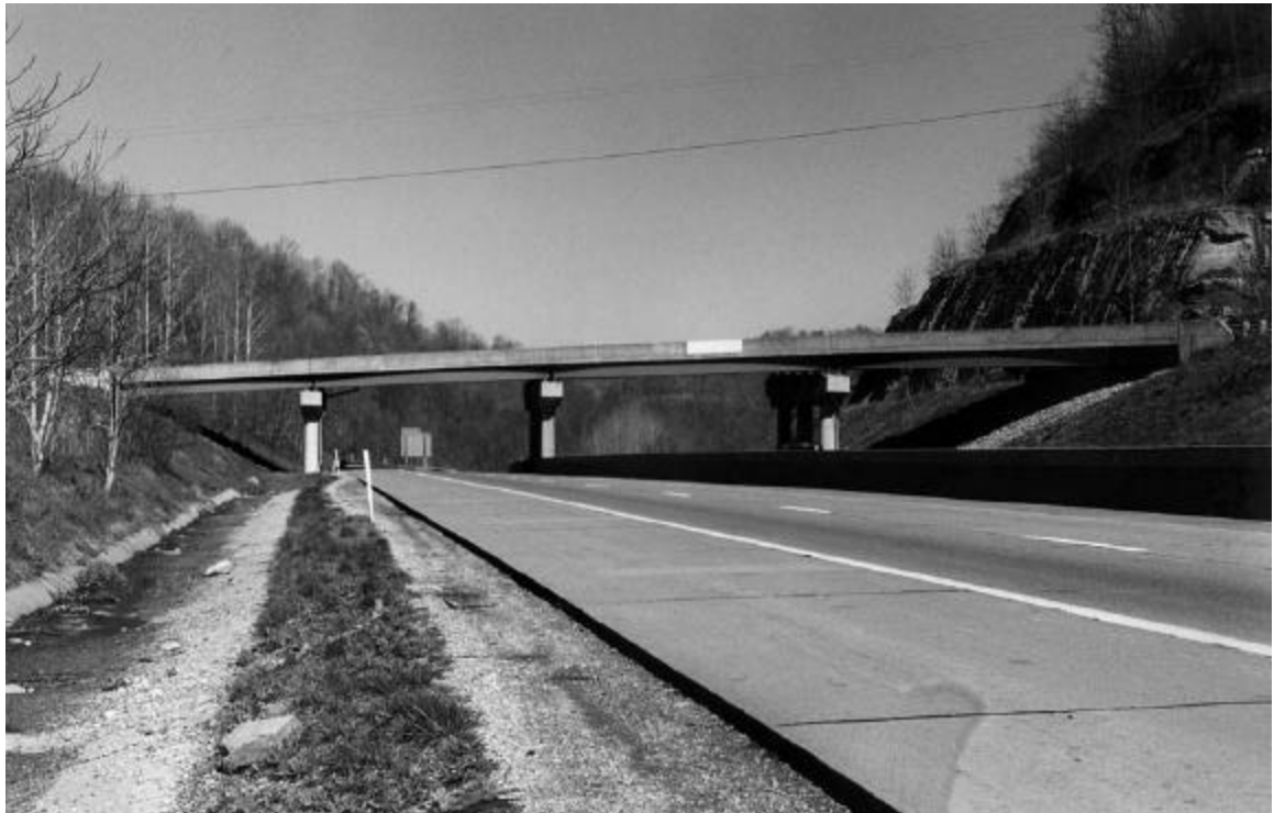
Exhibit 10-4. Typical Grade Separation Structure With Open-End Span
