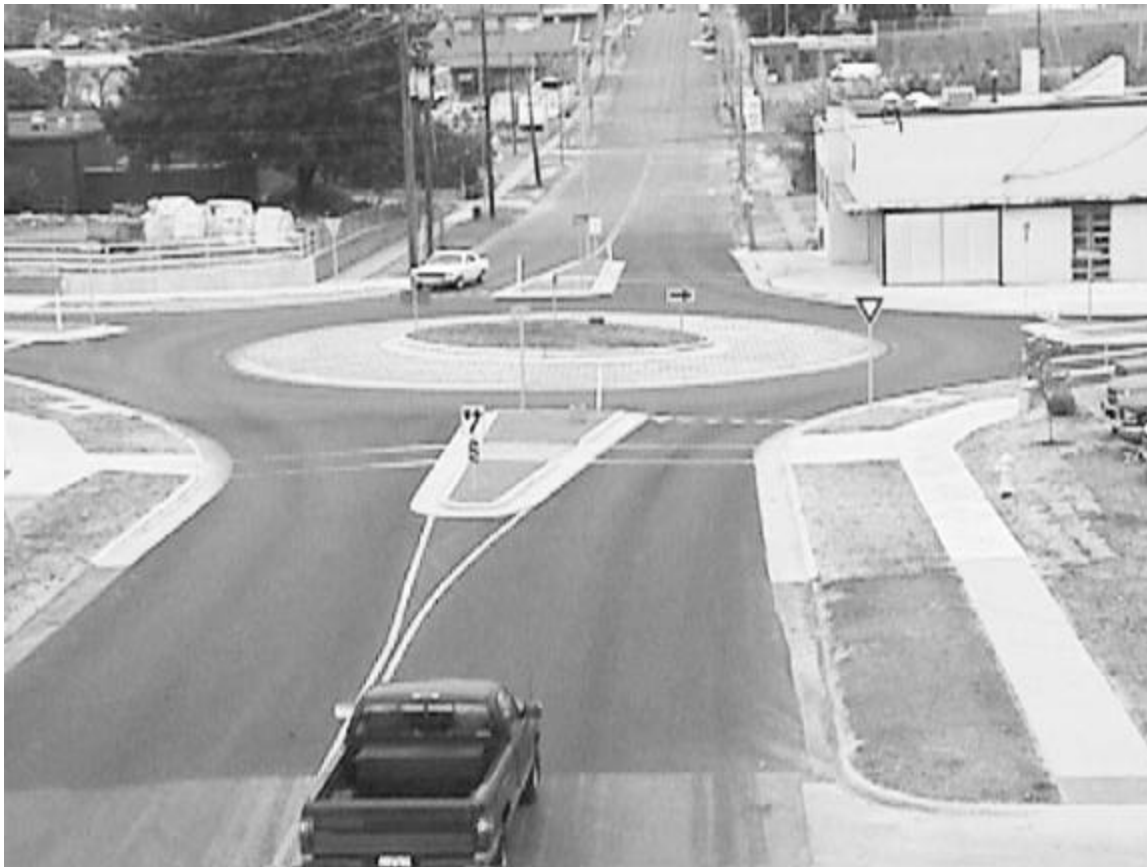
Exhibit 9-16. Typical Modern Roundabout
