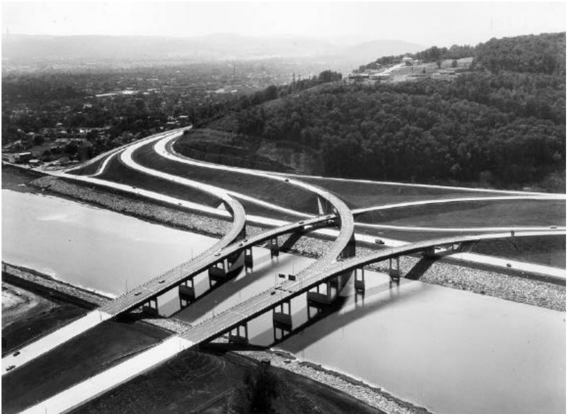
Exhibit 10-13. Directional Three-Leg Interchange of a River Crossing
