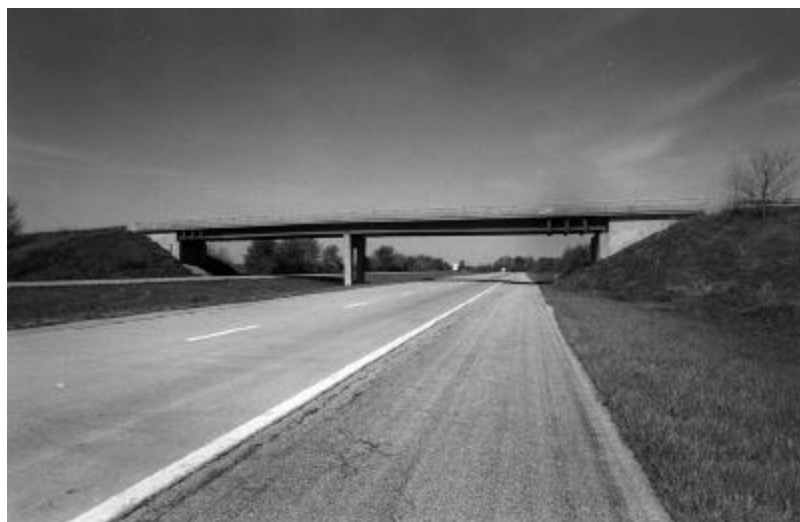
Exhibit 10-3. Typical Grade Separation Structures With Closed Abutments
