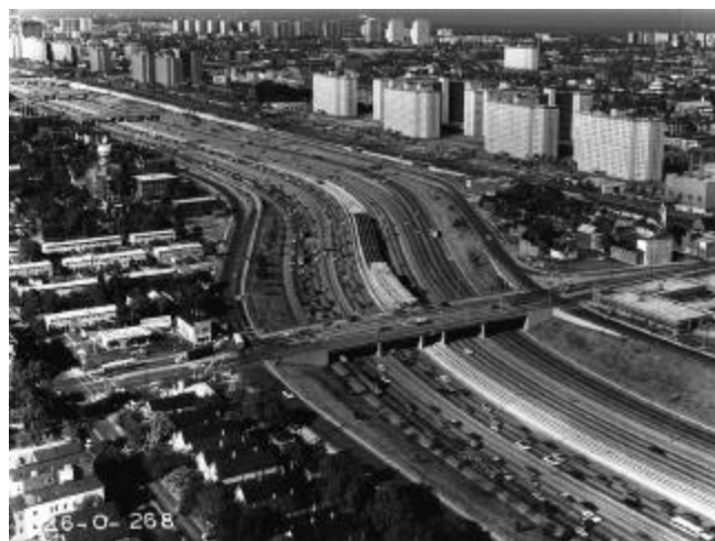
Exhibit 8-25. Dual-Divided Freeway With a 4-3-3-4 Roadway Arrangement
