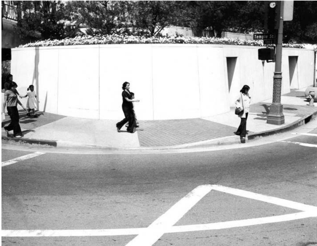
Exhibit 4-23. Sidewalk Curb Ramp at Middle of Radius—Discouraged Where Pedestrian and/or Vehicular Volumes are Moderate to High
