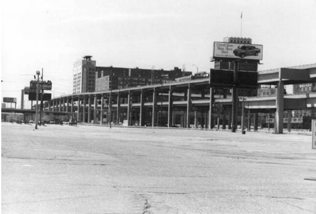
Exhibit 8-13. Two-Level Viaduct Freeway
