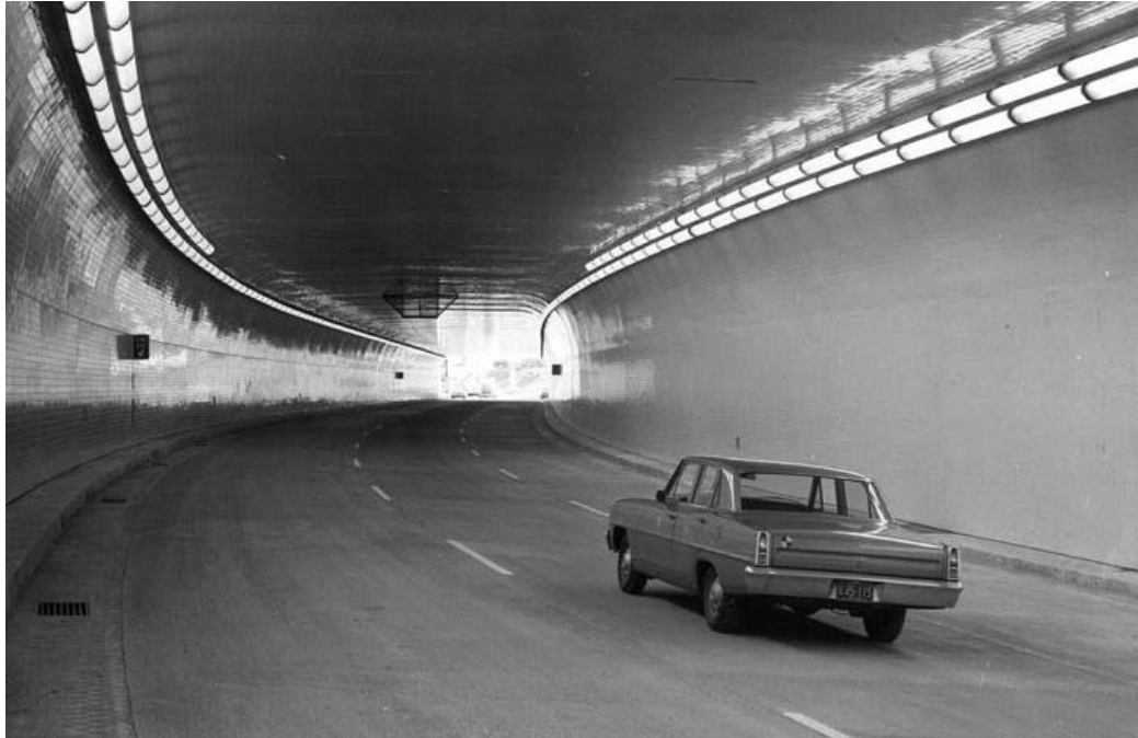
Exhibit 4-20. Interior of a 3-lane One-way Tunnel
