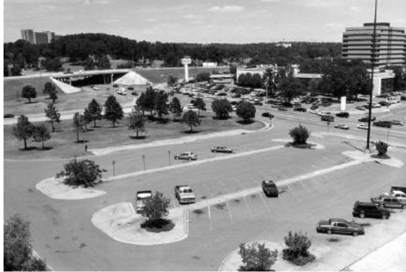
Exhibit 4-30. Typical Park-and-Ride Facility
