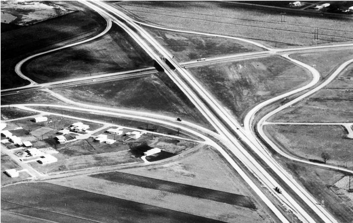
Exhibit 10-20. Existing Four-Leg Interchange With Diamond Stage Construction
