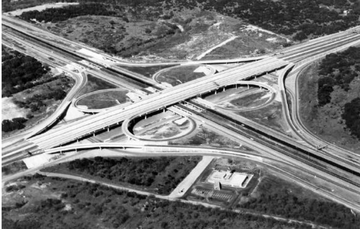
Exhibit 10-42. Freeway with a Three-Level Cloverleaf Interchange
