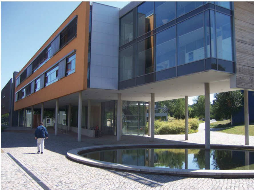
Fig. 7.2 Exterior view of the research institute (From Sailer 2010, p. 83. Copyright 2010 by K. Sailer)
