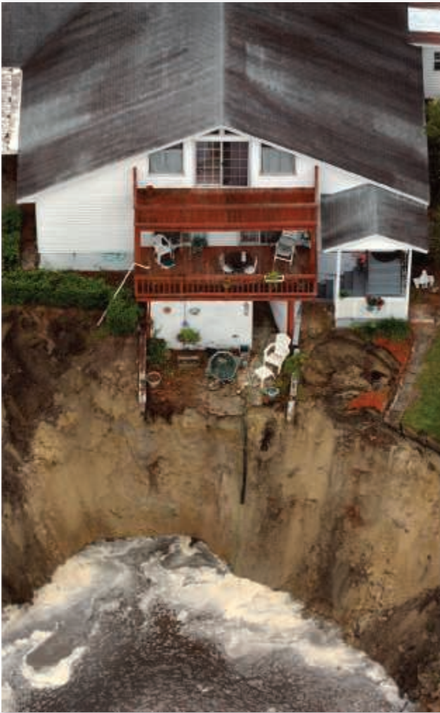
Figure 3.46 Sinkholes can be geologic hazards. This sinkhole formed suddenly in the backyard of a home in Lake City, Florida. Sinkholes such as this one form when the roof of a cavern collapses. (Jon M. Fletcher/The Florida Times-Union/AP Images)
