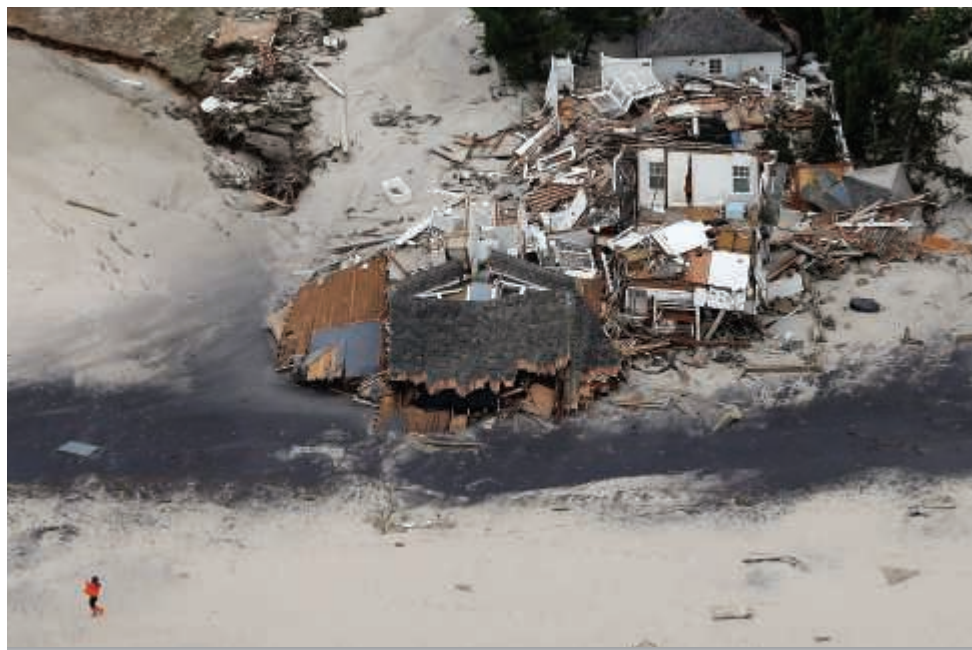
Figure 10.8 Hurricane Sandy A portion of the New Jersey shoreline shortly after this huge storm, unofficially called "Superstorm Sandy," made landfall just south of New York City in late October 2012. The extraordinary storm surge caused much of the damage pictured here. Many shoreline areas are intensively developed. Often the shifting shoreline sands and the desire of people to occupy these areas are in conflict. There is more about hurricanes and hurricane damage in Chapter 14. (Photo by Mario Tama/Getty Images)
