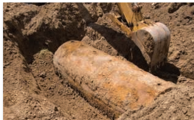
Figure 3.42 Potential sources of contamination Sometimes materials leached from landfills and leaking gasoline storage tanks contaminate an aquifer. (Landfill photo by Picsfive/Shutterstock; storage tank photo by Earth Gallery Environment/Alamy)
