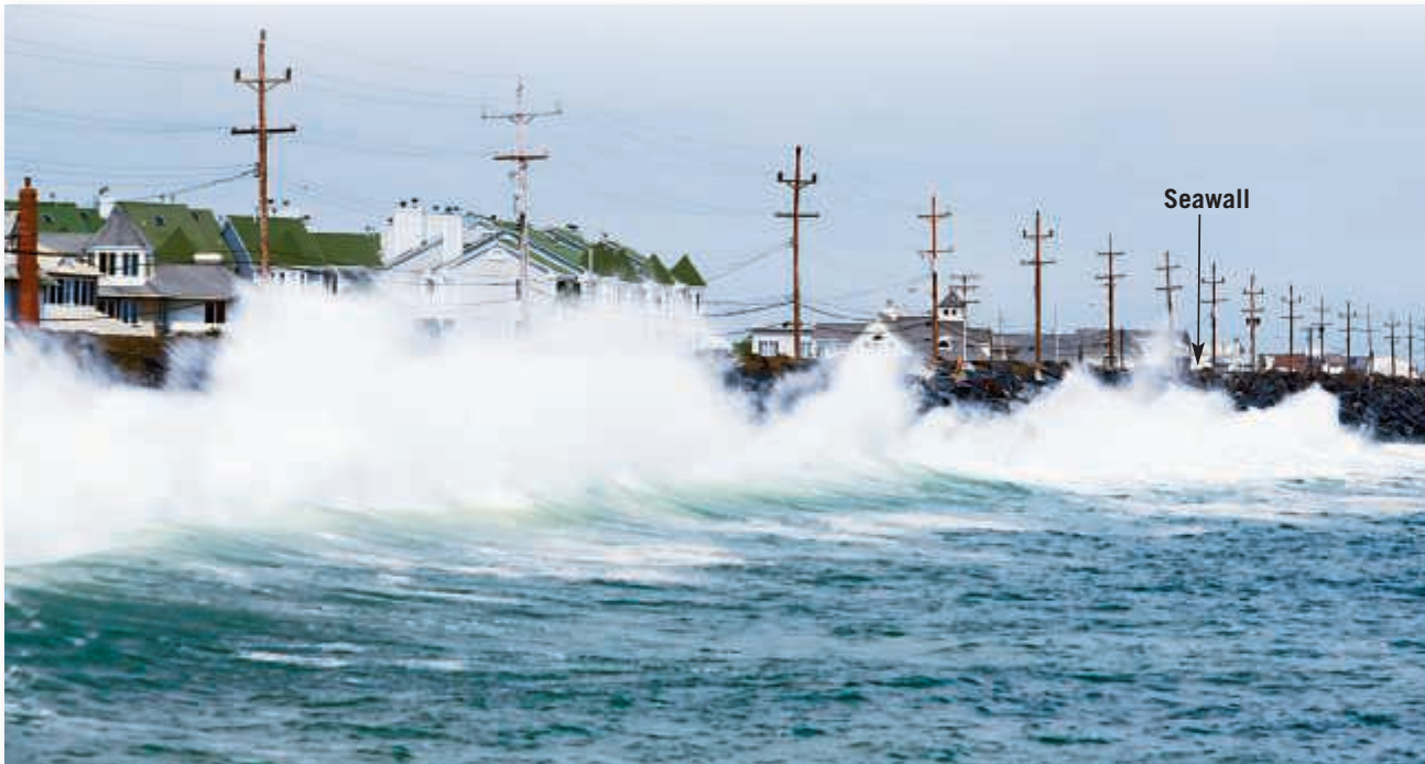
Figure 10.27 Seawall Seabright in northern New Jersey once had a broad, sandy beach. A seawall 5 to 6 meters (16 to 18 feet) high and 8 kilometers (5 miles) long was built to protect the town and the railroad that brought tourists to the beach. After the wall was built, the beach narrowed dramatically. (Photo by Rafael Macia/Science Source)
