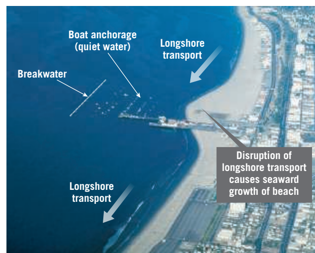
Figure 10.26 Breakwater Aerial view of a breakwater at Santa Monica, California. The structure appears as a line in the water behind which many boats are anchored. The construction of the breakwater disrupted longshore transport and caused the seaward growth of the beach. (Photo by University of Washington Libraries, Special Collections, KC8275)
