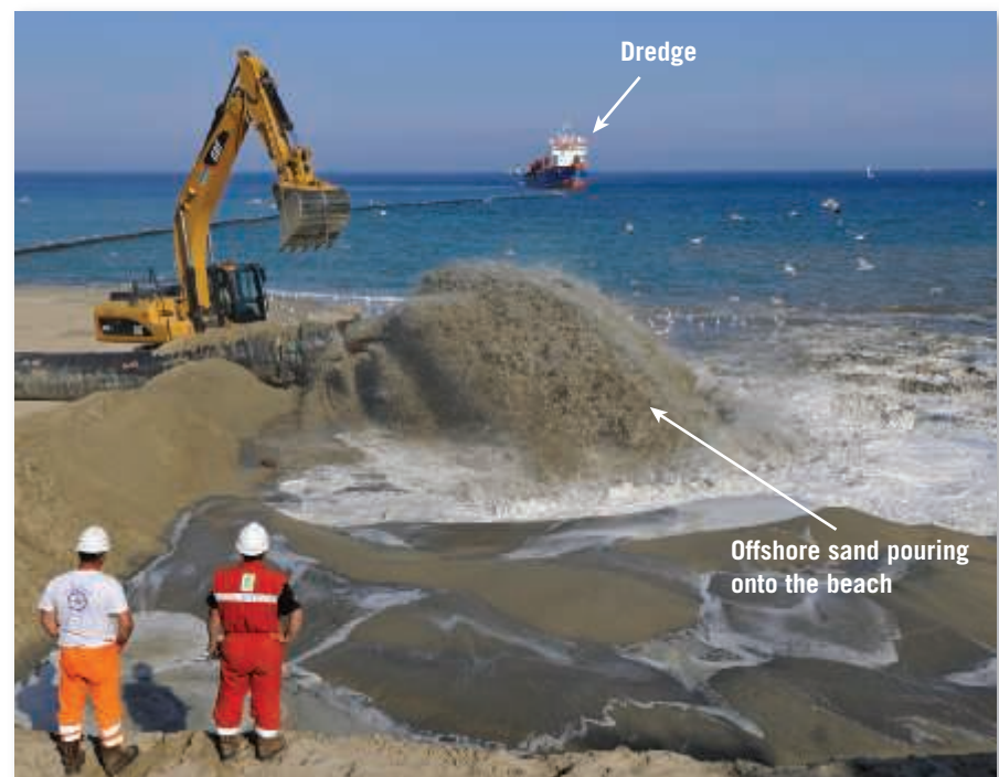
Figure 10.28 Beach nourishment If you visit a beach along the Atlantic coast, it is more and more likely that you will walk into the surf zone atop an artificial beach. (Photo by Michael Weber/Image Broker/Alamy Images)
