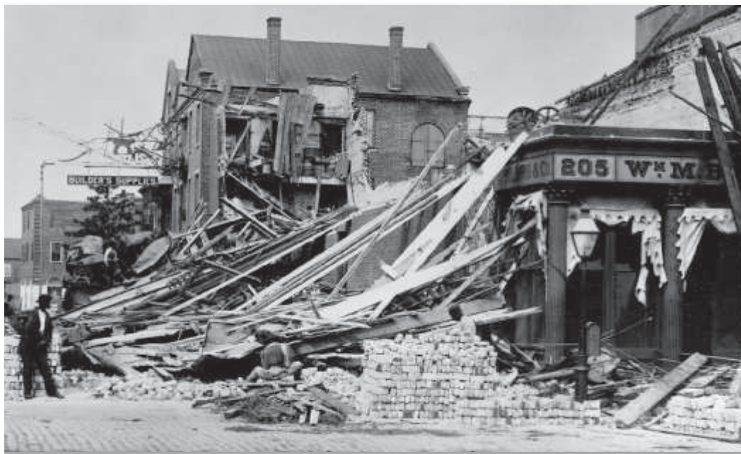
Figure 6.15 Damage to Charleston, South Carolina, caused by the August 31, 1886, earthquake (Photo courtesy of USGS)
