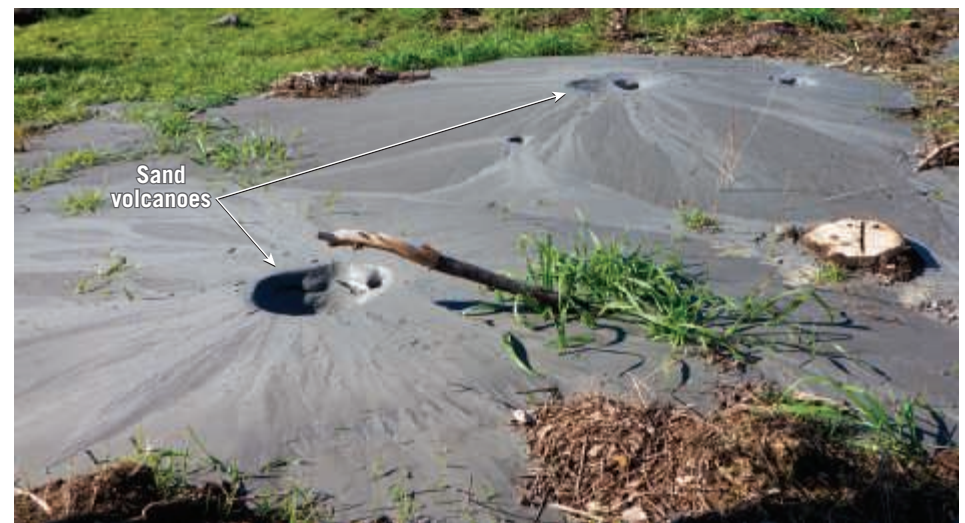
Figure 6.27 Liquefaction These “sand volcanoes,” produced by the Christchurch, New Zealand, earthquake of 2011, formed when “geysers” of sand and water shot from the ground, an indication that liquefaction occurred. (Photo by Diarmuid/Alamy)
