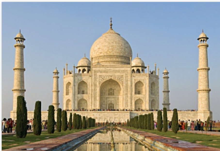
Figure 2.35 Marble, because of its workability, is a widely used building stone. The exterior of India’s Taj Mahal is constructed primarily of the metamorphic rock marble. (Photo by Sam Dacruz/Shutterstock)
