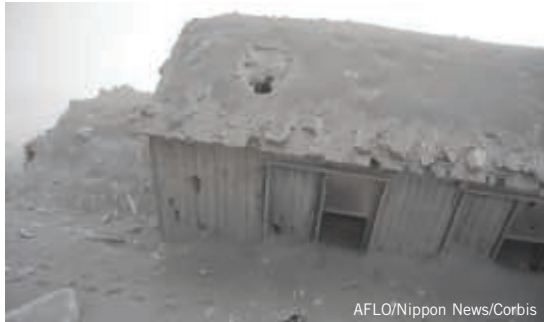
Ash and other pyroclastic materials can collapse roofs, or completely cover buildings.
