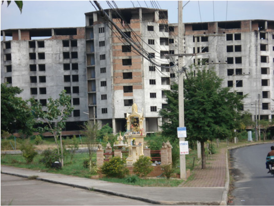
Fig. 13.2 Failed construction project, Chiang Mai
