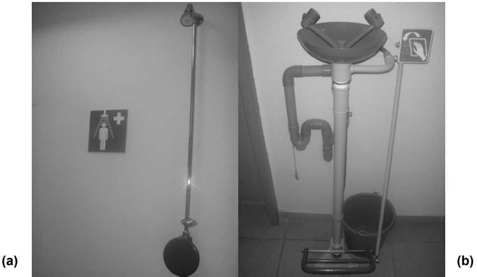
Fig. 18.1. Emergency decontamination shower (a) and eye wash station (b) for emergency decontamination at work (Source: Laboratory of Dr Denis Josse).
