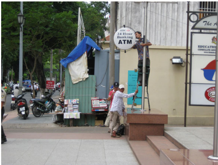
Fig. 8.1 Setting up the ATM network. Photograph by the author
