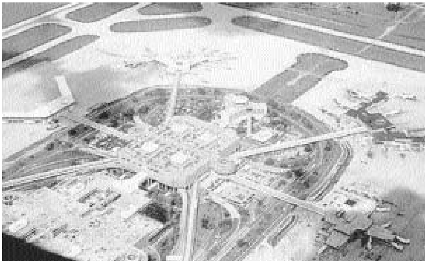
Figure 6-11. Example of airside-landside concept, Tampa International Airport. (Figure courtesy Hillsborough County Airport Authority)
