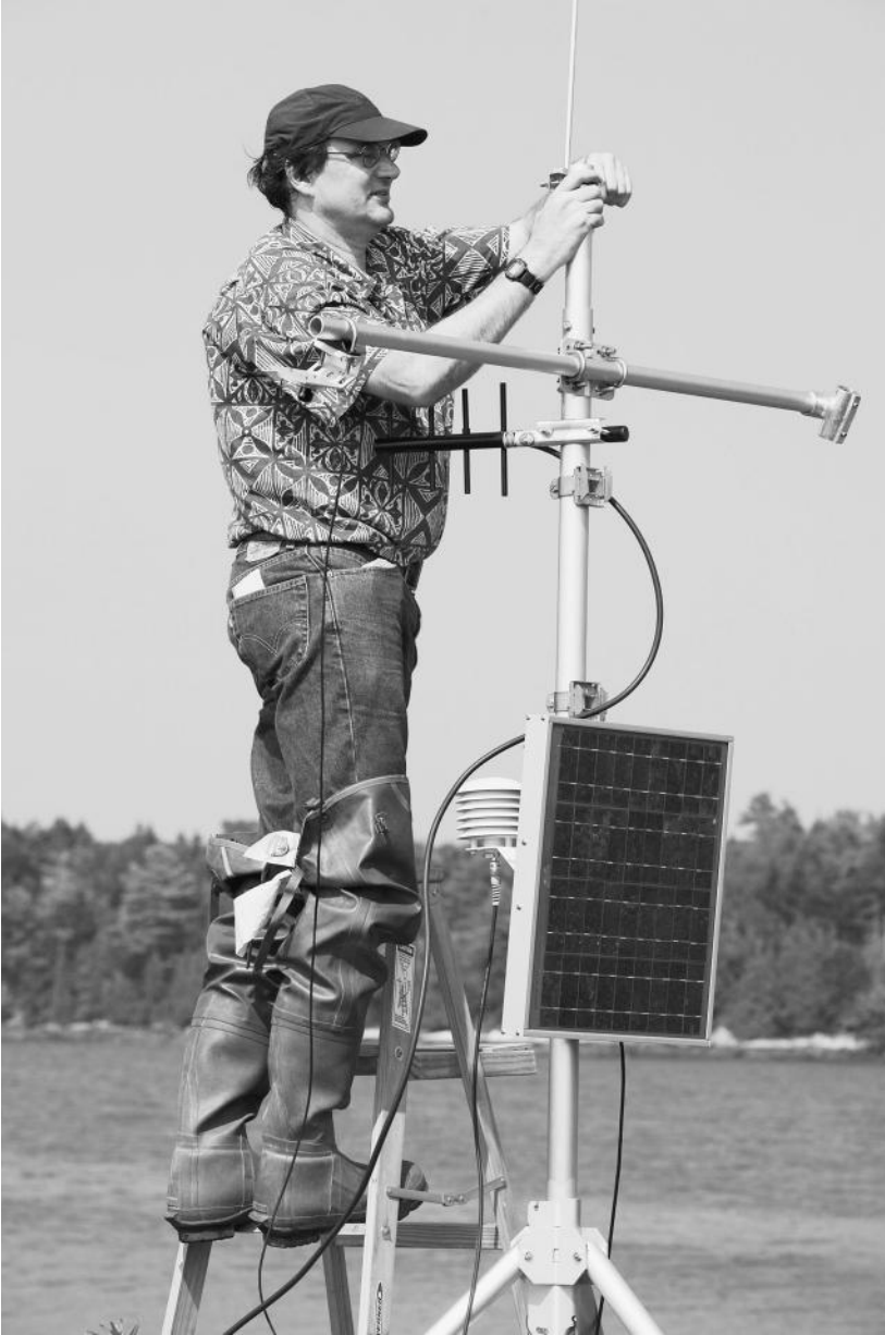
A professor stands on a ladder while constructing a weather monitoring station. ( James Marshall, The Image Works )
