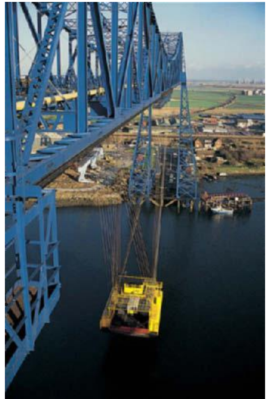
Plate 10 Bridges. View of the transporter bridge which spans the River Tees at Middlesbrough in the UK. The bridge was constructed in 1911 to replace the old ferryboat crossing there. It is a total of 260m wide and around 68m high. A cradle suspended from the main girder ferries cars and passengers across the 174m stretch of water in about 2 minutes. (With permission from Science Photo Library).
