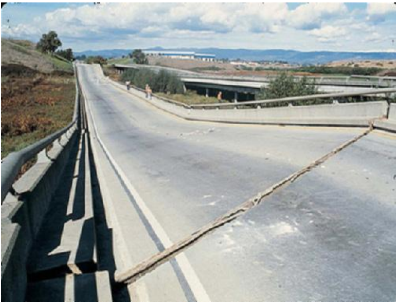
Plate 29 Earthquake Excitation and Response of Buildings. Earthquake damage. Collapsed road bridges after an earthquake. Earthquakes are caused when sections of the earth (tectonic plates) move against each other to relieve stress. Photograph of highway near Watsonville in California, USA, in 1990. California lies on the boundary between the North American and Pacific plates. (With permission from Science Photo Library).
