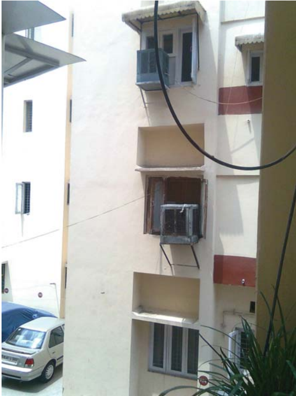
Plate 29 Many residences in India, like this apartment building in Delhi, use “coolers” to battle the summer heat. The coolers operate on a reservoir of water and can be fertile mosquito breeding grounds if not maintained regularly. (The Dynamics of Urban Malaria in India. Photo by Anubha Wadhwa.)
