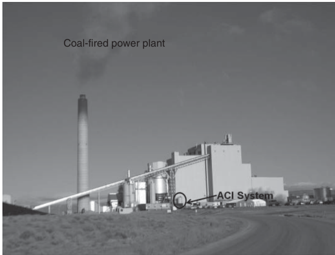
Figure 18.1 Perspective on ACI system in relation to other air pollution control equipment at a coal-fired power plant.
