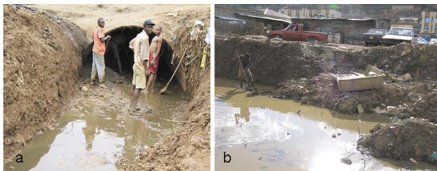
Fig. 6.17 Local initiatives to improve drainage conditions: (a) opening up of closed culvert; (b) excavation of Nyabugogo River
