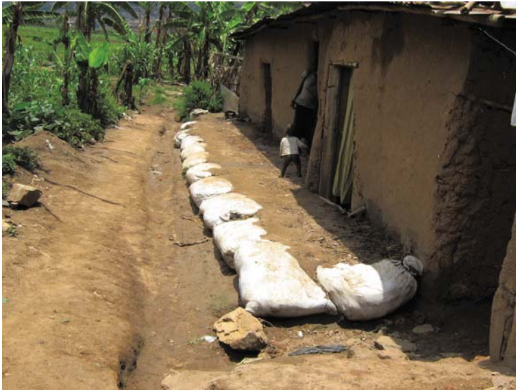
Fig. 6.16 Inadequate flood protection measure
