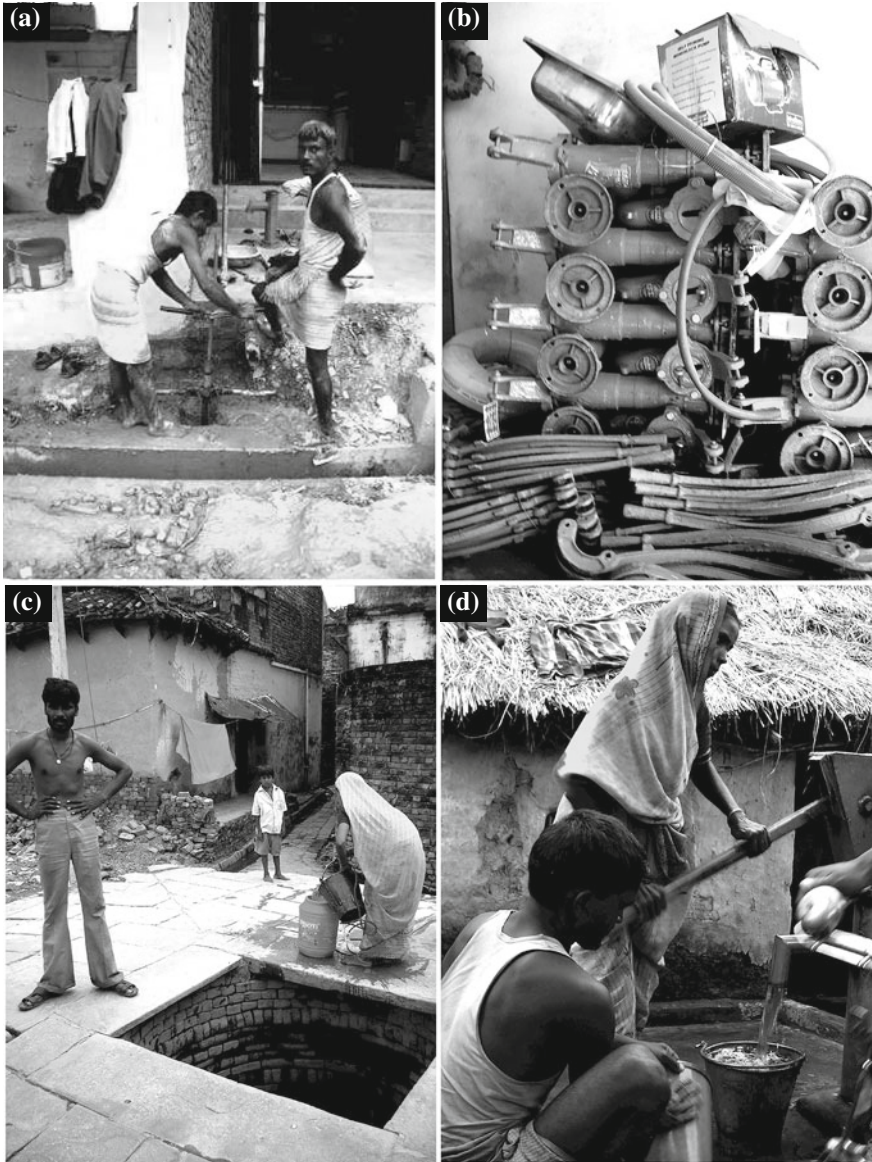
Fig. 4.19 Private alternatives to the water supply network. a Two workers in the process of installing a handpump in front of a house. Although basic, this technology has become extremely popular among households. By purchasing a handpump, the client is freed from the constraints inherent in using public services and this at a relatively low cost. b A growing number of wealthier households are opting to buy electric (or even fuel-powered) pumps, such as that seen on top of the pile of handpumps. This is a much more expensive investment as a deeper borehole is required and a storage tank has to be installed on the roof of the house. These strategies are in stark contrast to those used by inhabitants who cannot afford to buy their own equipment and thus will have to continue to use public handpumps or even traditional wells ( c , d ). Source Author
