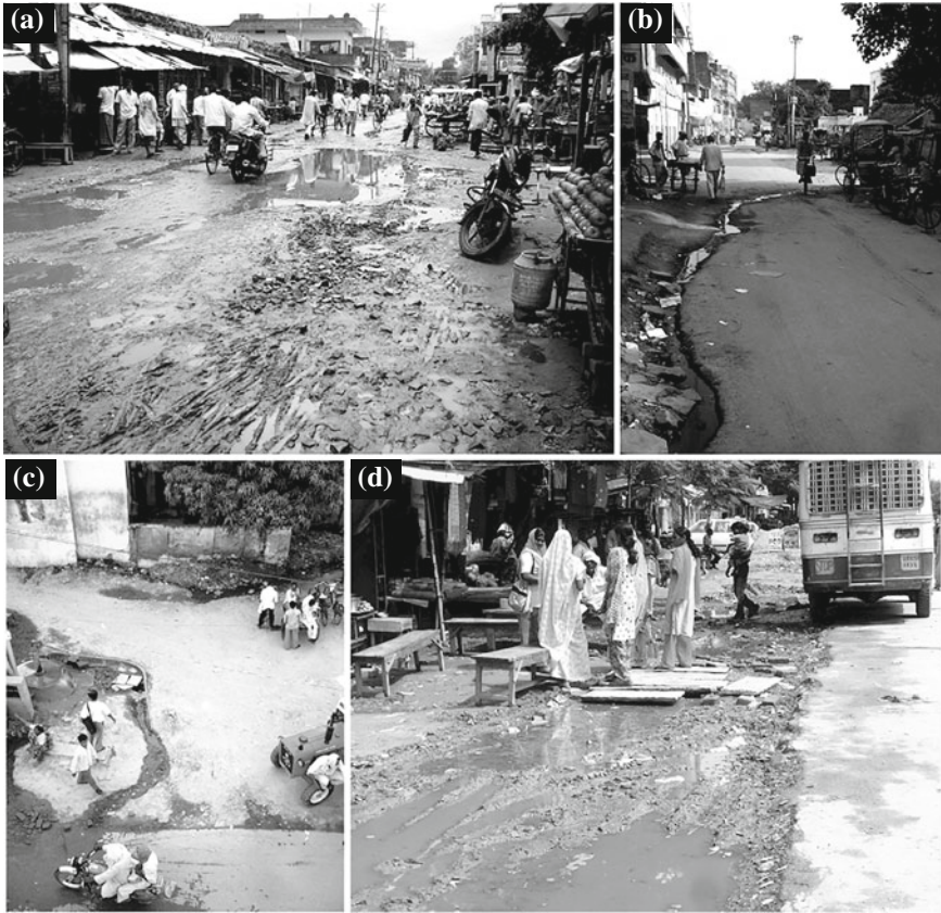
Fig. 4.4 Lack of sewerage. Note As there is no sewage system, wastewater tends to spill into the street (a), where it either flows across the road (b) or collects in pedestrian areas (c). The situation is even worse during the monsoons (d). (All of these photographs were taken in the centre of Chandauli). Source Author
