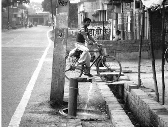
Fig. 4.17 Water supply. Note Water is distributed via the network two to three times a day, depending on the town. This water can sometimes be seen gushing out of taps that have inadvertently been left open, such as at this public water tap in a street in the centre of Phulpur. In addition, the water pressure varies from area to area, dropping as the distance from the water tower increases to the point where there is virtually no pressure at all at the end of the network. Source Author
