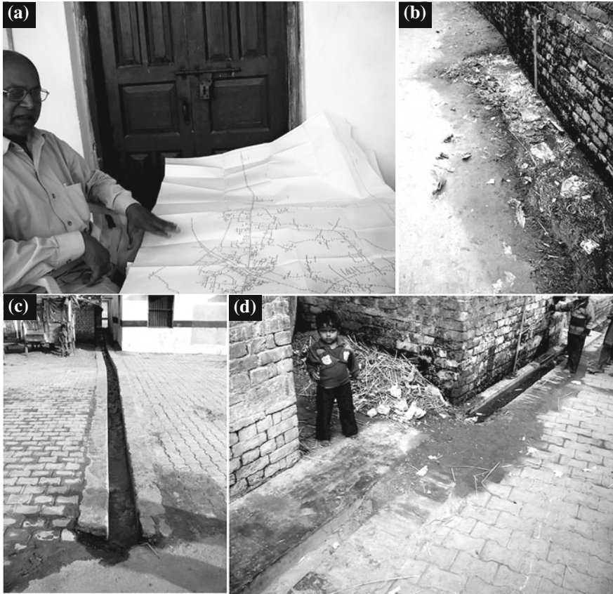
Fig. 4.6 The non-integrated design of nala. Note In Siddarthnagar, the Jal Nigam engineer bemoans the fact that, due to lack of coordination, the construction firms do not work off the town's topographic maps that he himself developed for a project, which was ultimately cancelled (a). He told us that "this would have prevented some of the problems now causing stagnant wastewater to collect in the street!" (b, c). According to the engineer, local residents are also partly responsible for these issues when, for example, they block up a nala to make it easier to cross a road (d). Source Author
