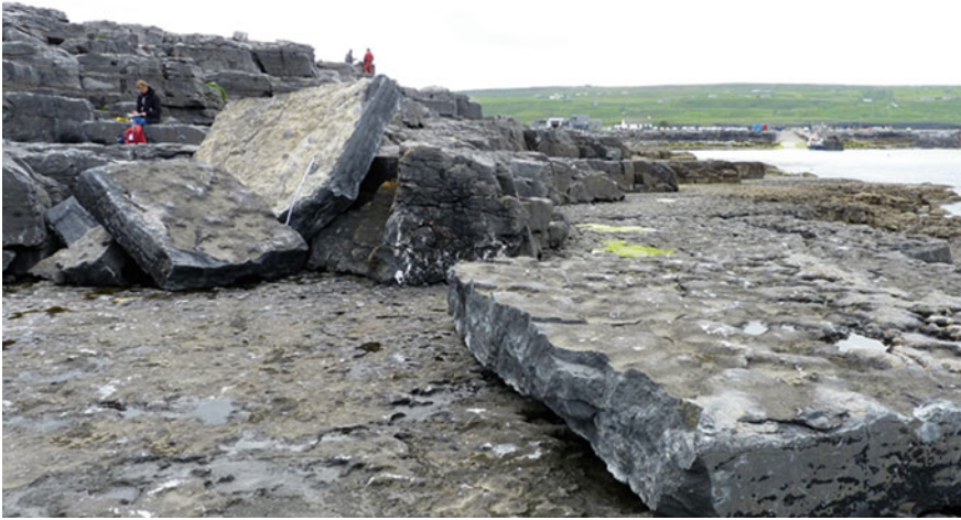
Fig. 3.47 Beside nearly unaffected sections of the cliff coast near Doolin Point and still east of it, significant fresh break outs of large boulders can be seen, like this boulder set with masses of 6.1 tons (with person sitting), 7 tons (steep inclining), and 20.3 tons (in the foreground) as the three largest ones. They represent about 33 tons from a source area nearby, which delivered about 41 tons from an area of 35 m 2 . The difference of 8 tons can be found in the smaller platy boulders below the person in this image ( Image credit D. Kelletat)
