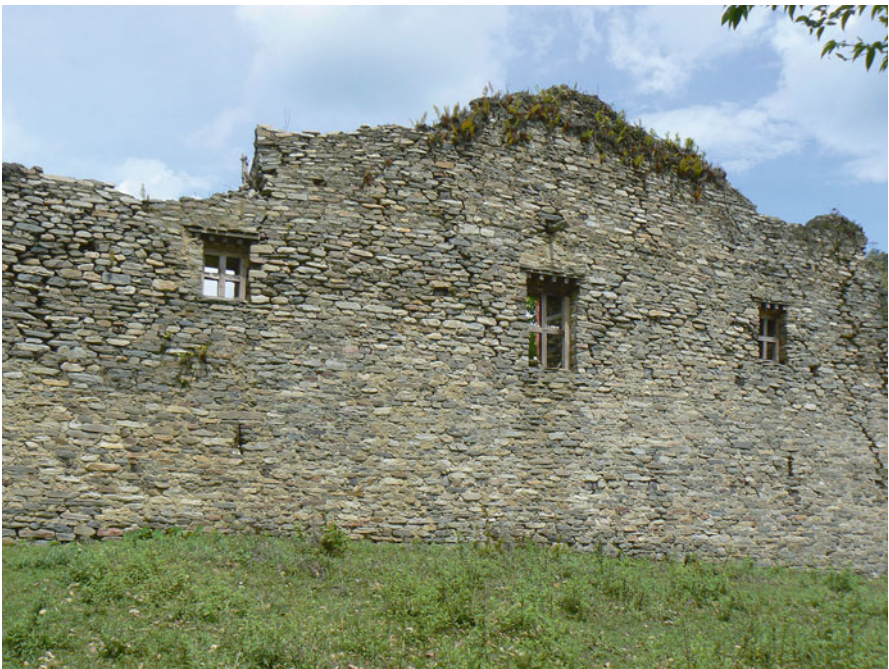
Fig. 3.4 A wall of Taklung Dzong [stag lung rdzong ]: this dzong consisted of three floors, but it was destroyed by an earthquake. It was later partially restored
