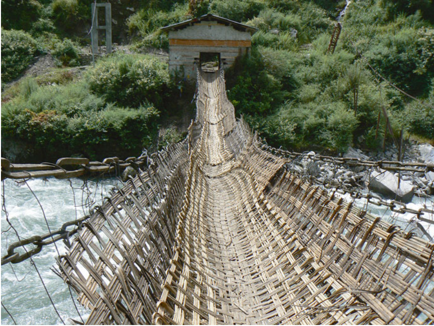
Fig. 3.2 Chaksam [lcags zam] ( lcags means “iron” and zam means “bridge”) was built by Thangtong Gyalpo [thang stong rgyal po] (1361–1485) in the Tawang area
