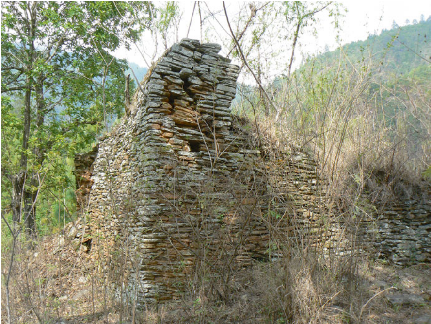
Fig. 2.6 The construction date of Dirkhi Dzong [bde skyid rdzong ] is estimated to be around 1400. The term dzong [ rdzong ] means “fortress”
