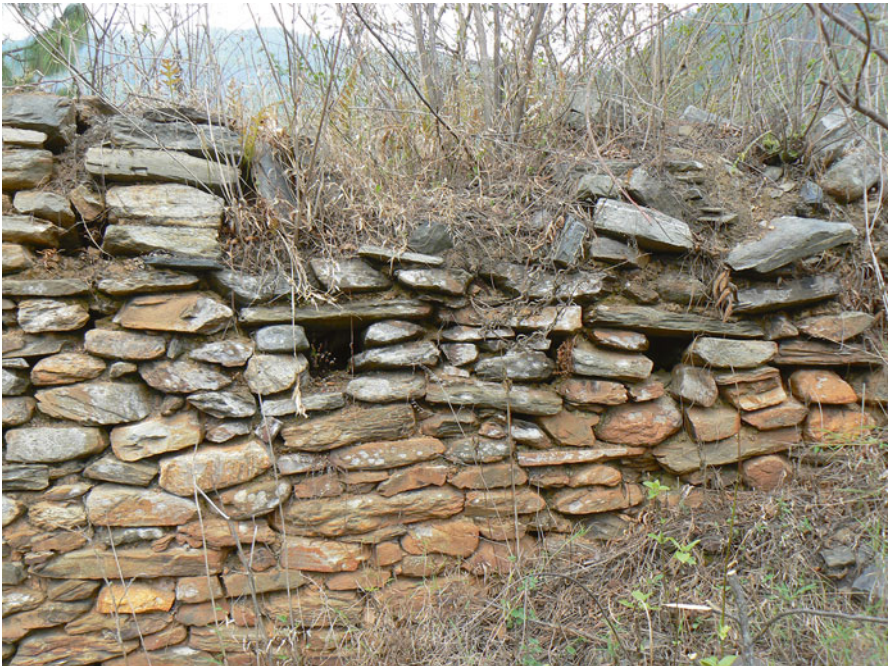
Fig. 2.7 Remains of Dirkhi Dzong [bde skyid rdzong ]: the holes in the wall are thought to be ventilation openings for the kitchens or crenels from which to shoot arrows
