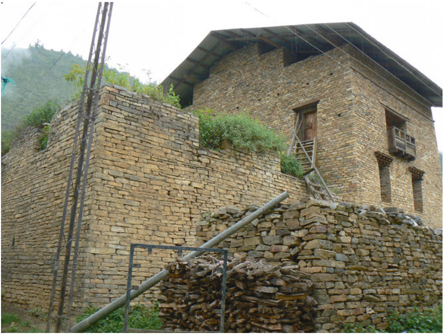
Fig. 3.11 Dirang Dzong [rdi rang rdzong ], the present fortress is believed to have been constructed in 1831 and it was restored in the early 2000s. The photograph shows the central four-story building with crenels. It is used as the dwelling of the dzongpon [rdzong dpon]. The structure visible on the left-hand side of the photograph was used as a jail
