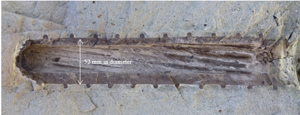
FIGURE 3.61 Failure evident at the cable/grout interface.
