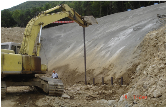
FIGURE 5.46 Setting an antislid pile on site.
