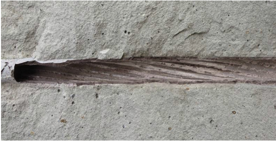
FIGURE 3.46 An example of failure of the cable at the cable/grout interface.
