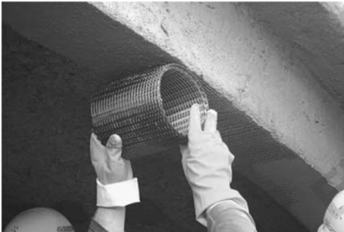
Figure 12. Placing of the textile reinforcement.
