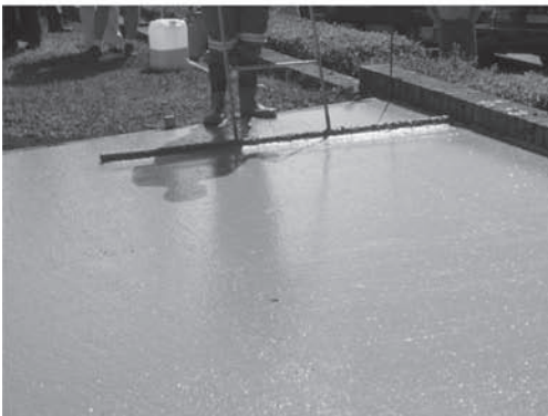
SDC-D: Finishing by rodding surface
