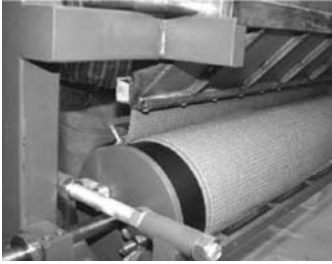
Figure 18. Application of the textile reinforced concrete.
