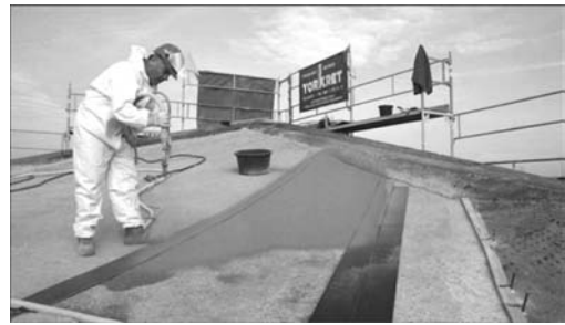
Figure 6. Spraying of a thin layer of fine-grained concrete.
