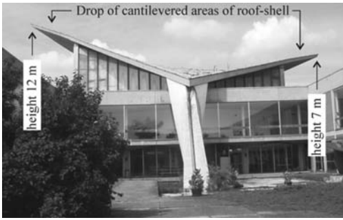
Figure 4. Steel reinforced concrete hyper-shell of FH Schweinfurt (Germany).
