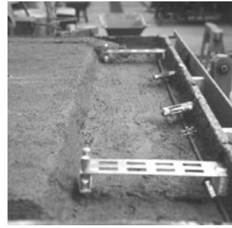
Figure 14. Placement of fixing elements and steel bar.
