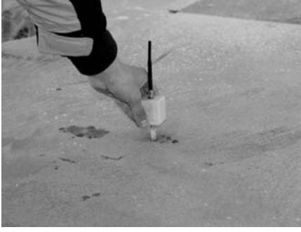
Figure 4. Wireless capillary pressure sensor to be used for on-site measurements.
