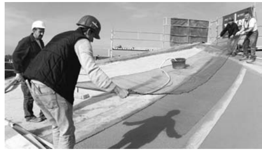
Figure 7. Placing of textile reinforcement.
