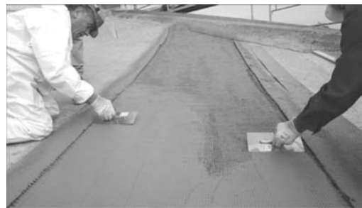
Figure 8. Embedding the textile reinforcement.
