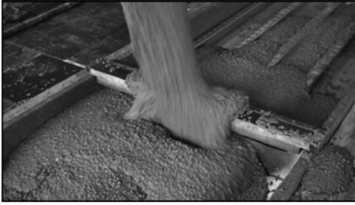
Figure 6. Casting a composite slab with pumped SCLC.
