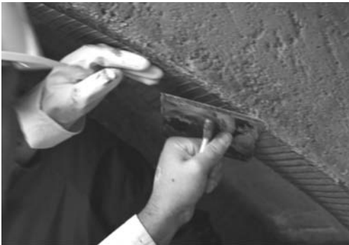
Figure 13. Embedding of the textile reinforcement.
