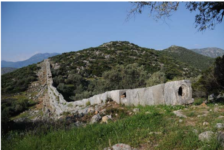
Fig. 1.10 Inverted siphon at Patara. Color version available in Appendix (copyright permission with L.M. Mays)
