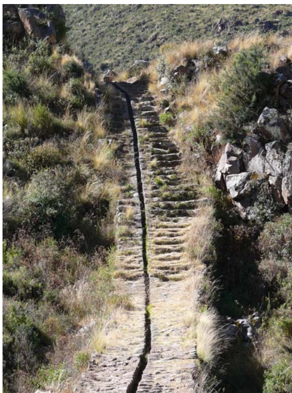
Fig. 9.17 Main aqueduct for Tipon. Note the stair steps on the steep terrain (photo copyright by Yuri Gorokhovich). Color version available in Appendix
