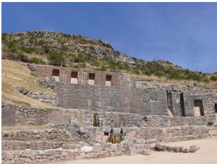
Fig. 9.28 Tambo Machay complex consisting of retaining wall and calvert with dual channels ( in the center of the picture ) (photo copyright by Yuri Gorokhovich)
