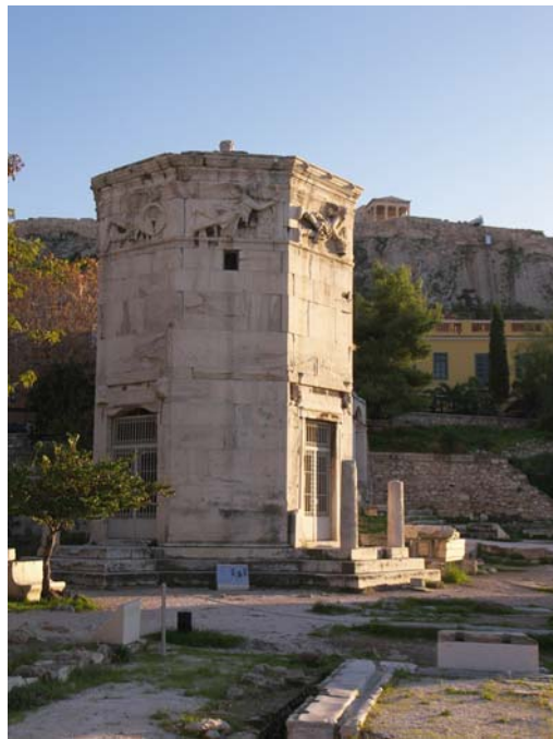
Fig. 1.13 Tower of the Winds. Located below the Acropolis in Athens, designed by the famous astronomer Andronikos of Kyrros to be an elaborate water clock (on the inside). The name is derived from the personifications of the eight winds carved on the eight sides of the building. Originally thought to have been built in the 1st century B.C. during the early Roman Empire, but now many archaeologists think the construction was in the mid-2nd century B.C. during the Hellenistic period (copyright permission with L.W. Mays)
