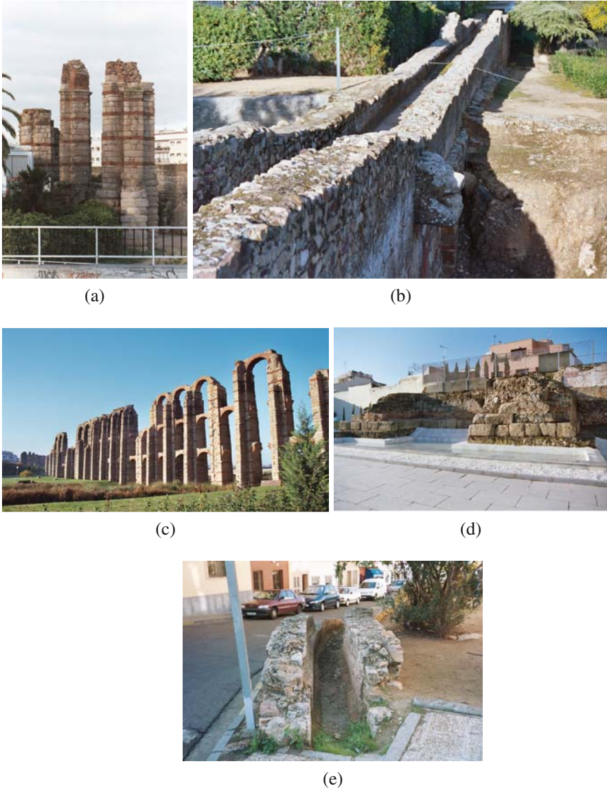
Fig. 7.17 Components of the water supply system in Merida (a) Only remains of the Las Thomas aqueduct bridge across the Rio Albarregas located near the hippodrome; (b) Las Thomas aqueduct downstream of the aqueduct bridge near the Roman theater. Shown on the right side of the aqueduct is a lion head made of stone which was used as a gutter spout. The remains of a castellum is nearby. (c) Los Milagros aqueduct bridge of the Proserpina aqueduct across the Rio Albarregas; (d) The remains and the reconstruction of the castellum downstream of the Los Milagros bridge; (e) Cornalvo aqueduct supplying water from the Cornalvo dam to Merida. Only a few remnants of this aqueduct are still visible near the bullfighting arena. (Copyright permission with L.W. Mays). Color version available in Appendix
