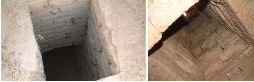
Fig. 5.5 Underground gutters at the northern platform
