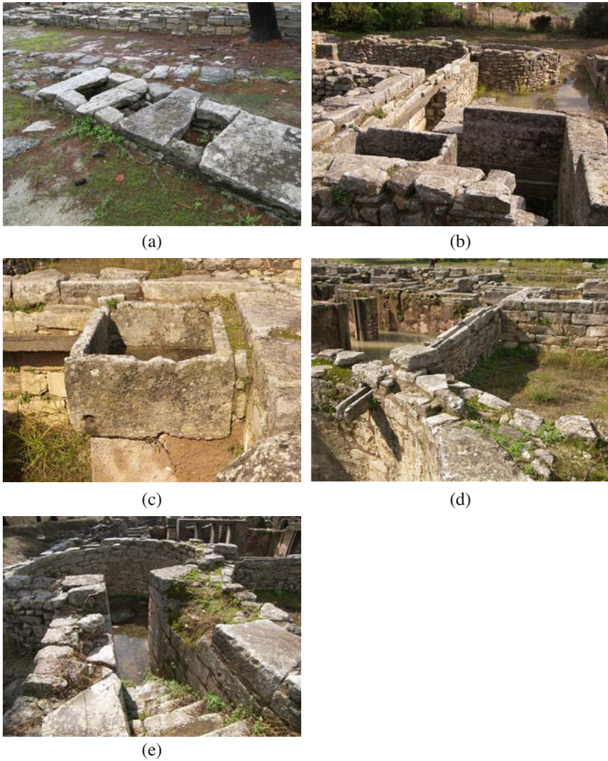
Fig. 1.7 Water system in Tyllissos, Crete. (a) Aqueduct bringing water from springs. (b) Sedimentation tank in foreground with stone channel connecting to cistern. (c) Sediment tank (d) Channel connecting sediment tank to cistern. (e) Steps leading down to cistern (photos copyright by L.W. Mays). Color version available in Appendix
