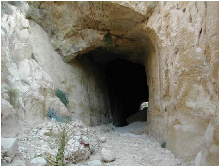
Fig. 1.17 Tunnel excavated by Nabataeans to divert flood water at the entrance of the Siq from Wadi Musa into Siq Mudhlim tunnel (photo courtesy of Mac McKee)
