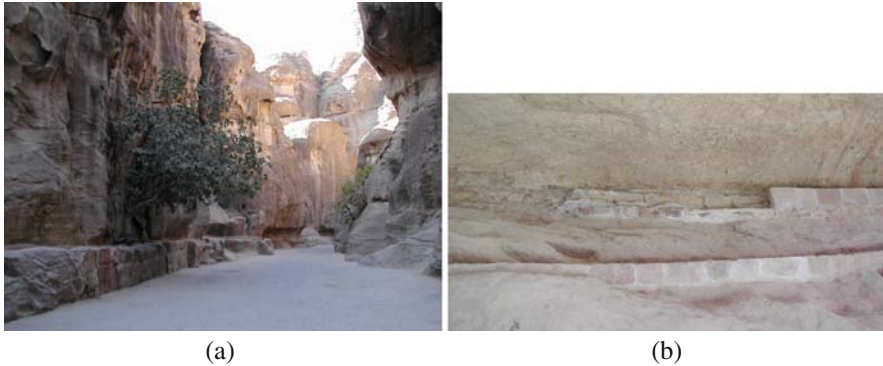
Fig. 1.18 The Siq (a) The gravine with the water channel (elevated bench flume) along the side. (b) Piping elements in the Siq showing clay pipes with bell and spigot joints filled with mortar (photos courtesy of Mac McKee)
