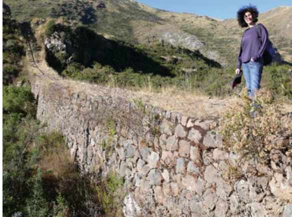
Fig. 9.18 Elevated portion of the main aqueduct in Tipon (photo copyright by Yuri Gorokhovich). Color version available in Appendix
