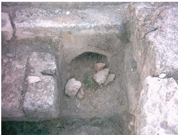
Fig. 8.10 Entrance of the water in the guard tower (point 2 in Fig. 8)
