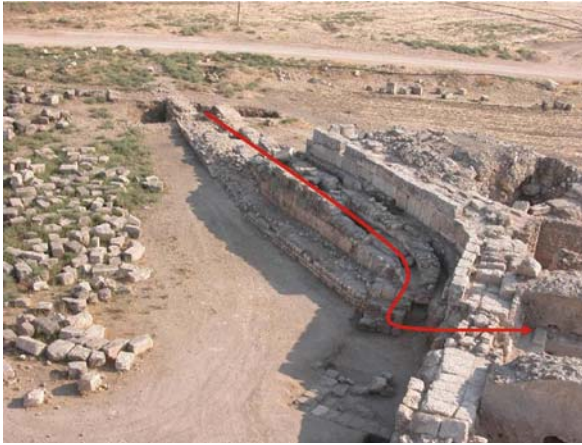
Fig. 8.6 Outer aqueduct delivering water into a cistern. Color version available in Appendix
