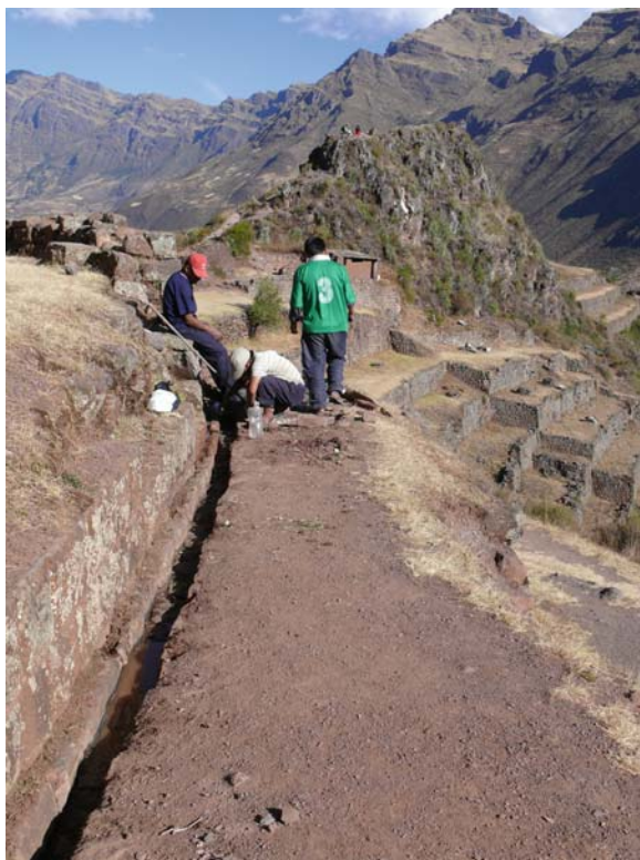
Fig. 9.27 Reconstruction of ancient water works often “masks” the original structure (photo copyright by Yuri Gorokhovich)
