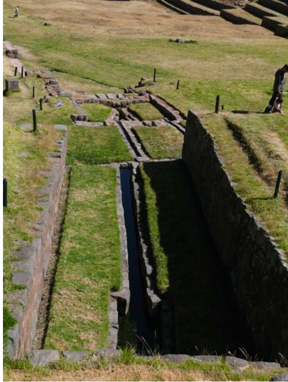
Fig. 9.21 Tipon spring located at the head of the central terrace ravine. Water was distributed to ceremonial fountains and to irrigated agriculture through canals (photo copyright by Yuri Gorokhovich). Color version available in Appendix
