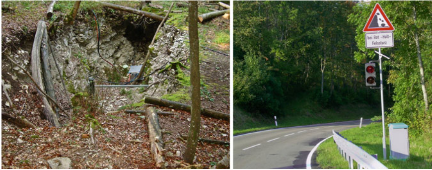
Fig. 2.10 Early warning system at Winkelgrat landslide equipped with automatic extensometers ( left ) and traffic light for road closure ( right )
