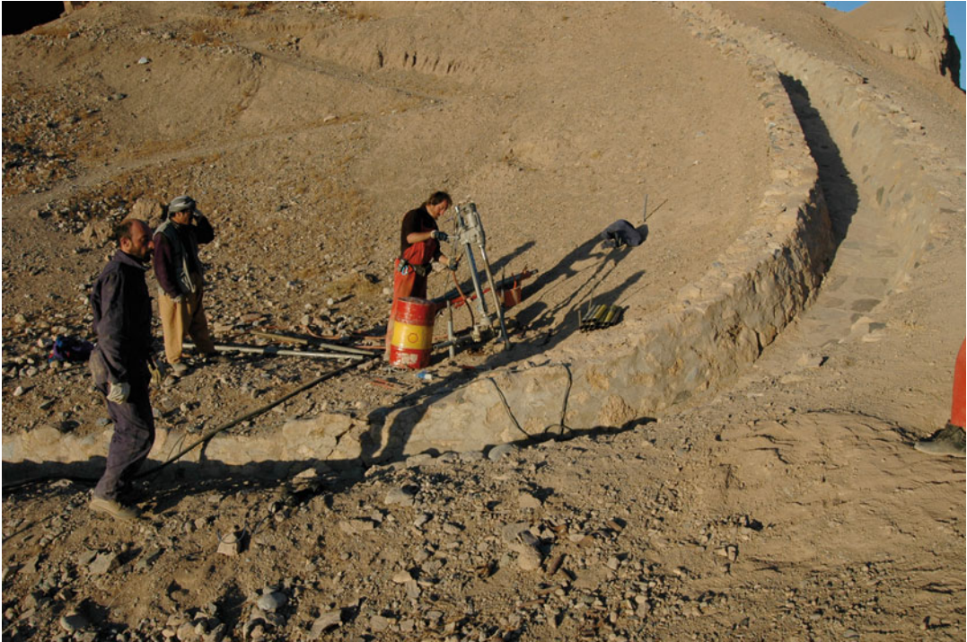
Fig. 11.40 Detail of the grouting from the top of cliff
