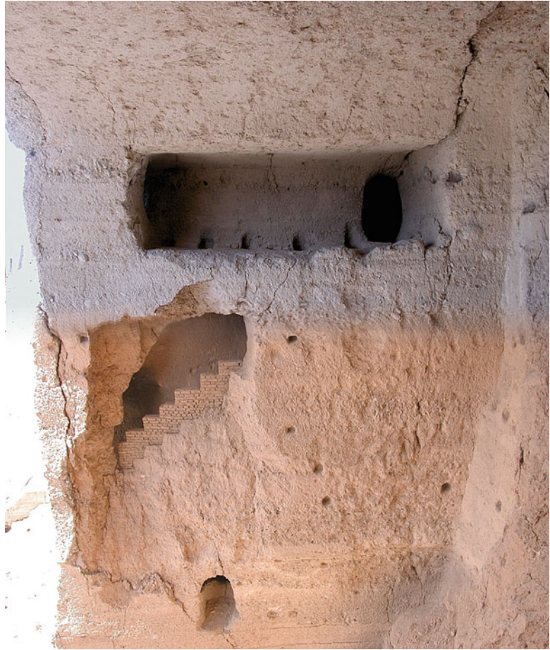
Fig. 11.20 The most unstable element (pillar) in the western side of Eastern Giant Buddha niche
