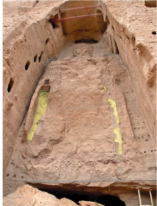
Fig. 13.1 Eastern Buddha, preserved original clay plaster layers (marked in yellow), in total about 21 m 2 , preserved in 2008 by gluing and needling
