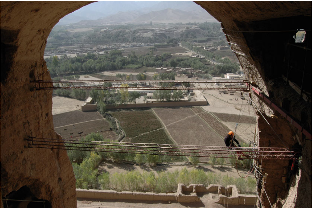
Fig. 11.28 Drilling for nails
