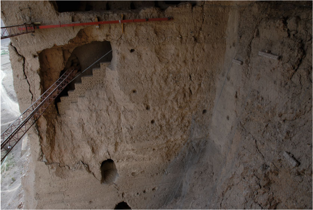
Fig. 12.3 The metallic net protecting from the detachment of small rocks from the shear band of destroyed statue. The photo also shows the wooden spacers, covered
