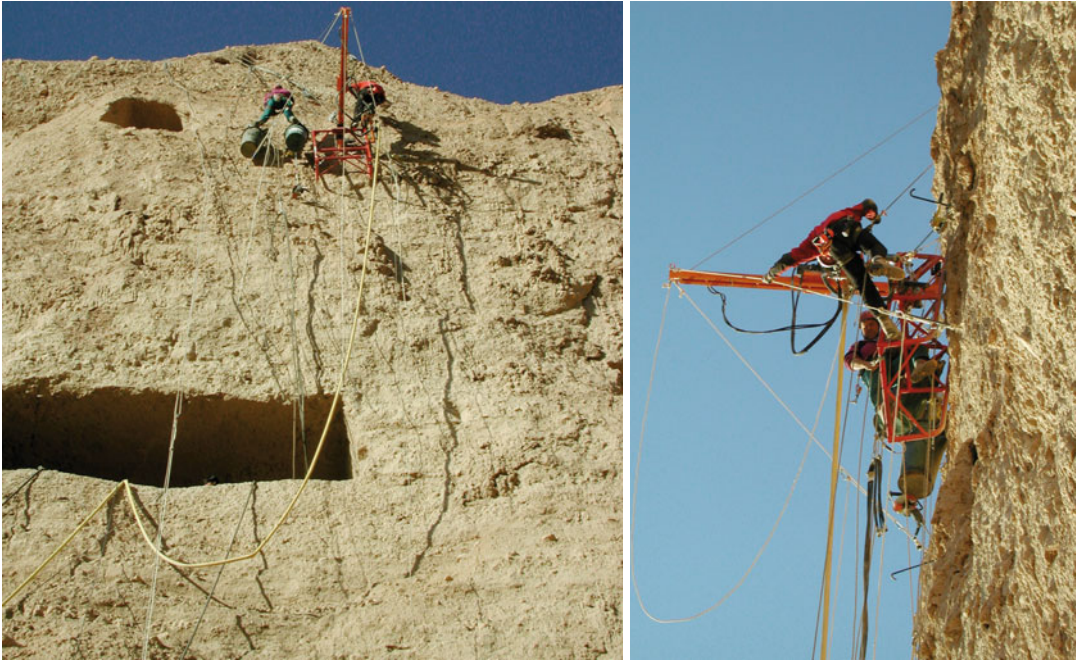
Fig. 11.11 Final consolidation with the use of professional climbers and large rotary machine
