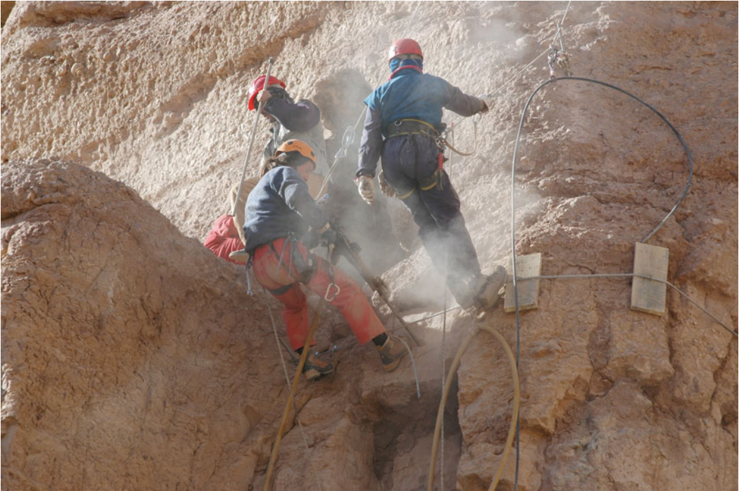
Fig. 11.42 Drilling in the lower part of the niche
