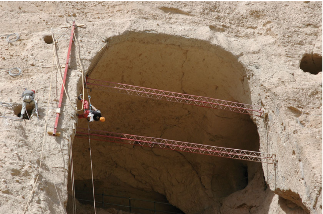
Fig. 11.24 Temporary protection on the west side of the niche
