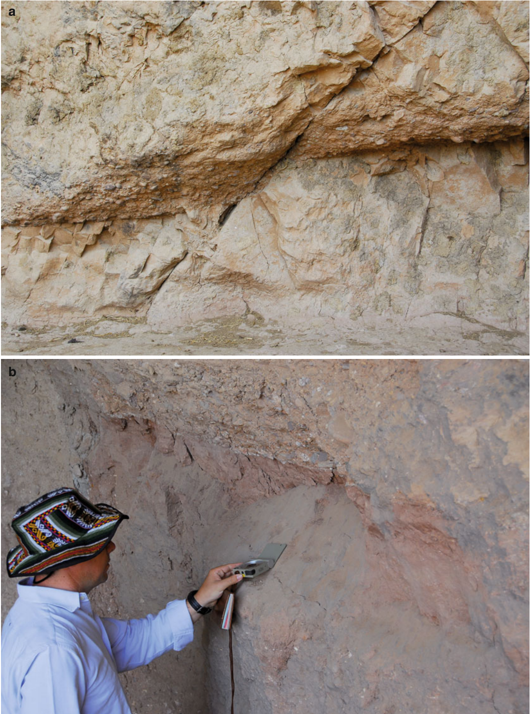
Fig. 5.16 View of medium-low angle faults affecting the outcropping base rocks in the eastern side of the cliff
