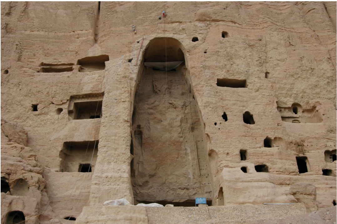
Fig. 11.32 View during execution of the work
