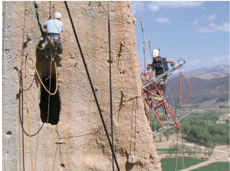
Fig. 11.11 Final consolidation with the use of professional climbers and large rotary machine
