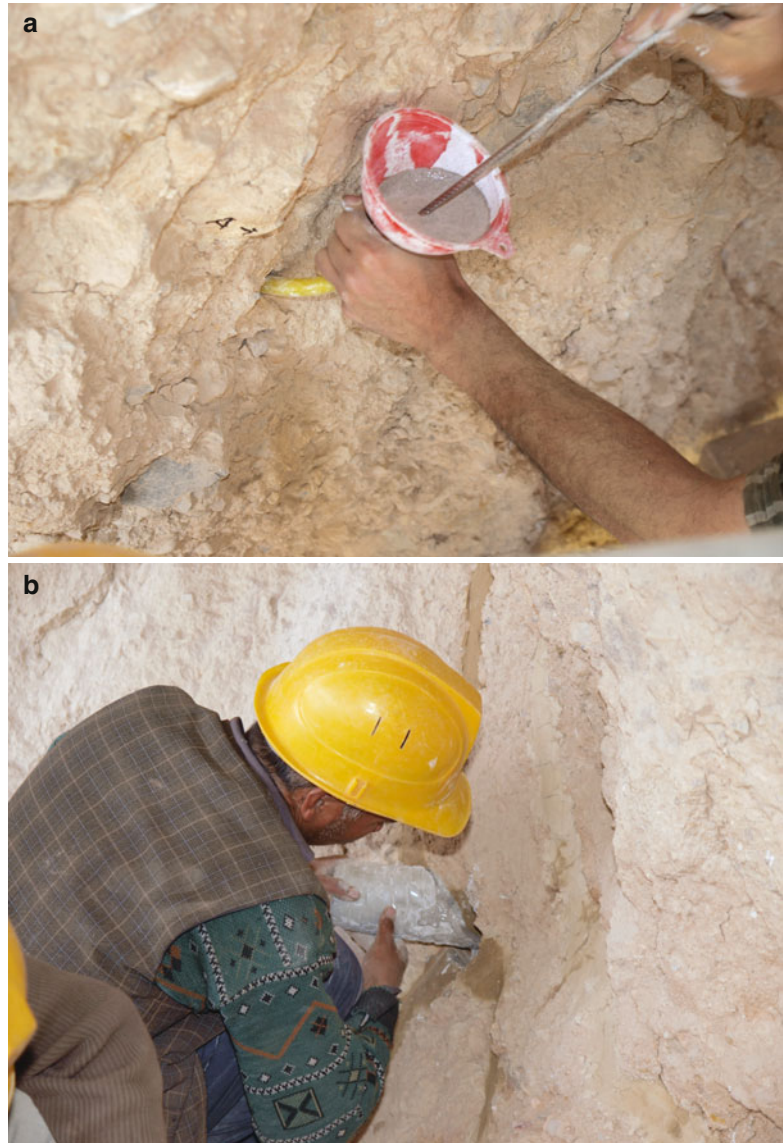
Fig. 13.14 (a, b) Backfilling the cracks with mortar
