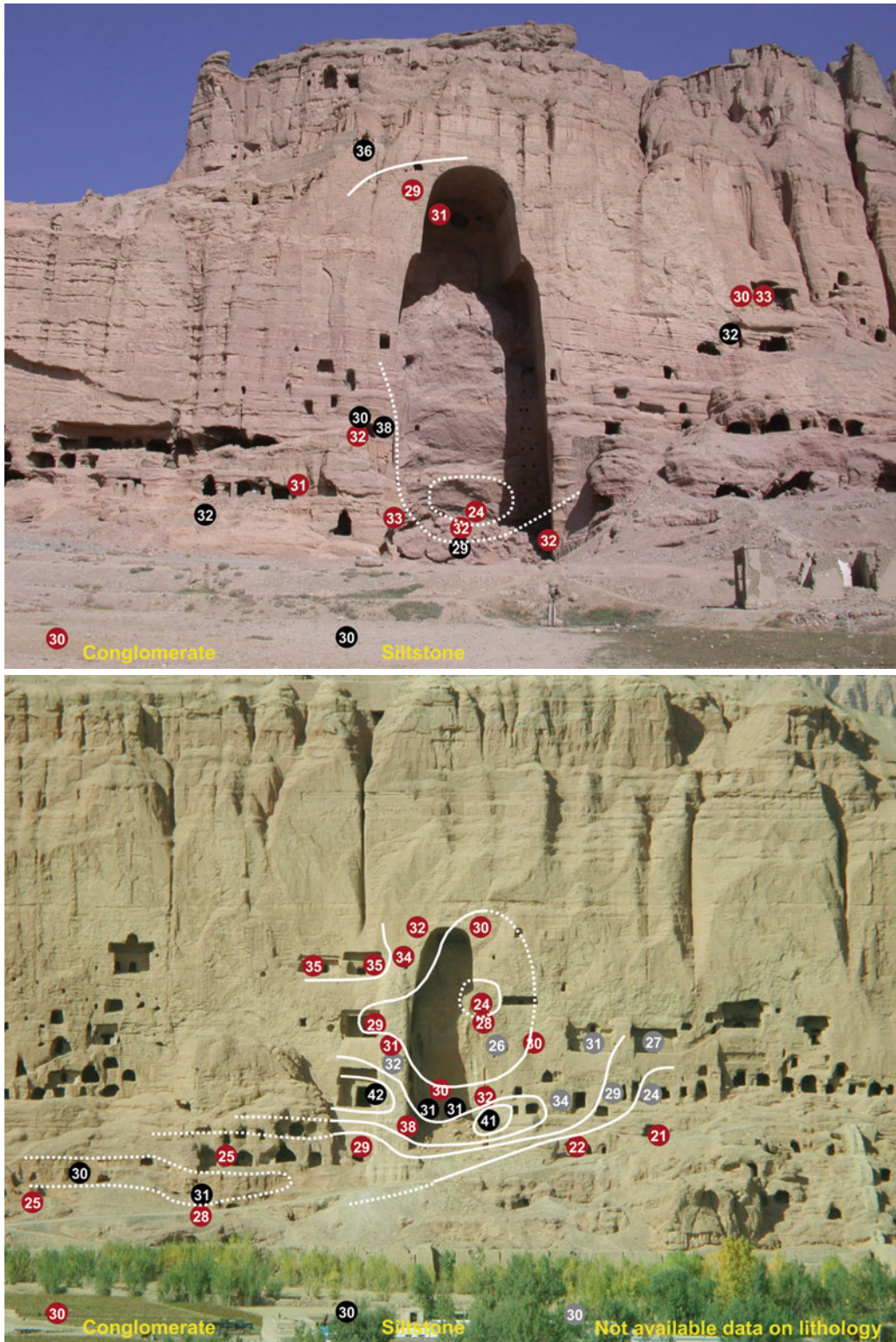
Fig. 7.15 Uniaxial compressive strength (MPa) from Schmidt hammer field survey, in the surrounding of both niches ( top the Western giant Buddha niche and bottom the Eastern Buddha)
