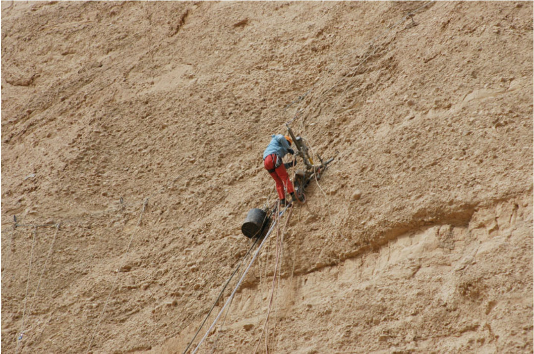
Fig. 11.31 Drilling for the installation of long anchors on top of niche
