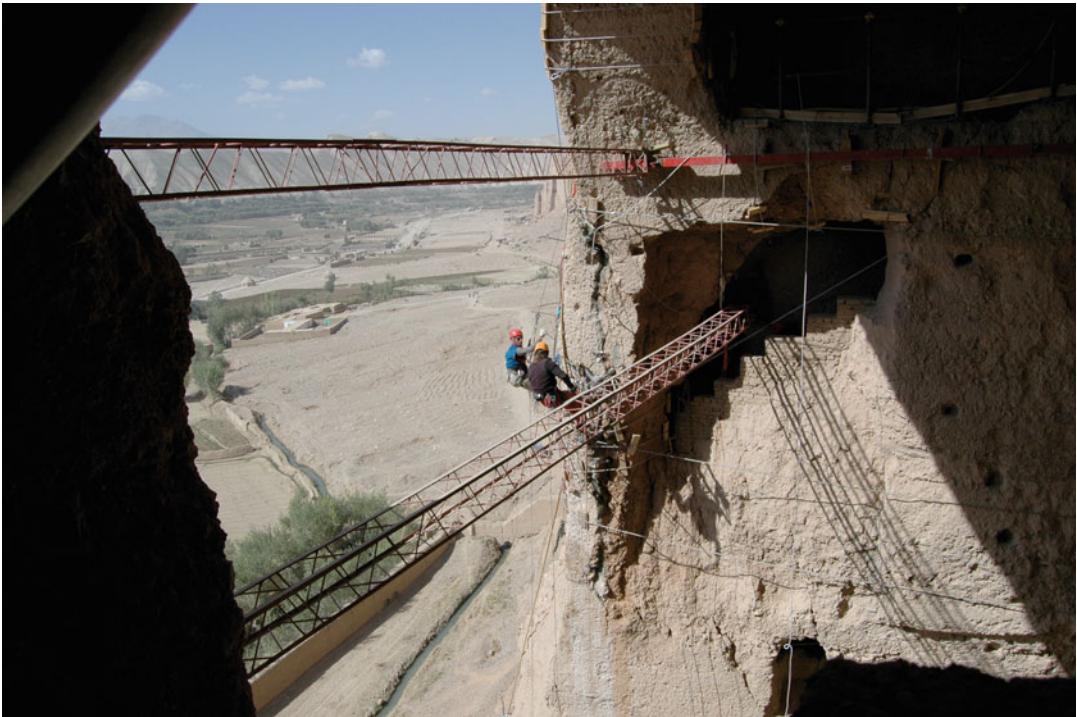
Fig. 11.26 Installation of steel cables as temporary protection
