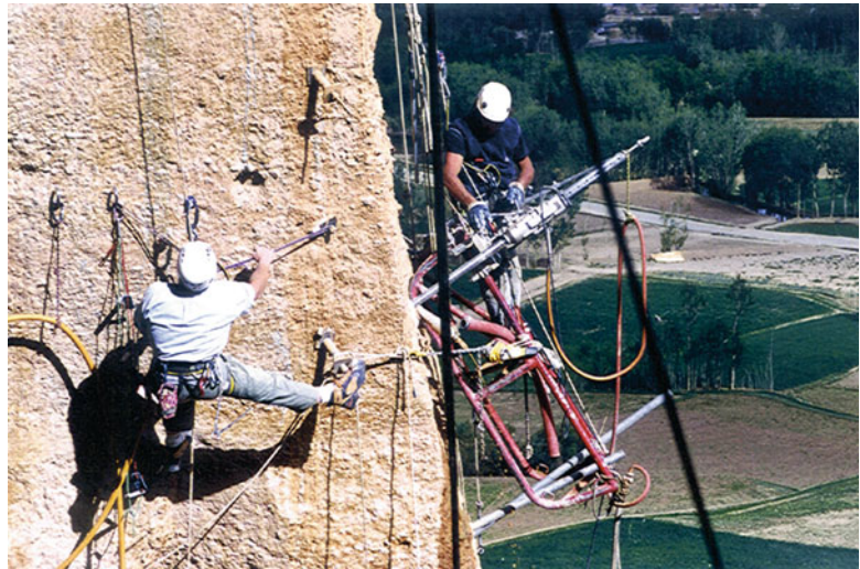
Fig. 11.14 Drilling for nails at the corner of niche
