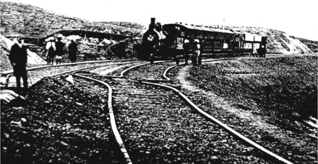
Plate 6.6 Contraction of the railway line where it crossed the 1892 Chaman fault (From Griesbach 1893). The sinistral fault slip is estimated here to have exceeded 70 cm
