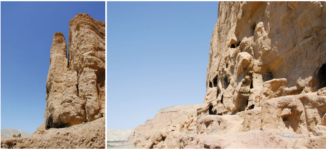
Fig. 5.29 Potential rock toppling in the western side ( left ) and fallen block caused by toppling in the eastern side ( right )
