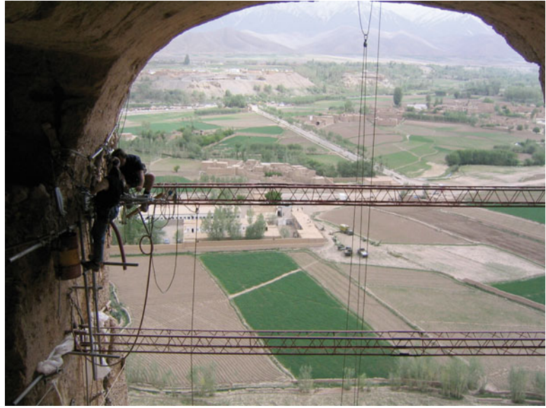
Fig. 11.13 Execution of nails on the roof of the niche
