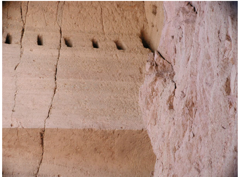
Fig. 12.7 ( Center on the left ) Detail of detachment in the Western Giant Buddha
