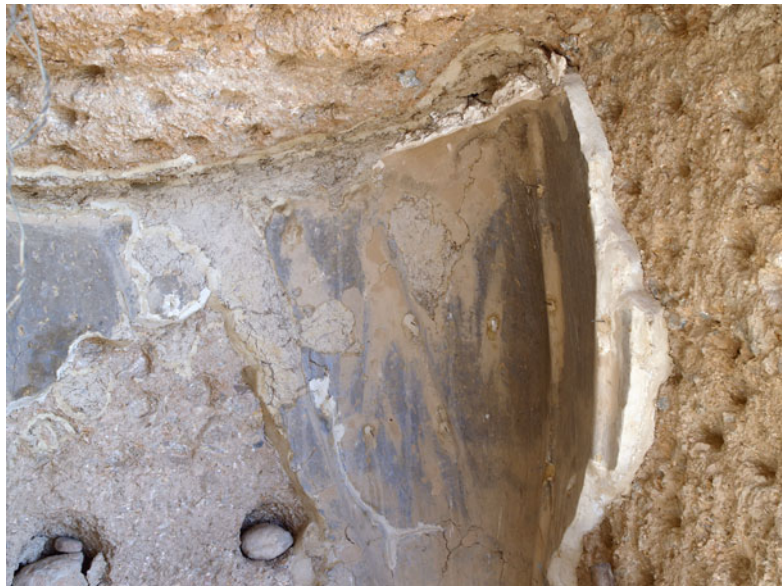
Fig. 13.9 Bonded and secured clay plaster fragment underneath the arm hole
