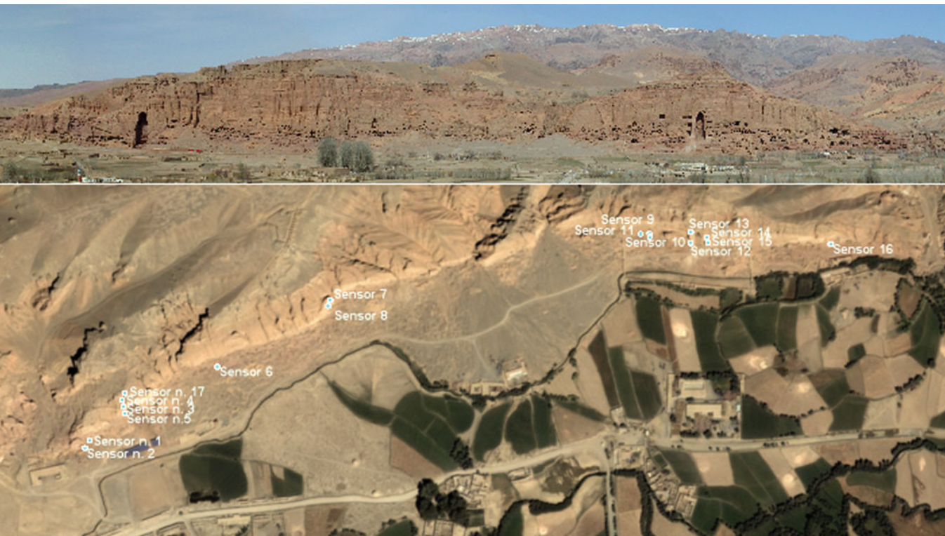
Fig. 10.5 The manual monitoring network for crack gauge measurement
