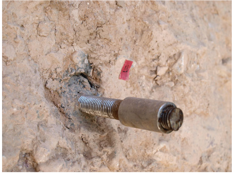
Figs. 13.20 and 13.21 Anchor of stainless steel (V2A) with a thickness of 22 mm
