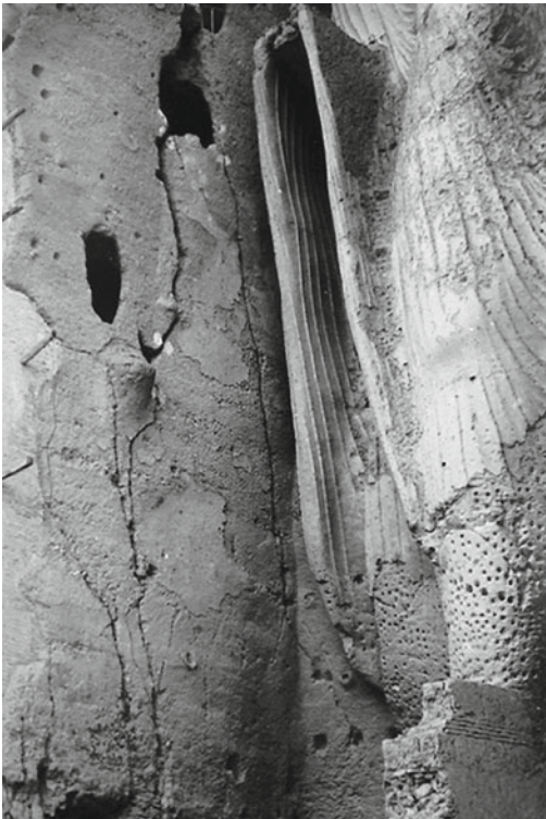
Fig. 9.5 Pattern of discontinuities in the Eastern Giant Buddha niche both before intervention of the Indian Archaeological Survey and currently (Courtesy Michel Jansen)
