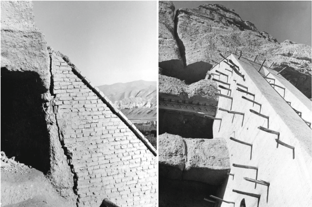
Fig. 9.1 The top of the buttress constructed by the French Archaeological mission (Photos A. Bruno, Sept. 1960)
