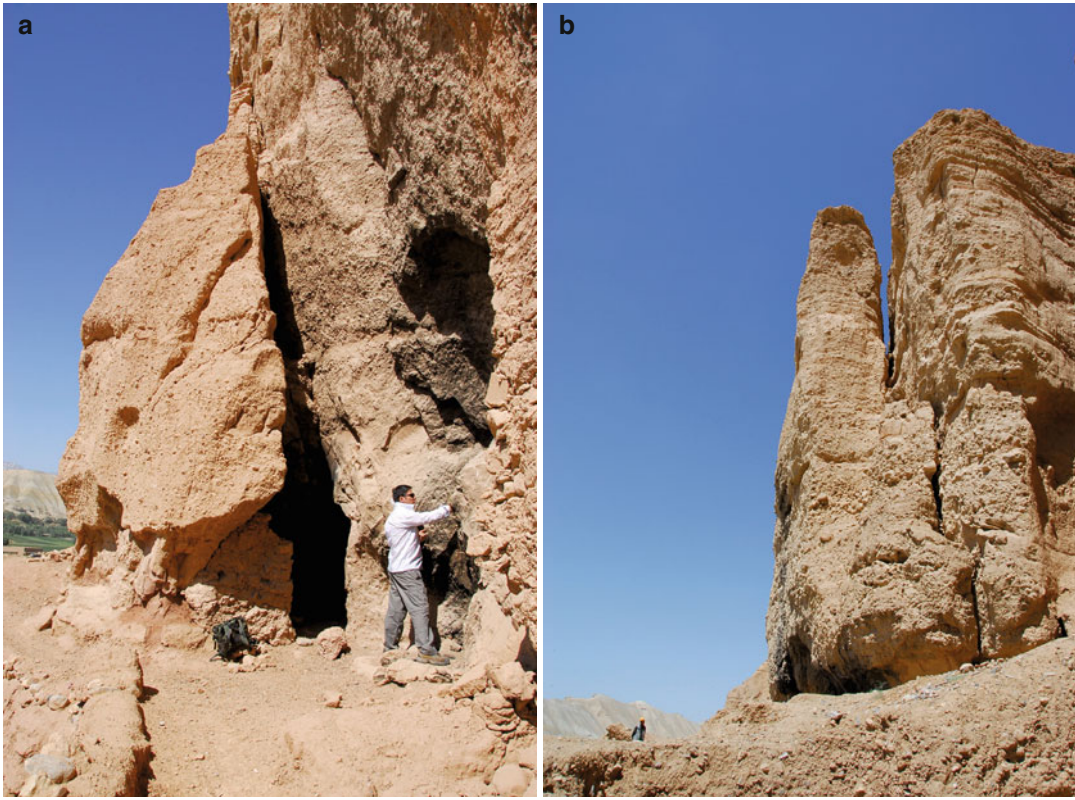
Fig. 5.15 Example of joints parallel to the cliff main orientation
