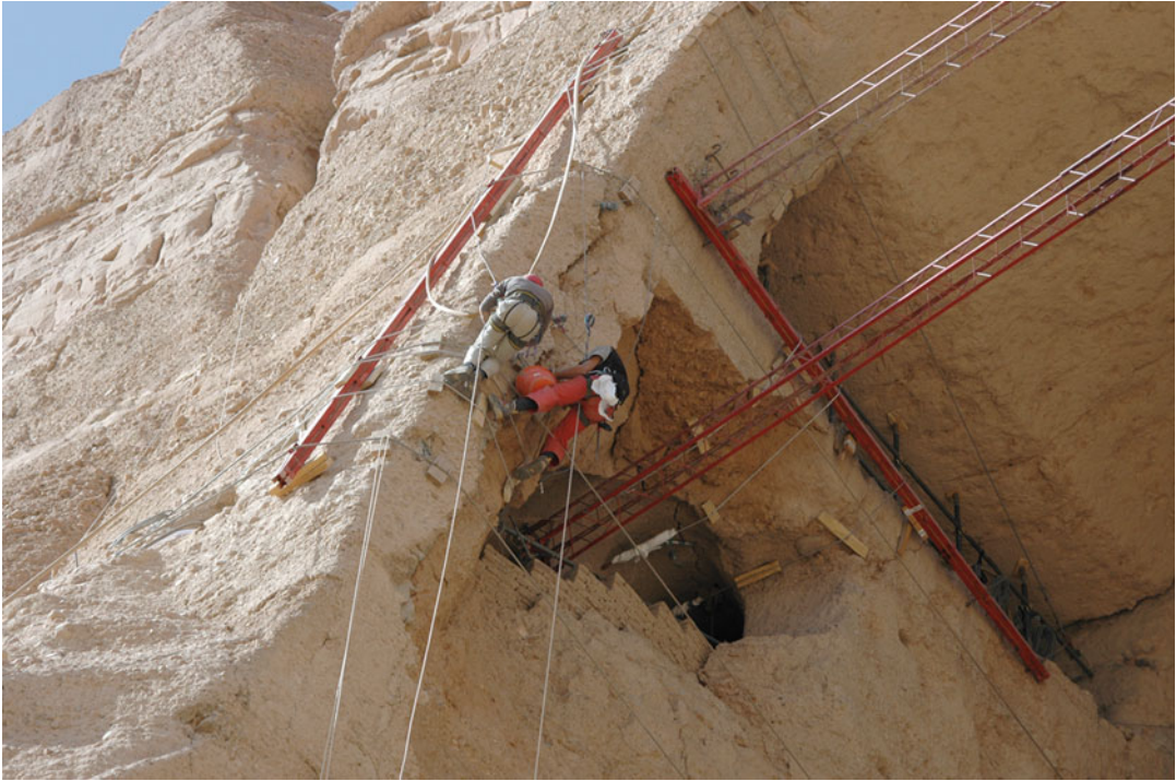
Fig. 11.22 The temporary support necessary for secure execution of the work in the western wall: two long iron beams replaced in the upper part of the niche, the short iron/wood struts for local support and the steel cables
