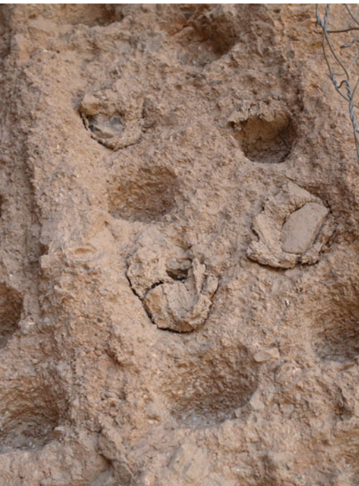
Fig. 13.5 Clay lumps pressed into the holes with stones
