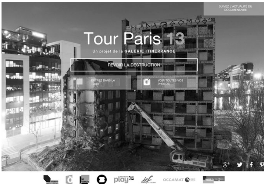
Fig. 10.4 On-line broadcast of the demolition of the Paris 13 tower. Source http://www.tourparis13.fr/destruction/src/index.php
