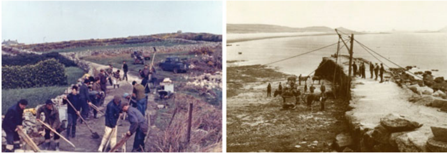
Fig. 5.28 Community action: roadworks on St Martin's (left, Source: Isles of Scilly Museum [around 1960c]); construction of St Martin's Quay (right, Source Isles of Scilly Museum [around 1960b])
