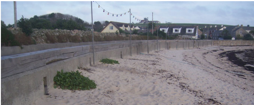
Fig. 5.37 Raised seawall in Old Town, December 2013
