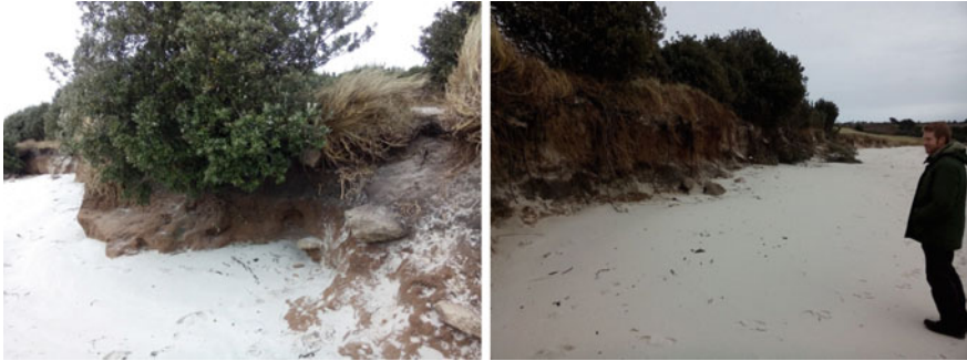
Fig. 5.15 Erosion on St Martin's, February 2014
