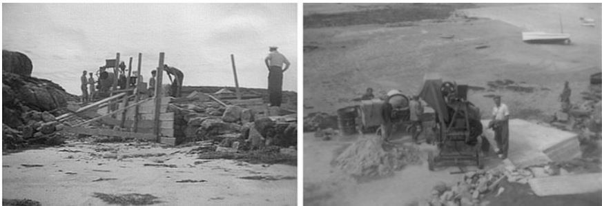
Fig. 5.29 Construction of Church Quay on Bryher, 1960s (Source both, Isles of Scilly Museum [around 1960a])
