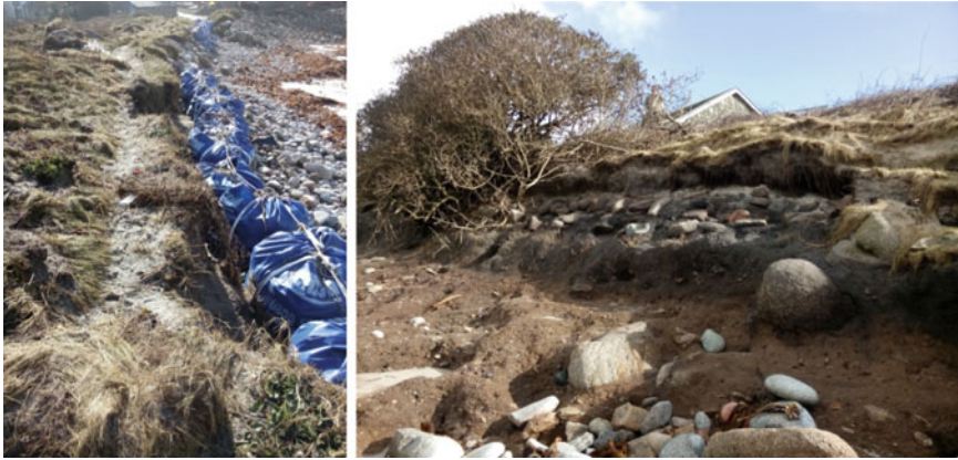
Fig. 5.45 Coastal protection on St Agnes: repaired seawall ( left ), and local solution to prevent erosion ( right ), both February 2014
