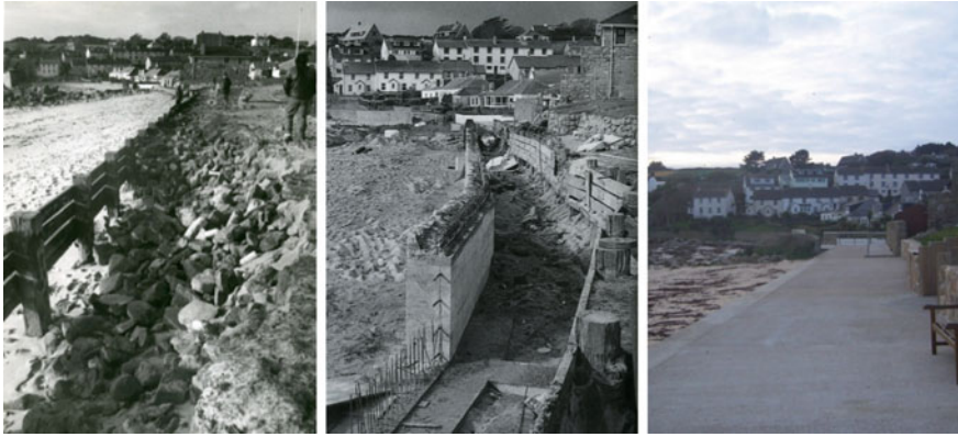
Fig. 5.36 Seawall at Portherssa (from left to right ): Wooden sea wall in the 1960s ( Source Isles of Scilly Museum [around 1960d]), concrete seawall under construction in 1995 ( Source Gibson 1997b: 26), redeveloped beachfront in 2014
