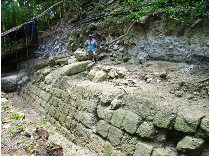
Fig. 12.14 Example of a Late Preclassic wall, found at the base of the third level of Danta pyramid at El Mirador, showing the large blocks placed with the long axis into the fill of the building, requiring much more material and labor to construct the same surface area. The entire structure of Danta is built in this fashion ( Photo R.D. Hansen)
