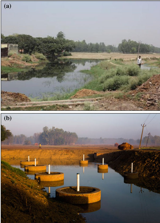
Fig. 3 Status of the UTFI site a before and b after implementation
