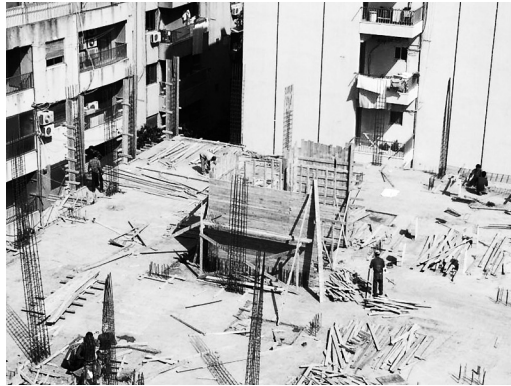
Figure 8.2 A very chaotic construction site.
